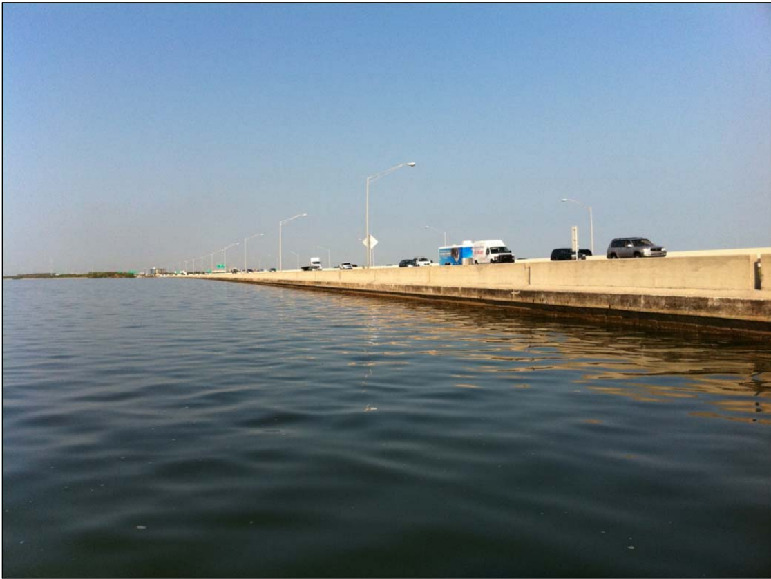
Photo 1. View of bridge embankment and seawall.
