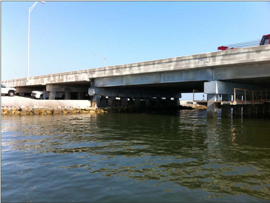
Photo 3. View of terminus of bridge embankment.
