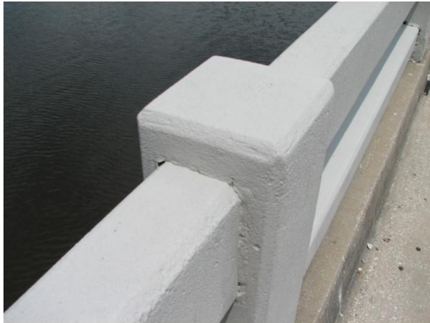
Light gray painted concrete guardrail
