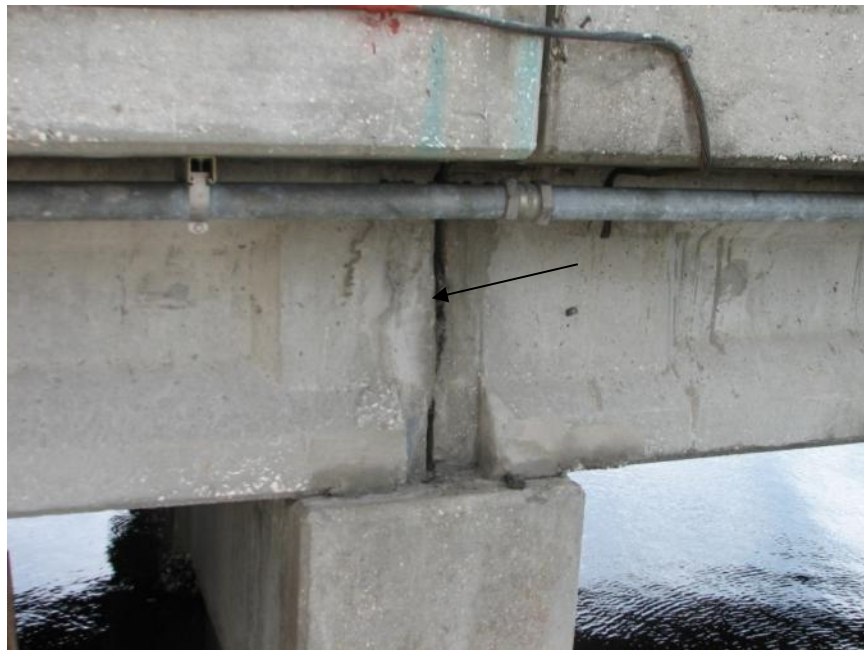
Homogeneous Material 2 – Expansion joint board between beams
