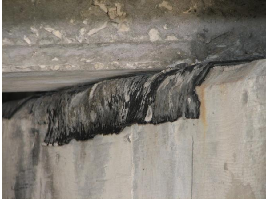
Homogeneous Material 1 – Black tar paper on all bent caps
