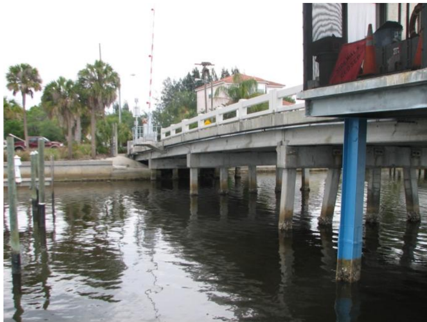
Homogeneous Material 4 – Various concrete elements (bents, decking, piles and guardrail)
