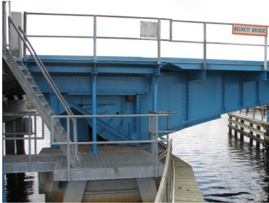
Blue painted structural steel and bascule bridge structure
