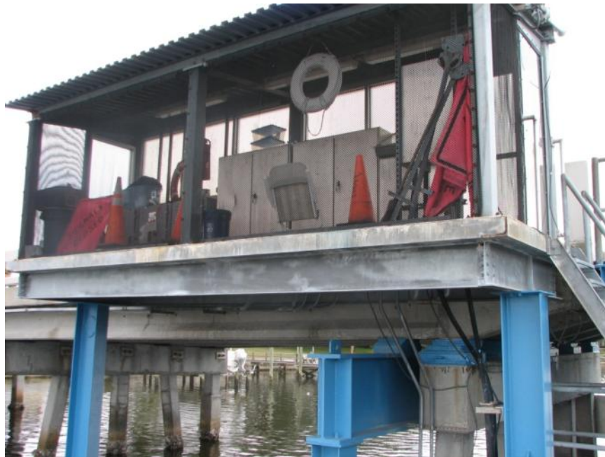
View of bridge tender house
