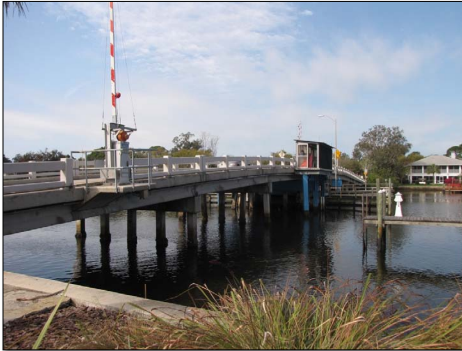
Figure 11.5 – Beckett Bridge (8PI12017) in Pinellas County, facing southwest
