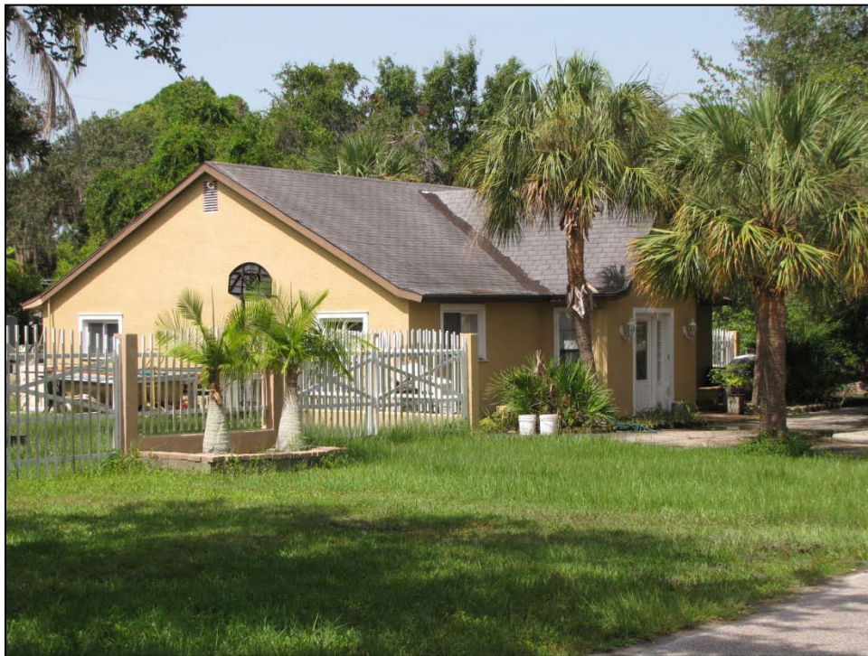
Figure 11.7 – 435 Doric Court (8PII2069) in Pinellas County, facing southwest
