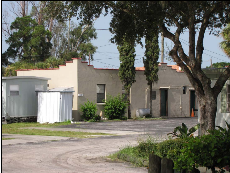
Figure 11.12 – 403 Riverside Drive (8PI12046) in Pinellas County, facing south
