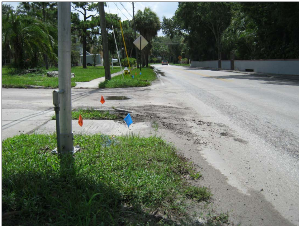
Figure 11.3 – Buried Utilities on Riverside Drive at Forest Avenue, facing east
