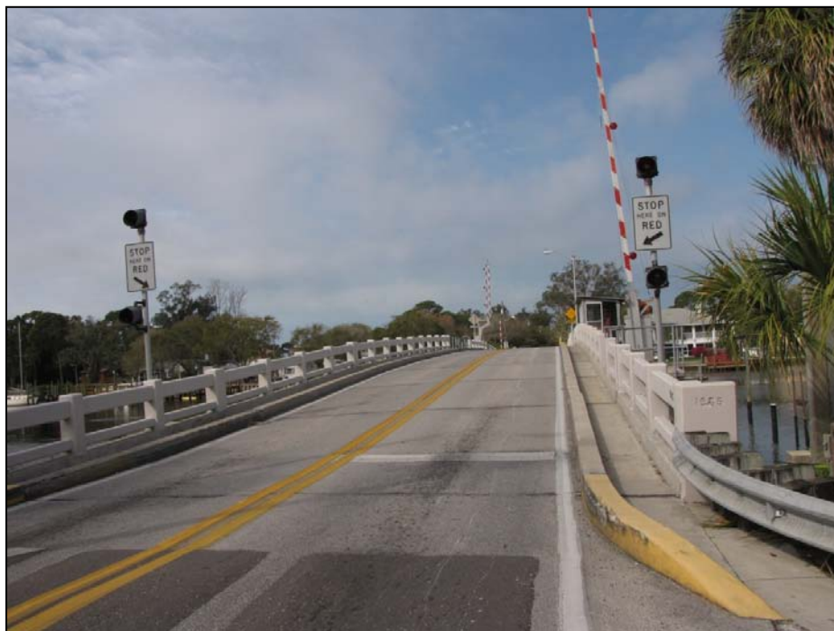
Figure 11.6 – Beckett Bridge (8PI12017) in Pinellas County, facing west
