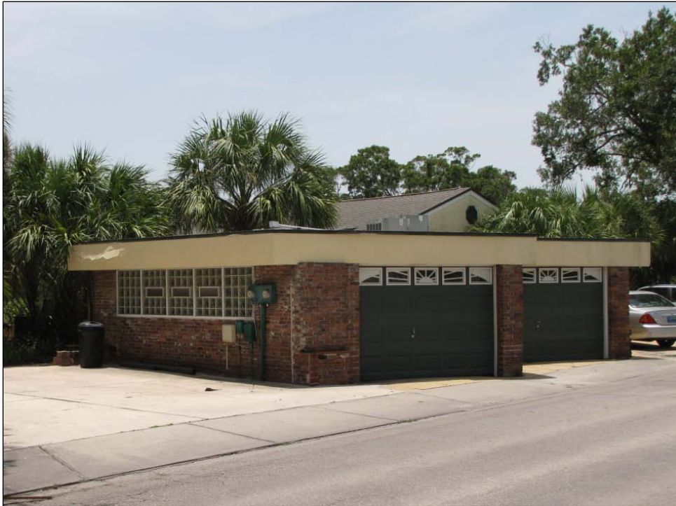
Figure 11.21 – 301 North Spring Boulevard (8PI12055) in Pinellas County, facing southwest
