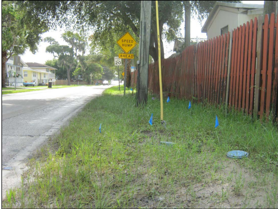
Figure 11.2 – Buried Utilities along Riverside Drive, facing east
