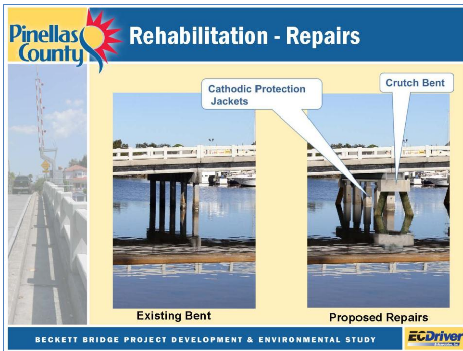
Figure 3.4 – Rehabilitation Repairs – Cathodic Protection Jackets and Bents
