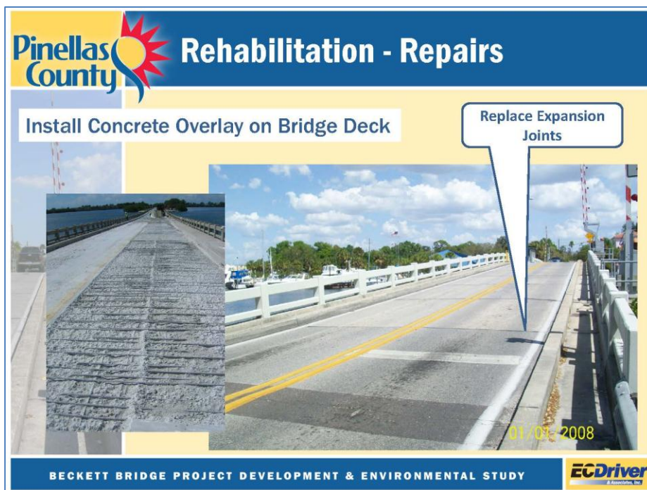
Figure 3.7 – Rehabilitation Repairs – Bridge Deck Concrete Overlay and Expansion Joint Replacement
