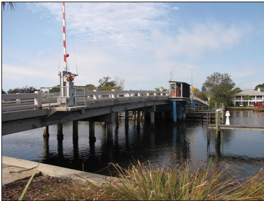
Figure 5.1 – Beckett Bridge (8PI12017) in Pinellas County, Facing Southwest
