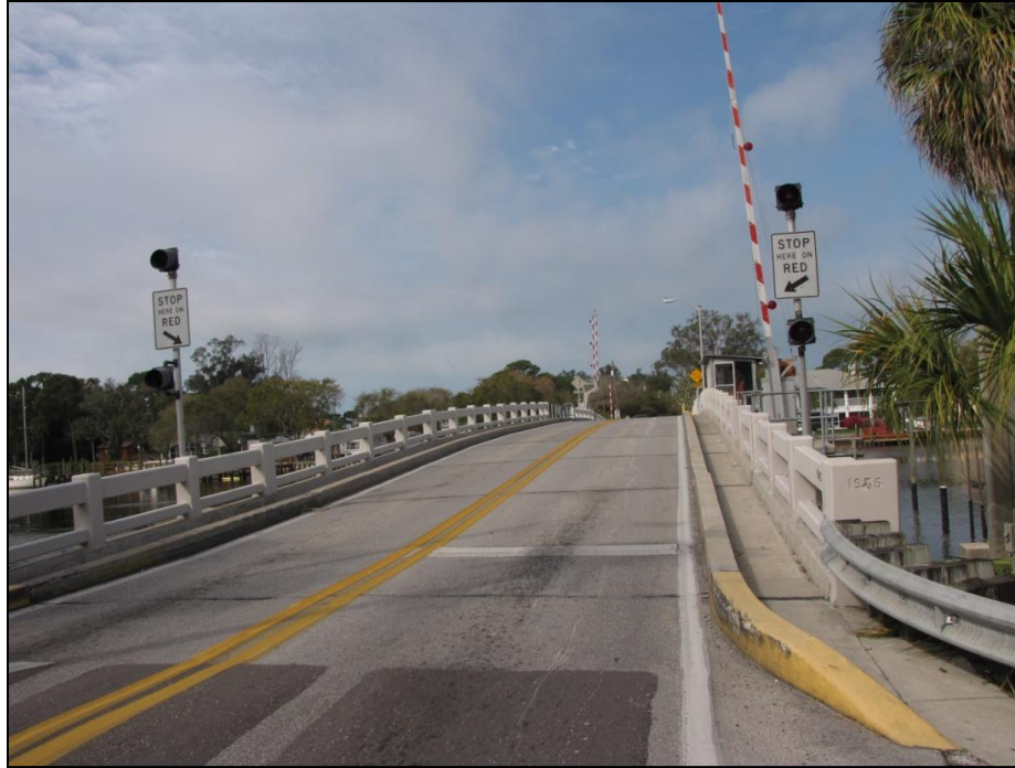
Figure 5.2 – Beckett Bridge (8PI12017) in Pinellas County, Facing West
