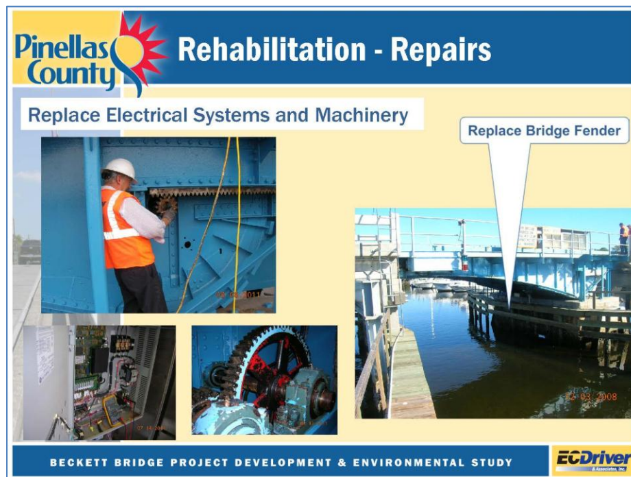
Figure 3.6 – Rehabilitation Repairs – Replacement of Electrical Systems, Machinery, and Bridge Fender
