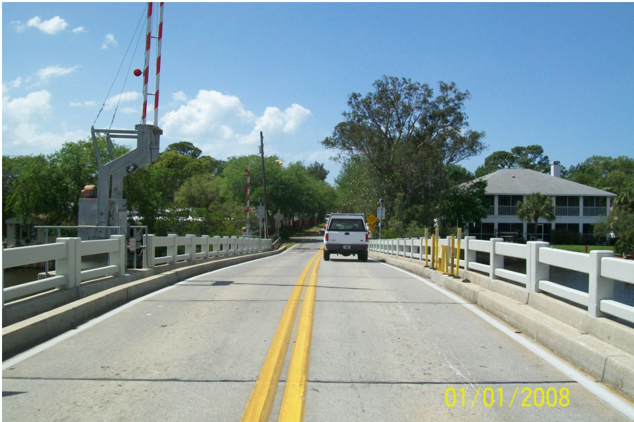
Beckett Bridge – View from Roadway
