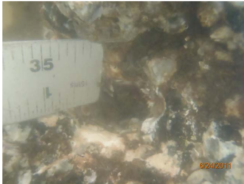
PHOTO 44: 204/4 P/S Conc Column
