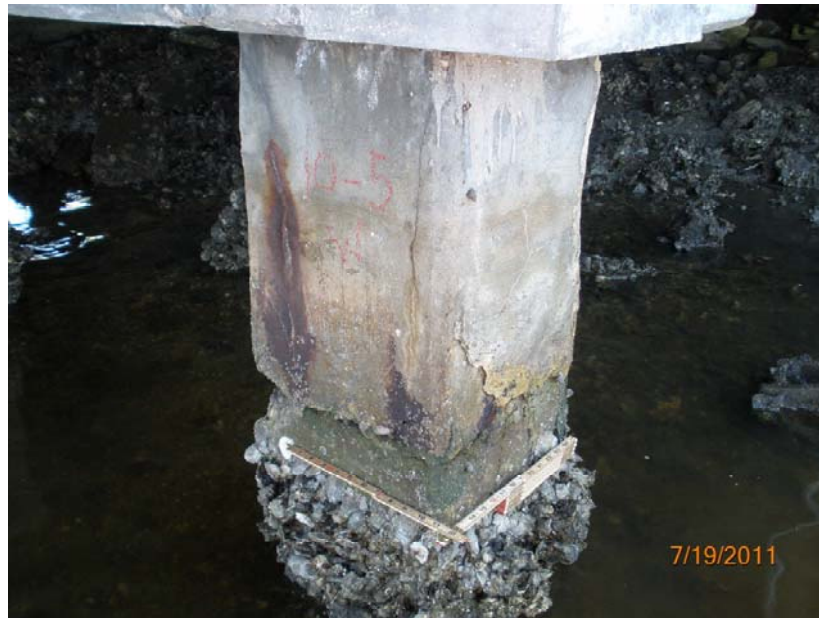
PHOTO 43: 204/4 P/S Conc Column
