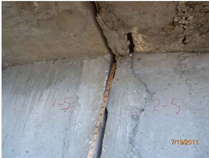
PHOTO 32: 12/4 Bare Concrete Deck
