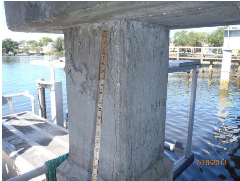
PHOTO 41: 204/4 P/S Conc Column
