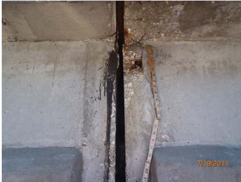
PHOTO 36: 109/4 P/S Conc Open Girder
