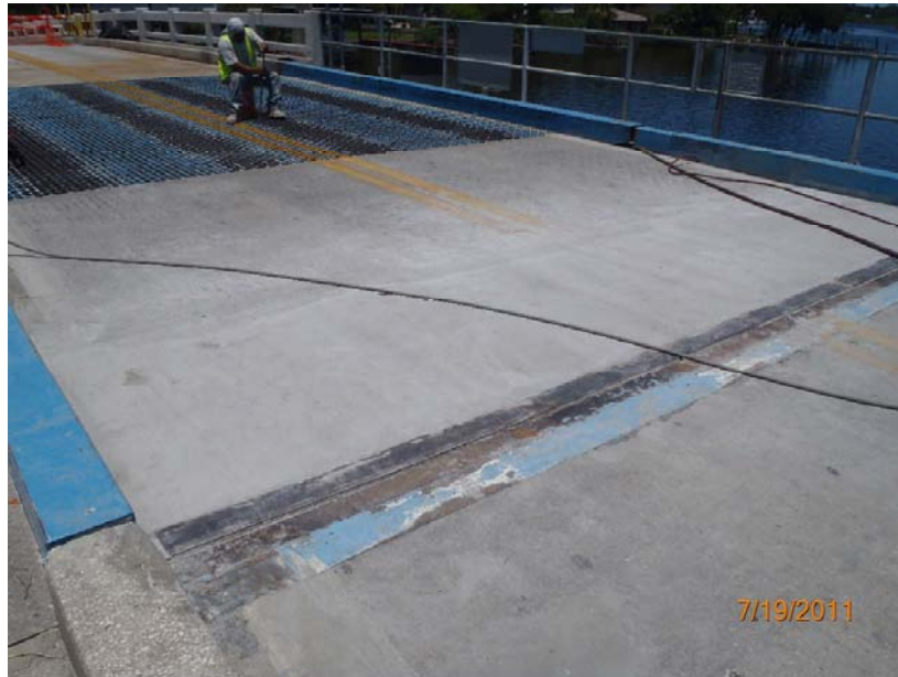
PHOTO 5: 29/4 Steel Deck/Conc Grid
