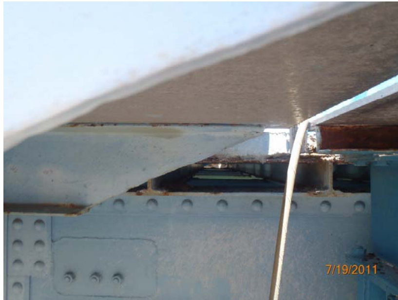
PHOTO 6: 29/4 Steel Deck/Conc Grid
