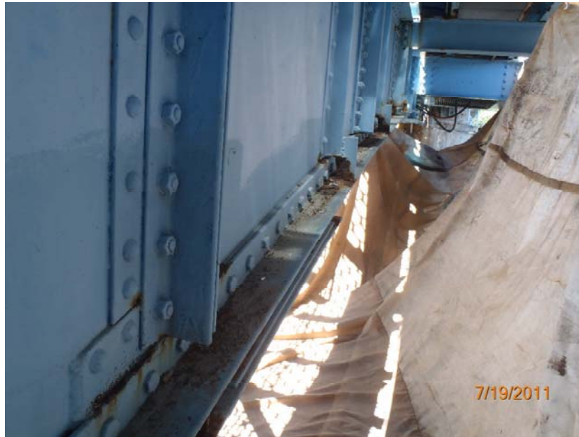
PHOTO 8: 107/4 Paint Stl Opn Girder
