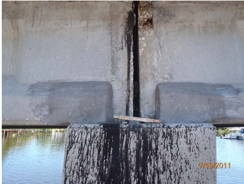
PHOTO 37: 109/4 P/S Conc Open Girder
