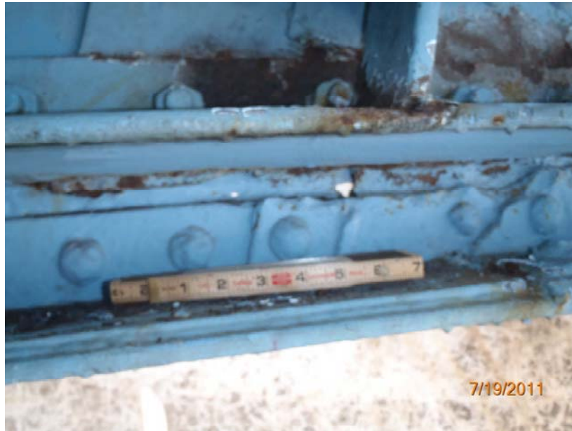
PHOTO 7: 107/4 Paint Stl Opn Girder
