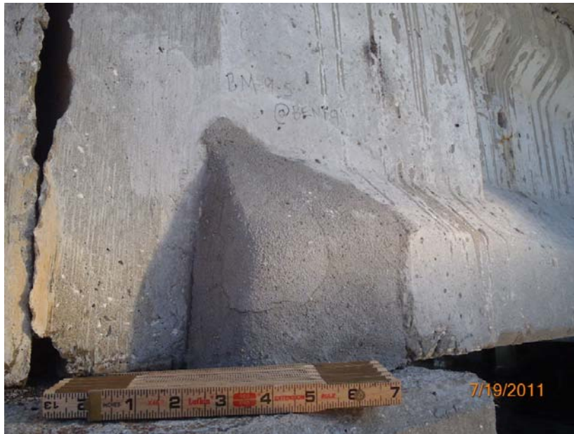
PHOTO 40: 109/4 P/S Conc Open Girder
