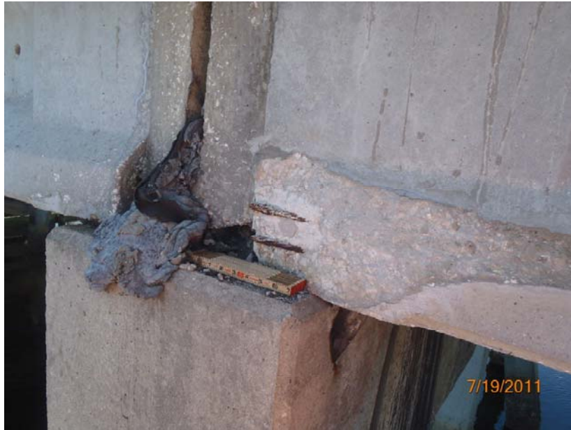
PHOTO 38: 109/4 P/S Conc Open Girder
