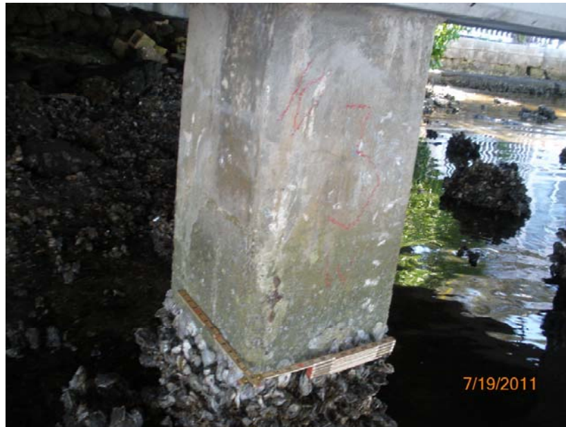
PHOTO 42: 204/4 P/S Conc Column
