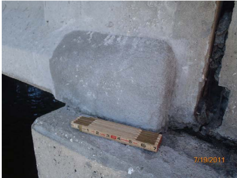
PHOTO 39: 109/4 P/S Conc Open Girder
