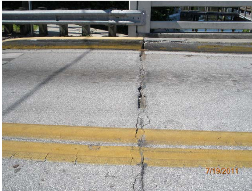
PHOTO 35: 301/4 Pourable Joint Seal
