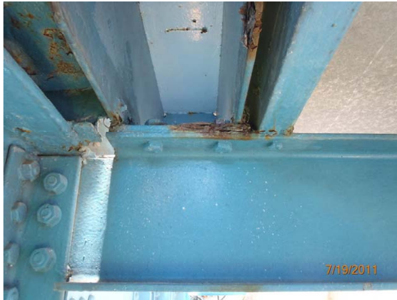
PHOTO 2: 28/4 Steel Deck/Open Grid
