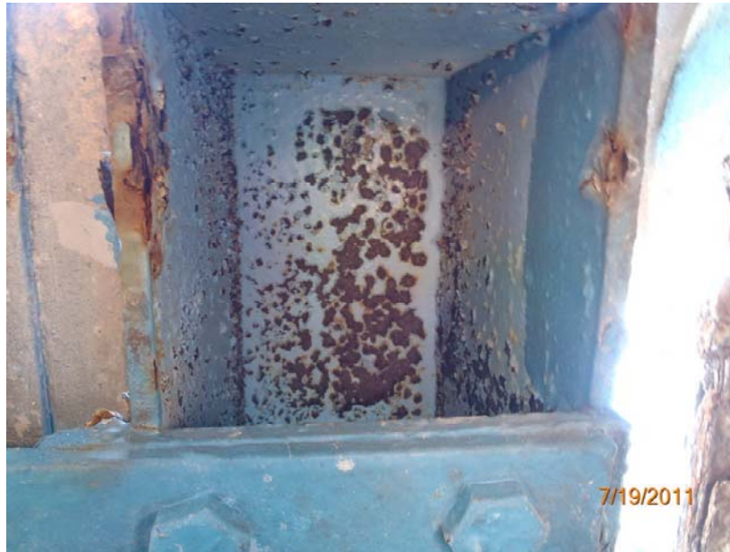
PHOTO 4: 28/4 Steel Deck/Open Grid
