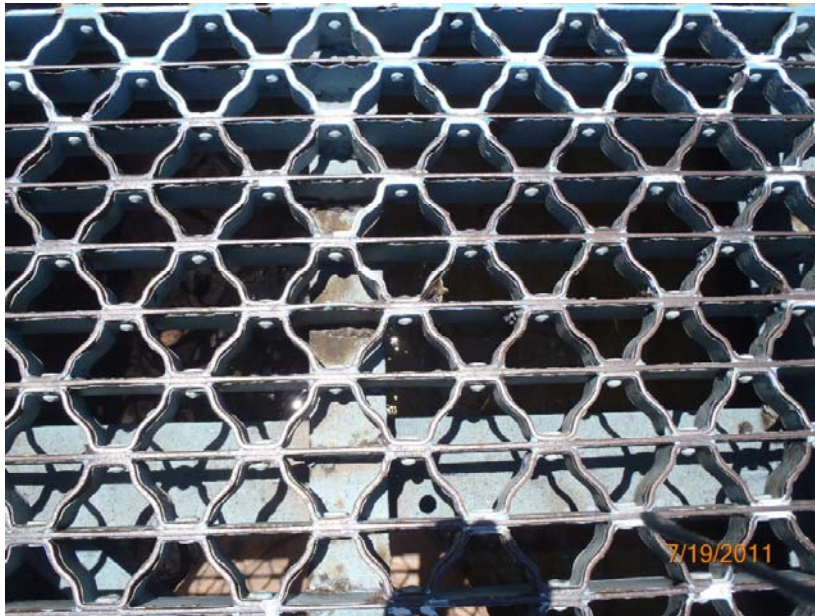
PHOTO 3: 28/4 Steel Deck/Open Grid
