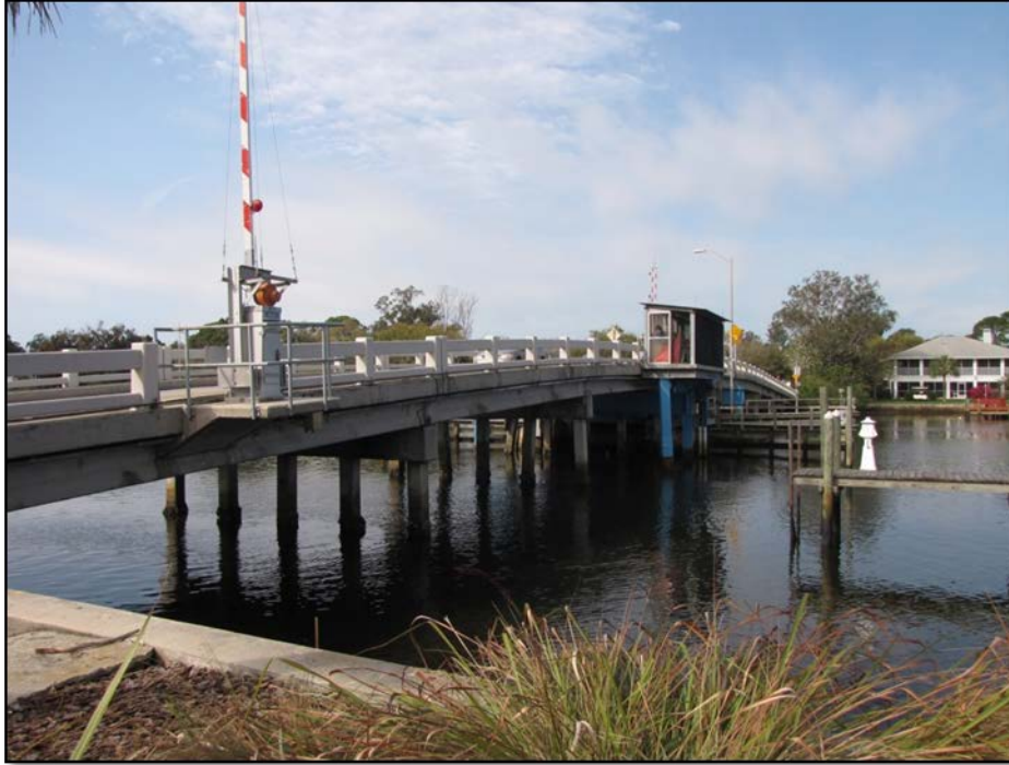
Photo 5: Beckett Bridge (8PI12017)
