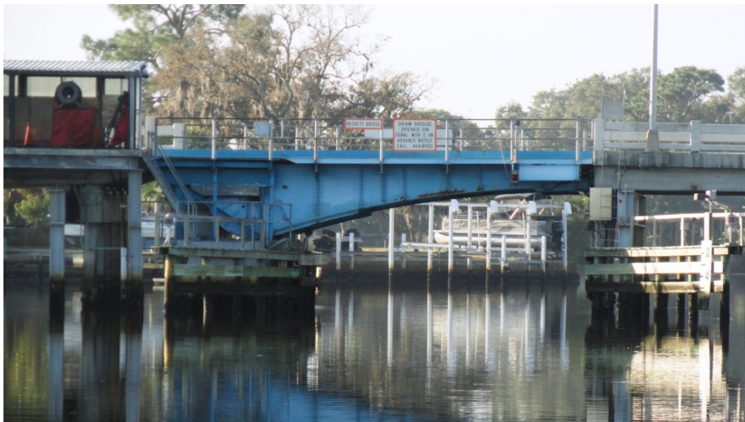
Photo 4: Bascule Leaf in Closed Position
