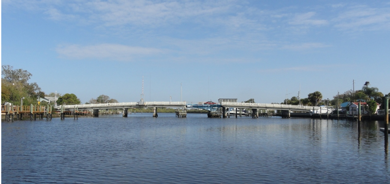
Photo 1: Beckett Bridge – South Elevation View
