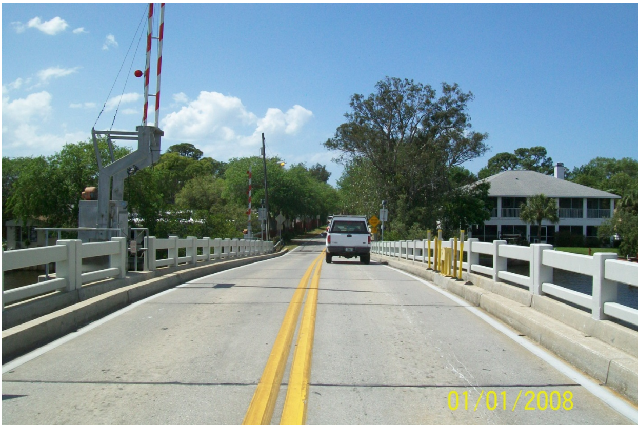
Photo 2: Beckett Bridge – View from Roadway, Looking West
