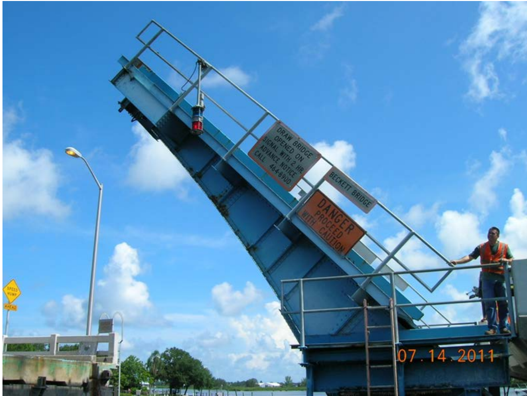
Photo 3: Bascule Leaf in Full Open Position
