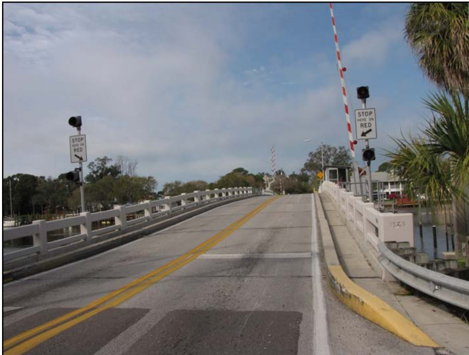
Photo 6: Beckett Bridge (8PI12017) in Pinellas County, Facing Southwest
