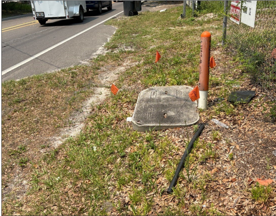
Figure 14. Marked buried utilities on the east side of Forbes Road, facing north.
