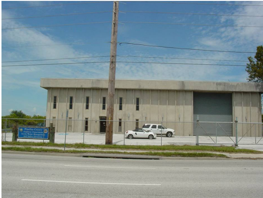
Parcel 26 – PINELLAS COUNTY HIGHWAY DEPT. STORMWATER MANAGEMENT & SAFETY 4051 118 th Avenue N
