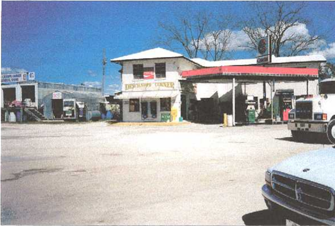
Photo #19: DesChamps Grocery and Gas, Site #4. View to the northwest of petroleum and kerosene tanks.
