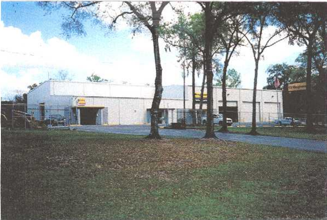
Photo #14: Ringhaver Parts Building, Site #5. View to the northwest.
