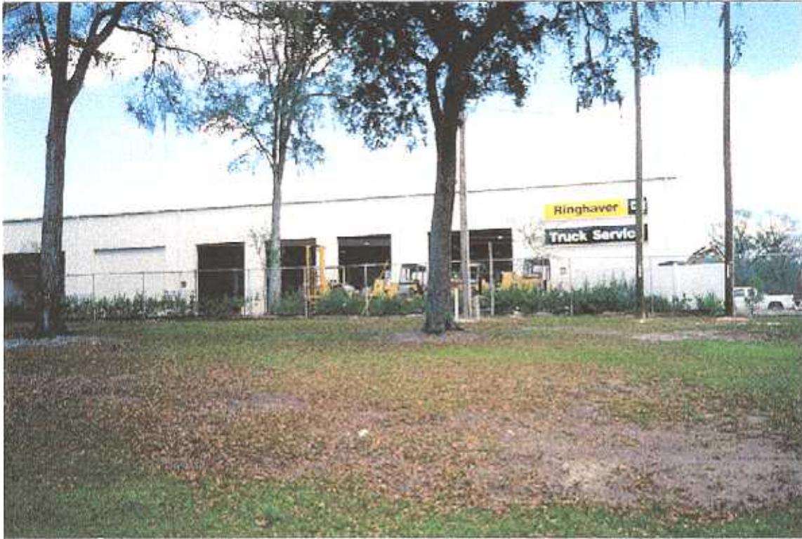
Photo #13: Ringhaver Service Buildings, Site #5. View to the northwest.
