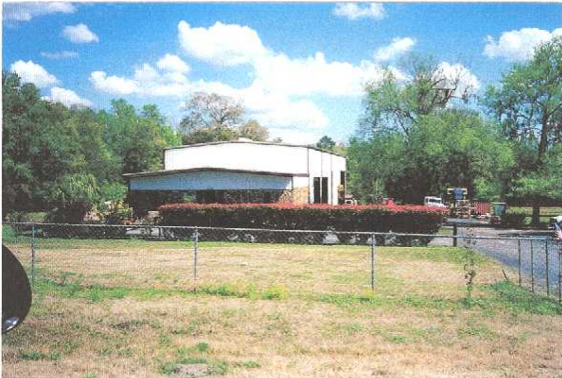
Photo #10: Industrial Welding and Maintenance, Site #I. View to the west from right-of-way.
