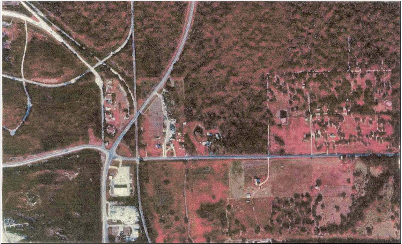
Aerial Photograph of Cobb Road and Yontz Road Intersection Justicia Cooleyi Site is in NE Quadrant of Intersection
