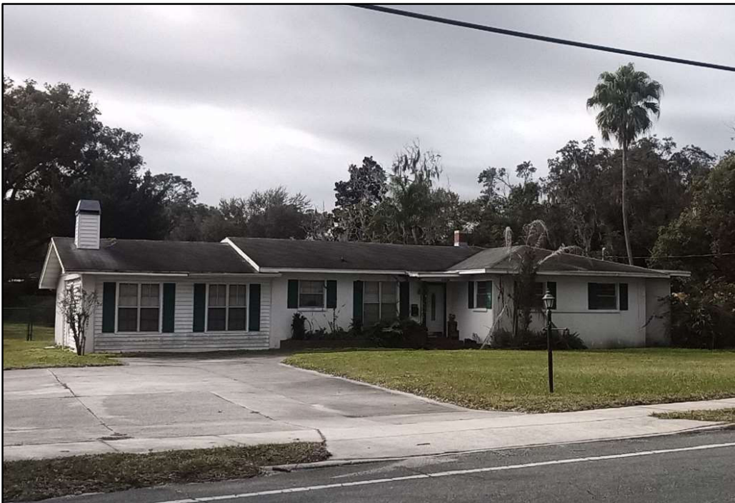
Figure 2: 37108 Meridian Avenue (8PA03651), facing southwest.
