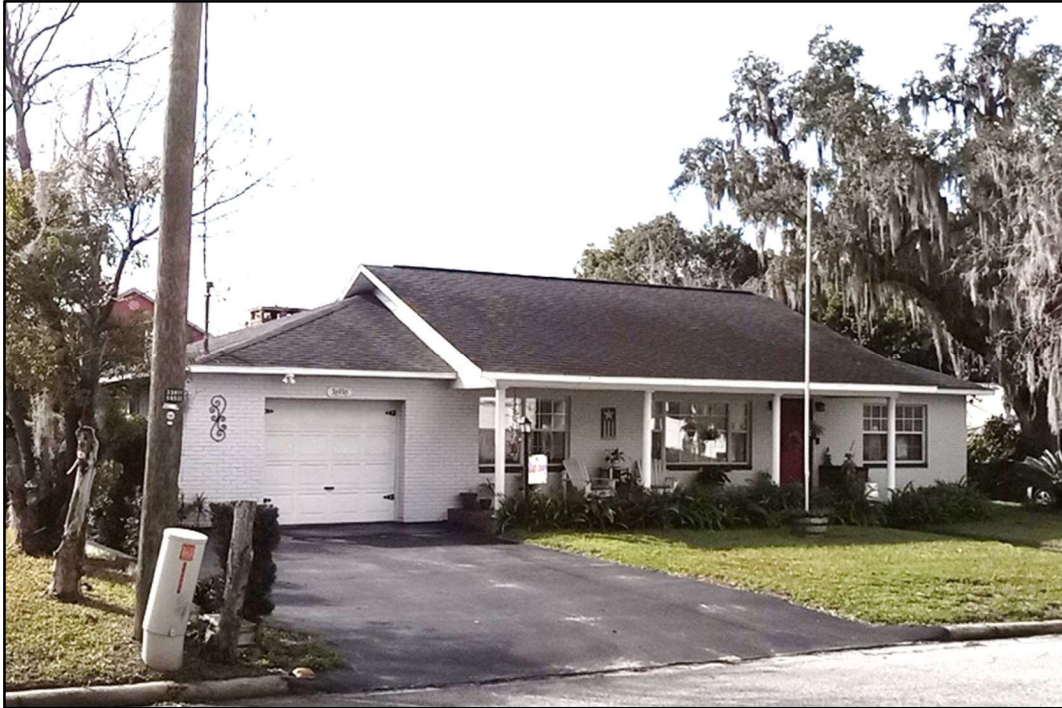
Figure 2: 36936 Suwanee Way (8PA03690), facing southwest.
