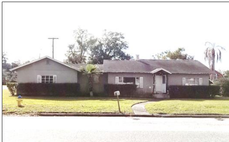
Figure 7.31: 36946 Suwanee Way (8PA03689), facing south.
