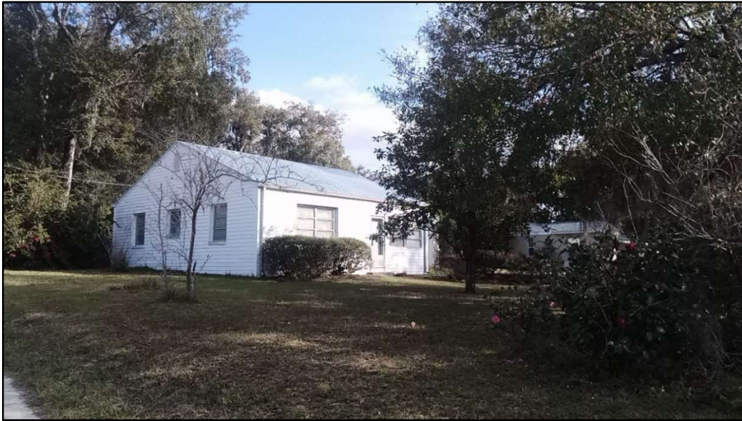
Figure 3: 37011 Church Avenue (8PA03646), facing northeast.
