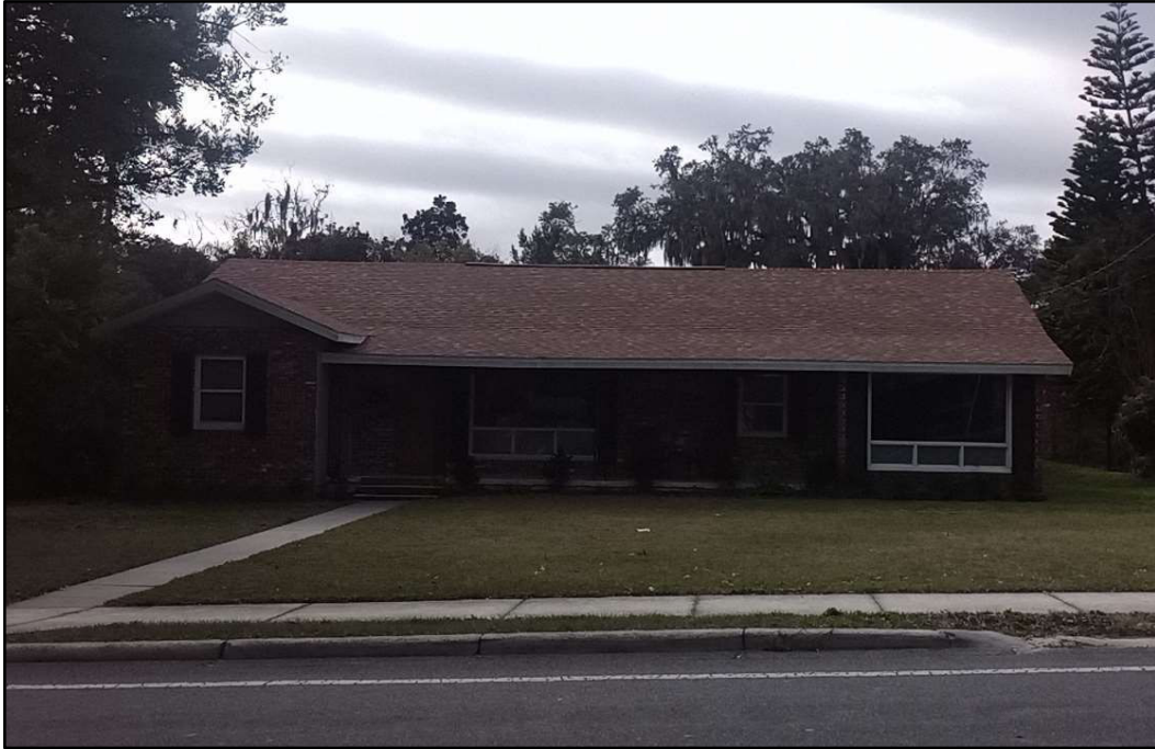
Figure 1: 37048 Meridian Avenue (8PA03650), front elevation, facing south.
