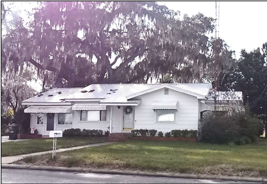
Figure 3: Davis Home (8PA03691), 36926 Suwanee Way, facing southeast.
