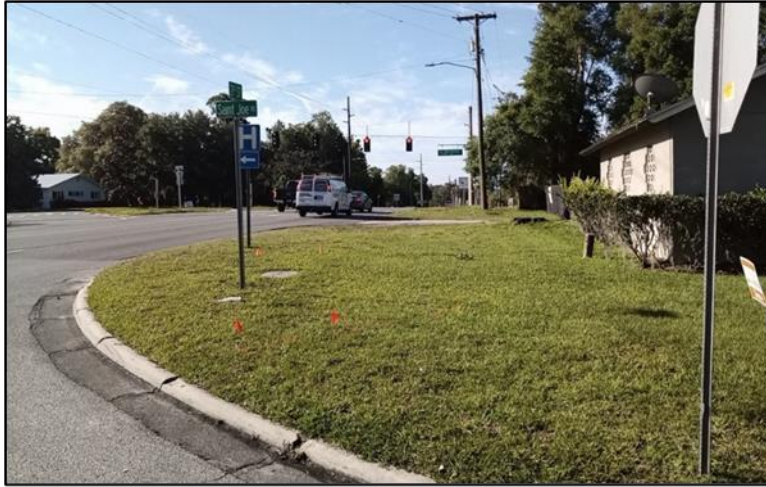
Figure 7.11: Buried utilities along western ROW of intersection of CR 52/21 st Street at Suwanee Way/St. Joe Road, facing south.
