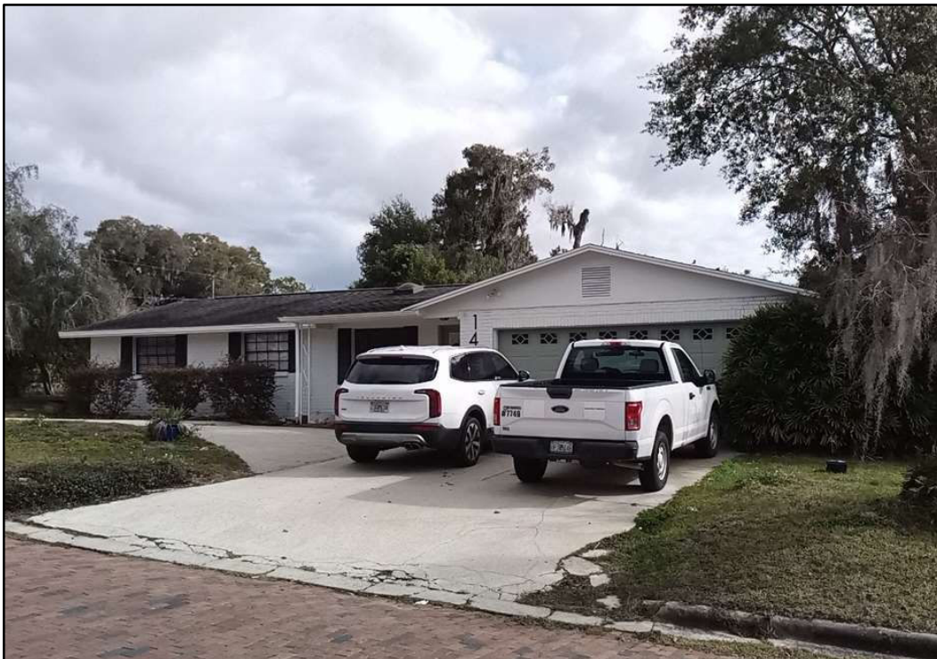
Figure 2: 14234 22 nd Street (8PA03694), facing northeast.
