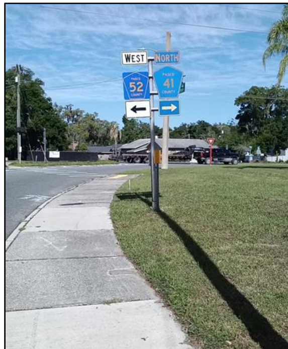
Figure 7.2: Buried utilities and sidewalk along eastern ROW of intersection of CR 52/21 st Street and Meridian Avenue, facing northwest.
