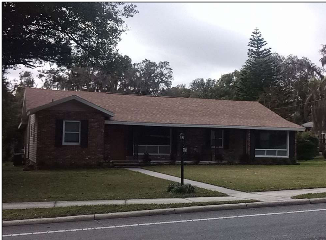
Figure 2: 37048 Meridian Avenue (8PA03650), facing southwest.
