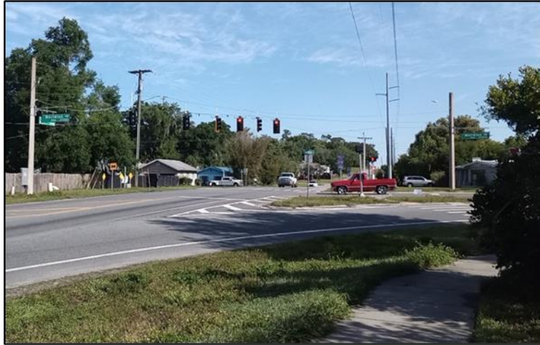
Figure 7.1: Buried utilities and sidewalk along eastern ROW of intersection of CR 52/21 st Street and Meridian Avenue, facing northwest.
