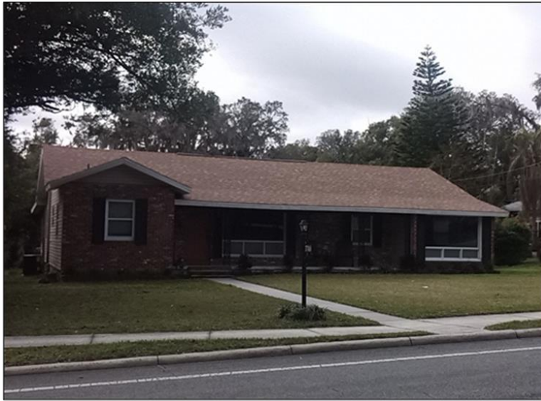
Figure 7.23: 37048 Meridian Avenue (8PA03650), facing southwest.
