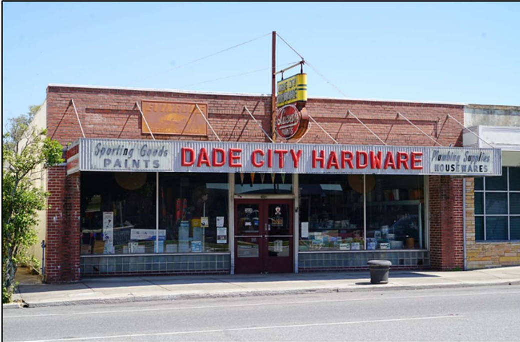
Figure 5: Photograph of Dade City Hardware shortly before its closure (Miller 2017).
