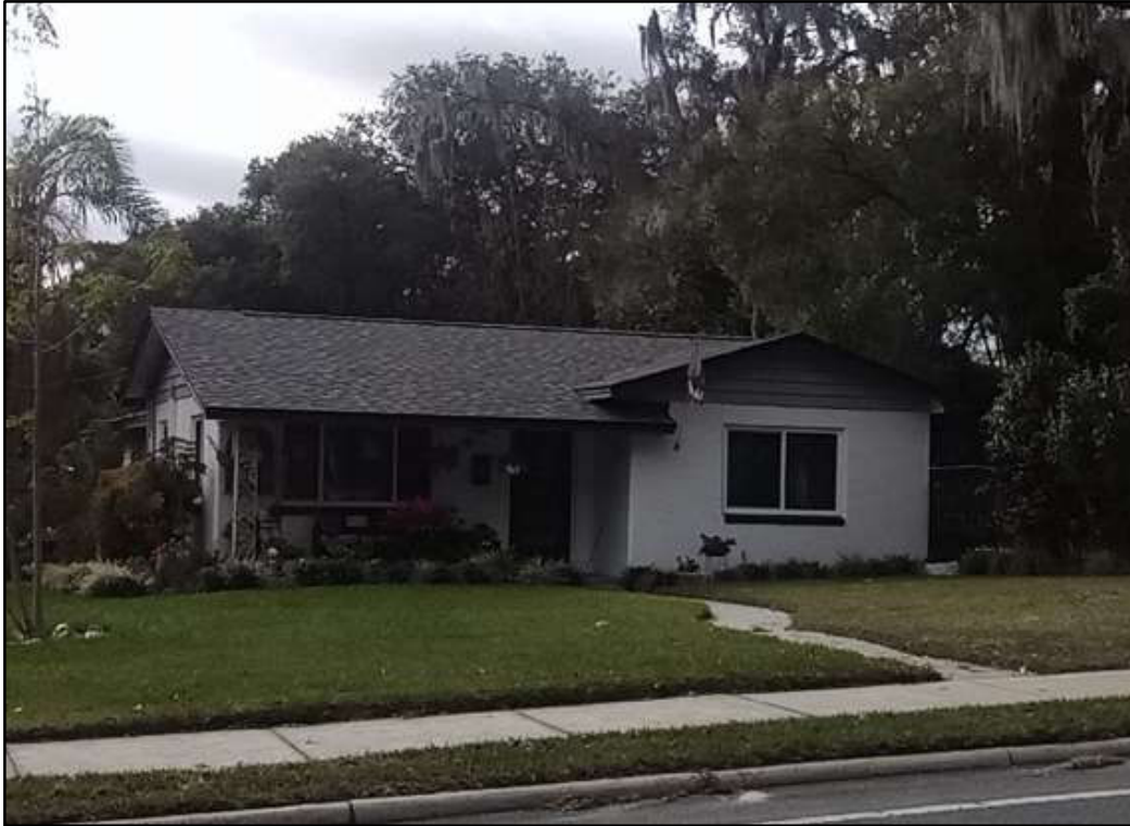
Figure 1: 37038 Meridian Avenue (8PA03649), facing southwest.
