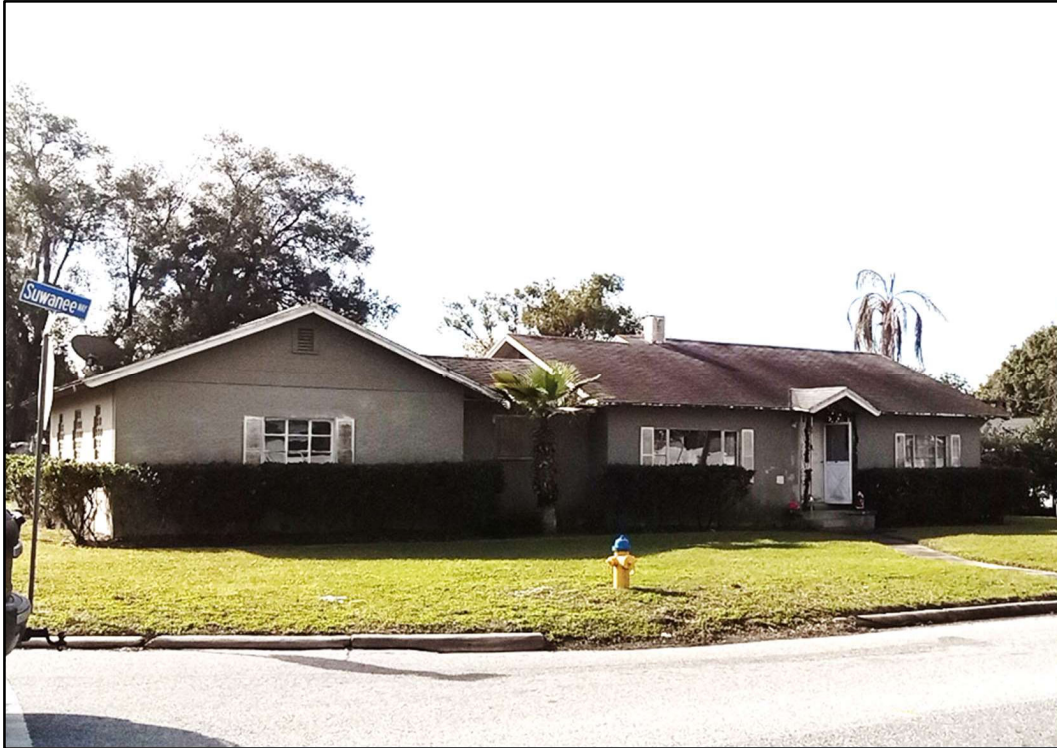
Figure 2: 36946 Suwanee Way (8PA03689), facing southwest.
