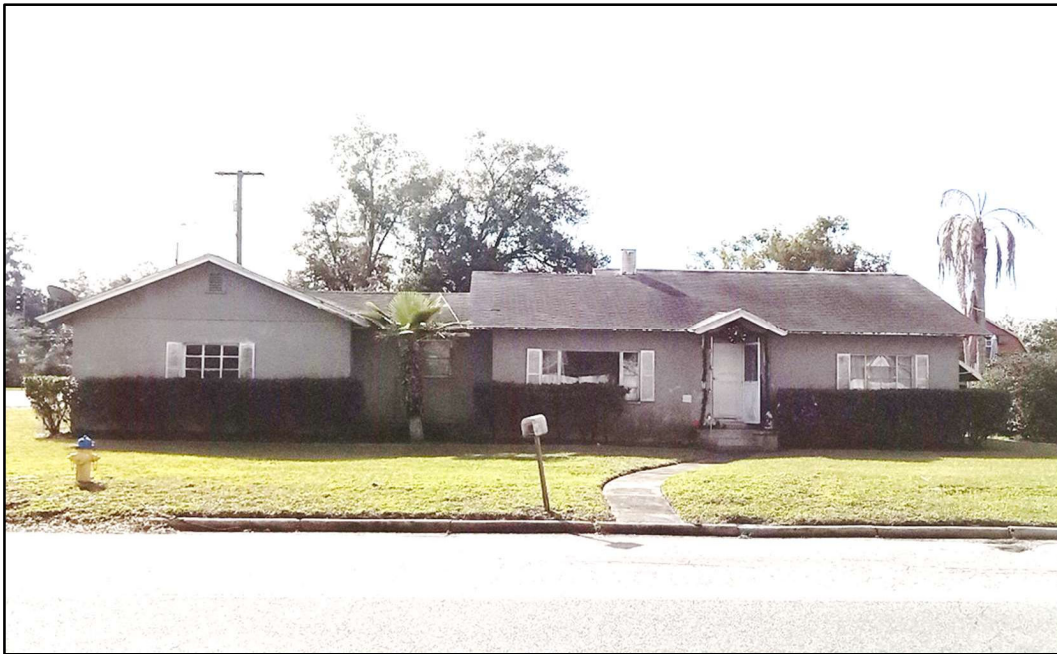
Figure 1: 36946 Suwanee Way (8PA03689), front elevation, facing south.
