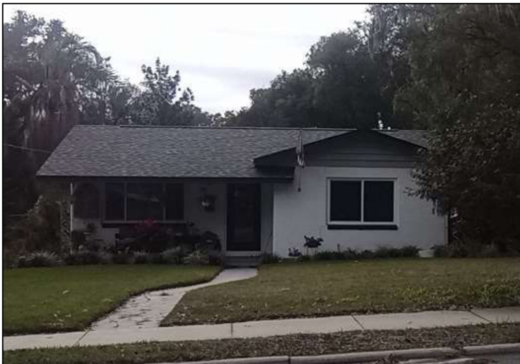
Figure 2: 37038 Meridian Avenue (8PA03649), front elevation, facing south.
