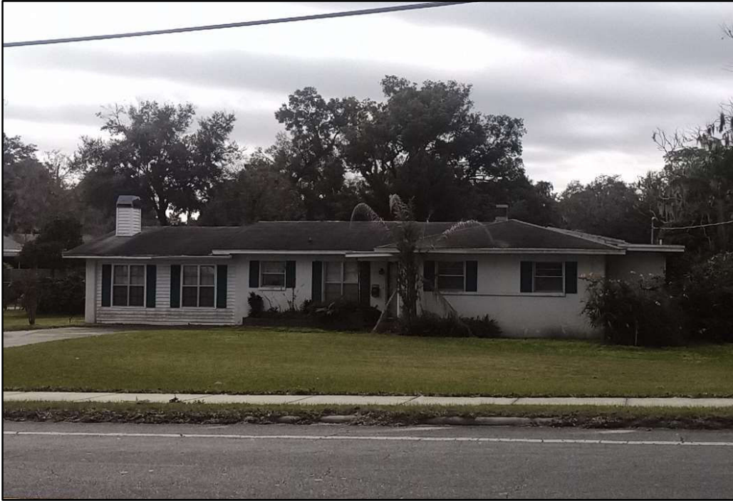
Figure 1: 37108 Meridian Avenue (8PA03651), front elevation, facing south.
