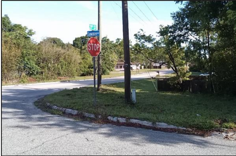
Figure 7.7: Buried utilities along eastern ROW of intersection of CR 52/21 st Street and Suwanee Way/St. Joe Road, facing northwest.
