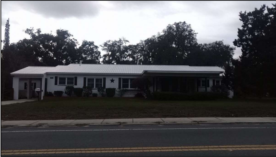
Figure 1: 37016 Meridian Avenue (8PA03647), front elevation, facing south.
