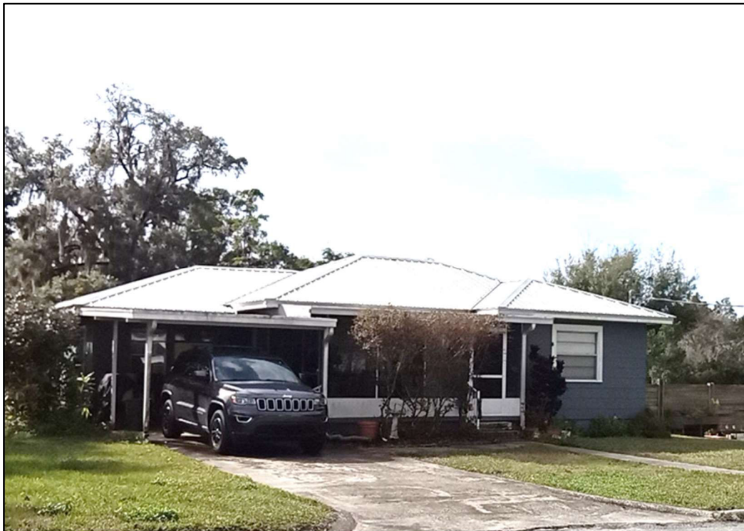
Figure 2: 36918 Suwanee Way (8PA03692), facing southwest.
