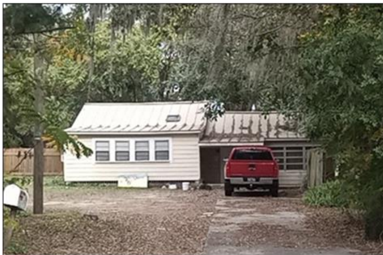
Figure 7.27: 37027 Meridian Avenue (8PA03683), facing north.
