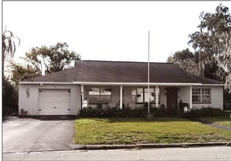
Figure 7.32: 36936 Suwanee Way (8PA03690), facing south.
