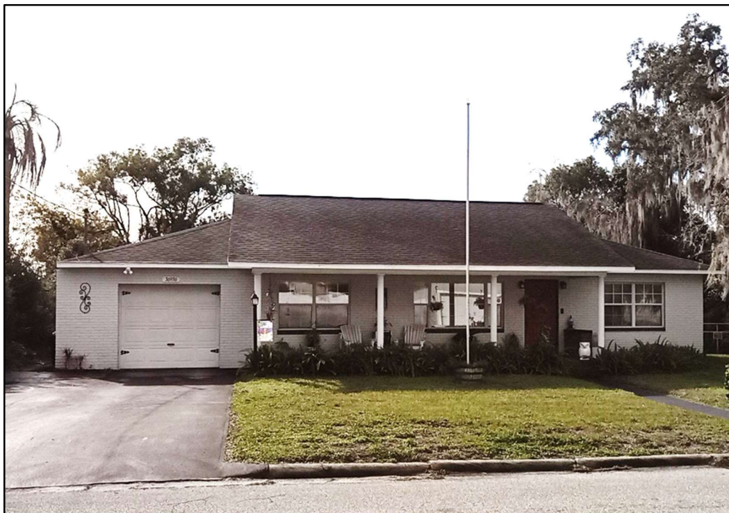
Figure 1: 36936 Suwannee Way (8PA03690), front elevation, facing south.
