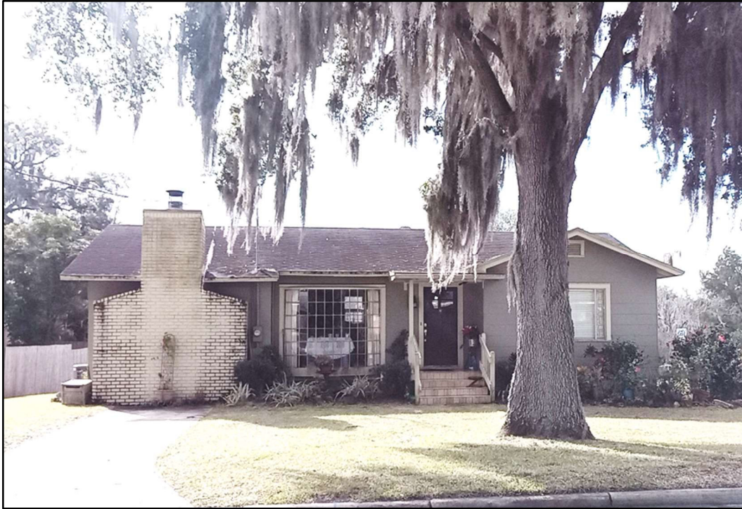
Figure 1: 36910 Suwanee Way (8PA03693), front elevation, facing south.
