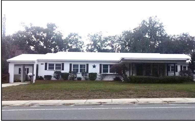
Figure 7.20: 37016 Meridian Avenue (8PA03647), facing south.
