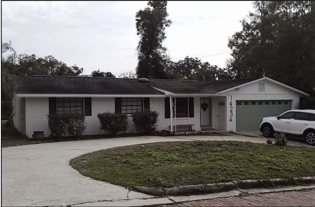
Figure 3: 14234 22 nd Street (8PA03694, facing southeast.
