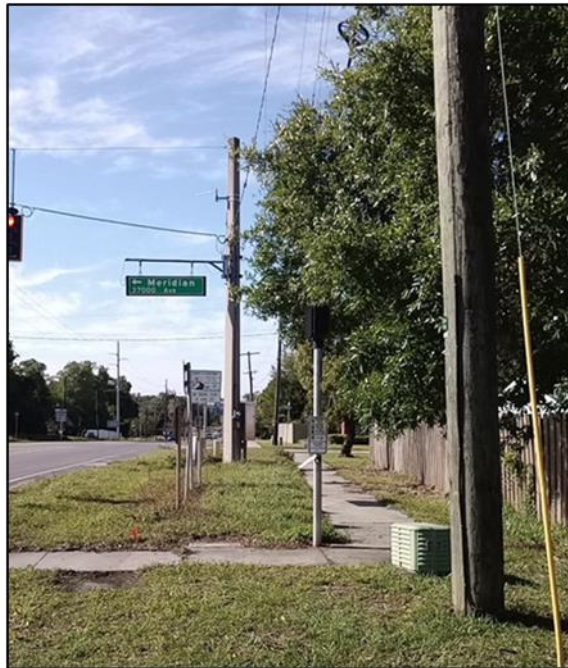
Figure 7.4: Buried utilities and sidewalk along western ROW of intersection of CR 52/21 st Street and Center Avenue/Meridian Avenue, facing south.
