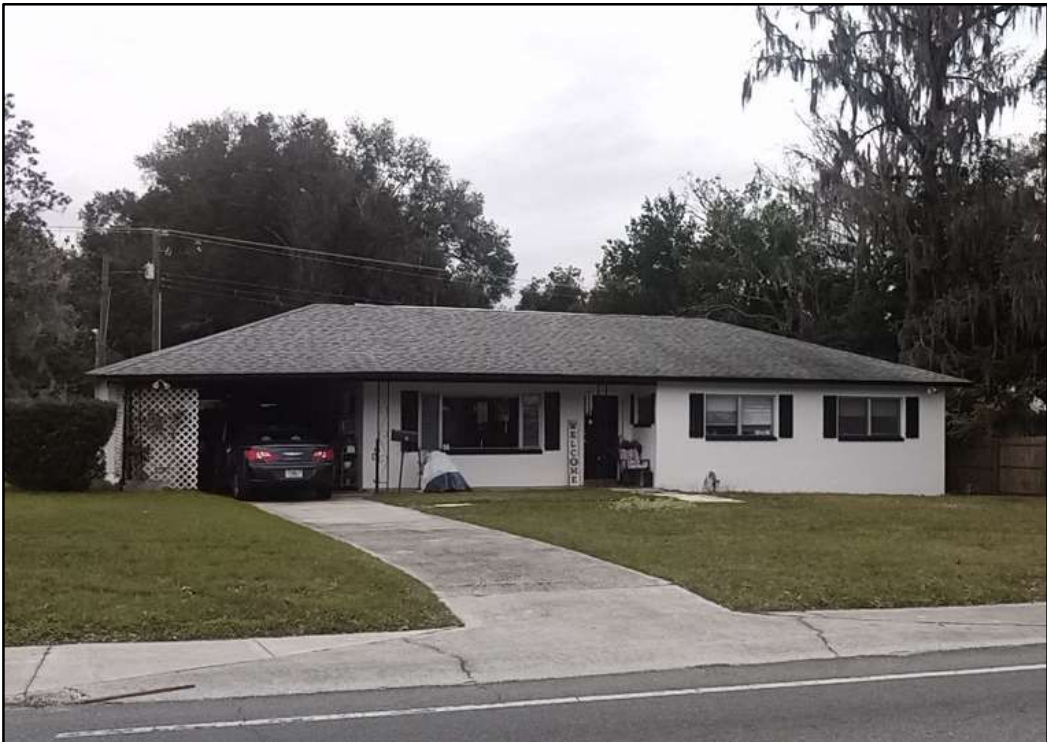
Figure 2: 37017 Meridian Avenue (8PA03684), facing northeast.
