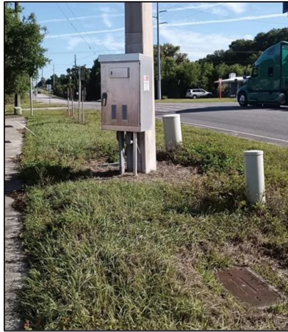
Figure 7.3: Buried utilities along western ROW of intersection of CR 52/21 st Street and Meridian Avenue, facing northeast.
