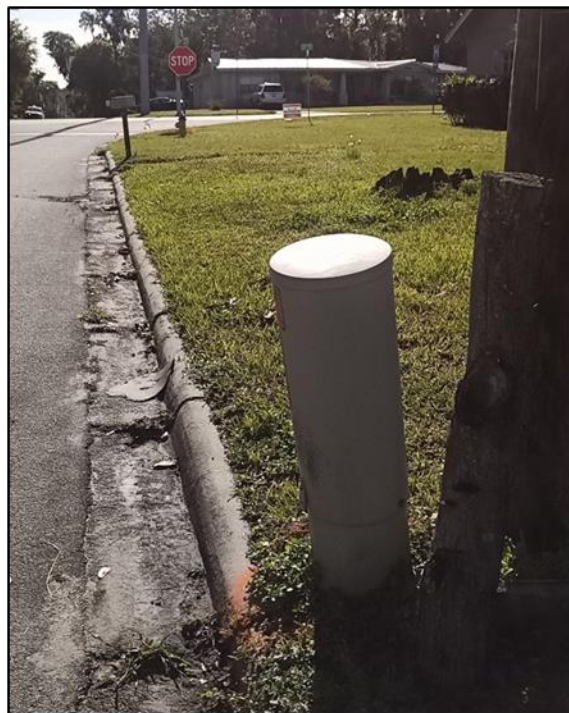
Figure 7.12: Buried utilities along southern Suwanee Way/St. Joe Road ROW, facing east.
