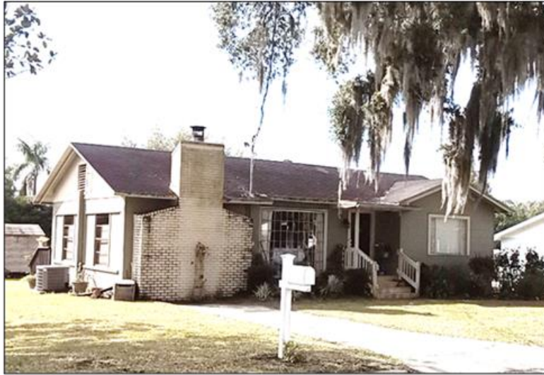
Figure 7.37: 36910 Suwanee Way (8PA03693), facing southwest.
