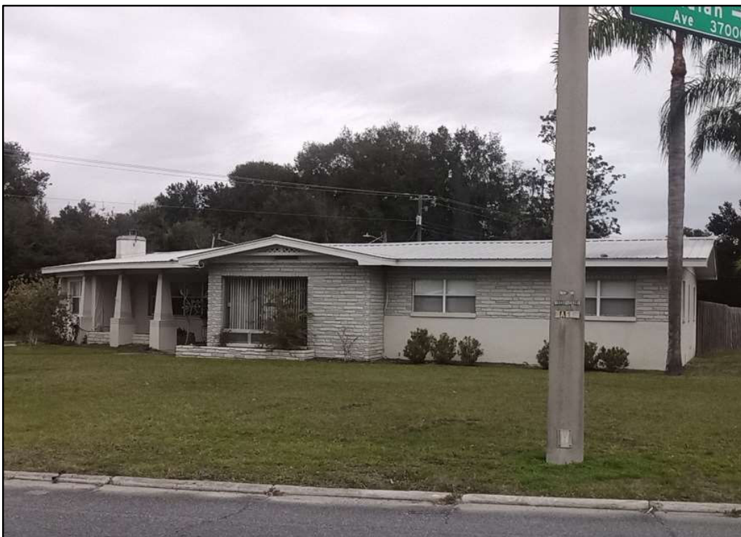
Figure 2: 37009 Meridian Avenue (8PA03685), facing north.
