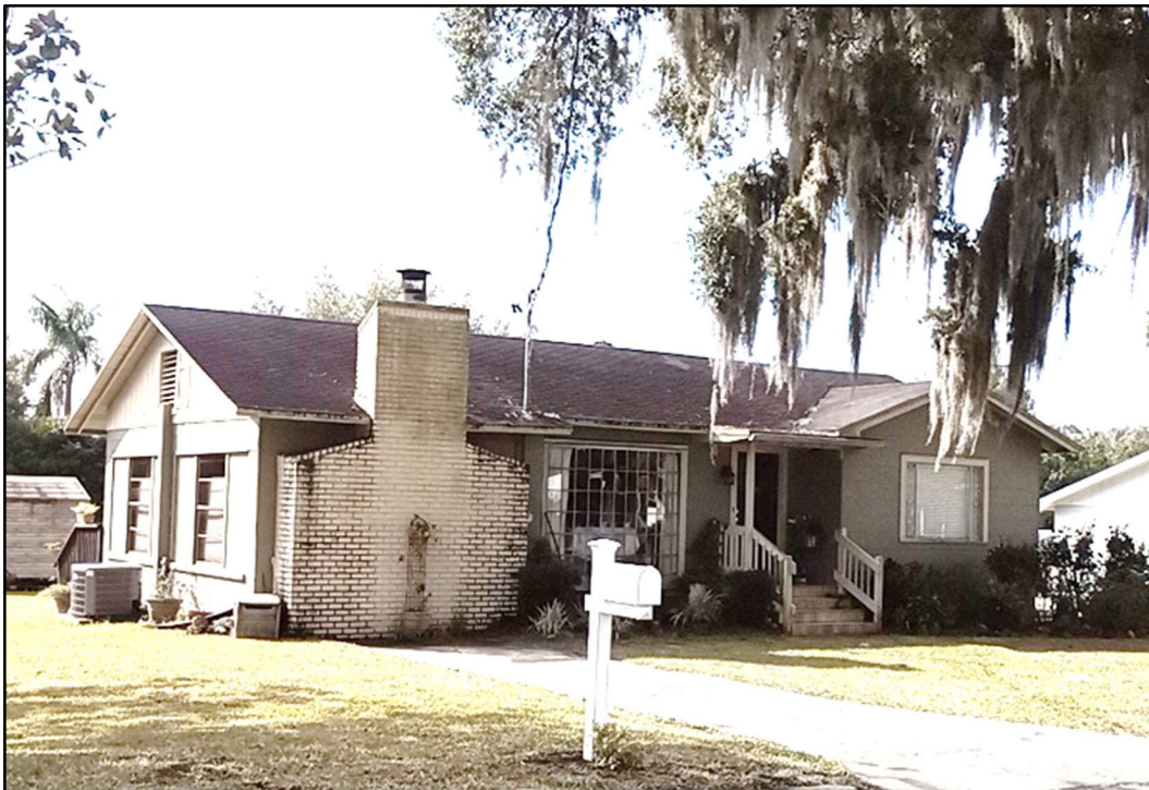
Figure 2: 36910 Suwanee Way (8PA03693), facing southwest.
