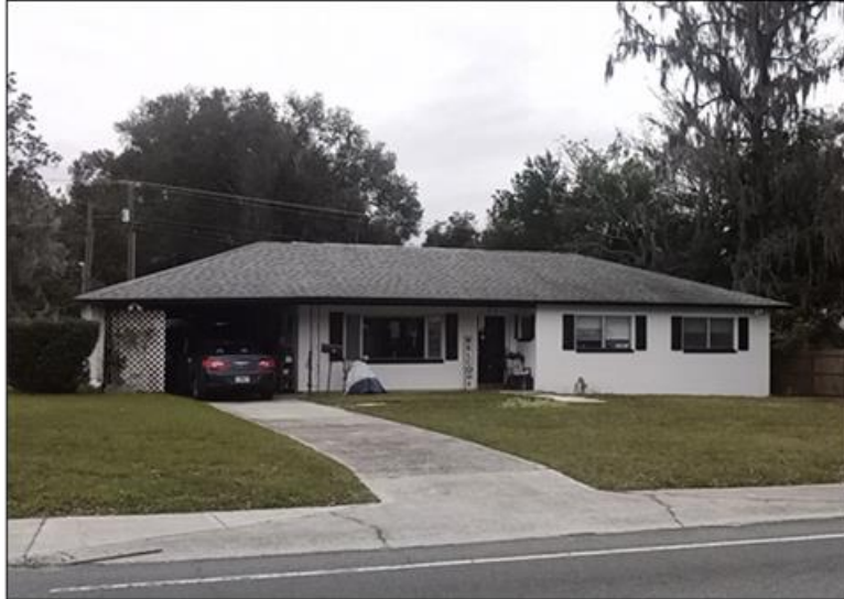
Figure 7.28: 37017 Meridian Avenue (8PA03684), facing northeast.
