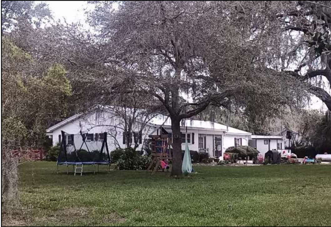
Figure 3: 37016 Meridian Avenue (8PA03647), facing southwest.
