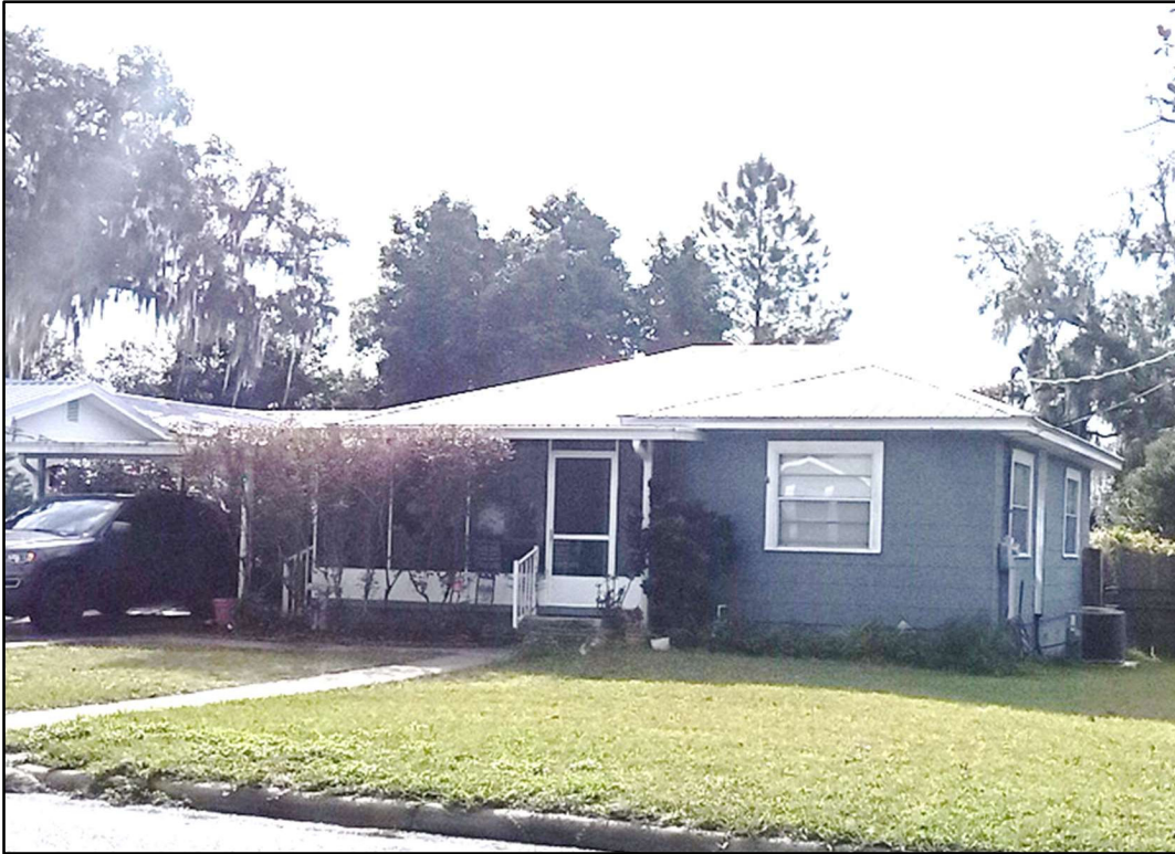
Figure 3: 36918 Suwanee Way (8PA03692), facing southeast.
