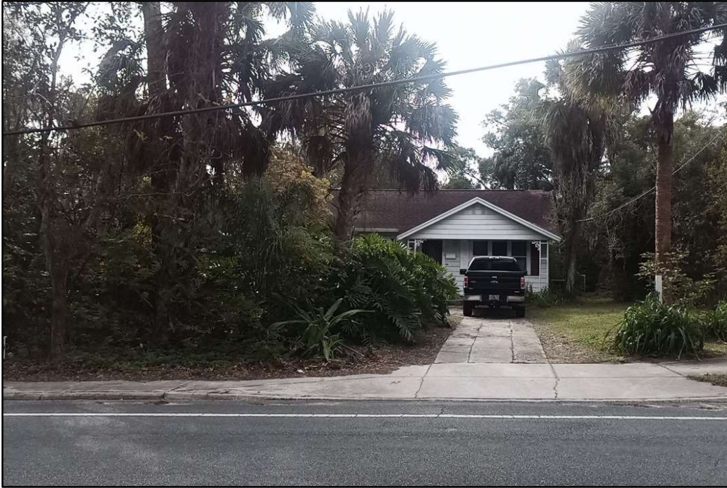
Figure 1: 37030 Meridian Avenue (8PA03648), front elevation, facing south.
