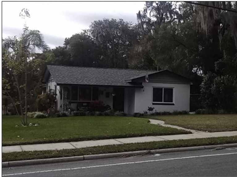
Figure 7.22: 37038 Meridian Avenue (8PA03649), facing southwest.
