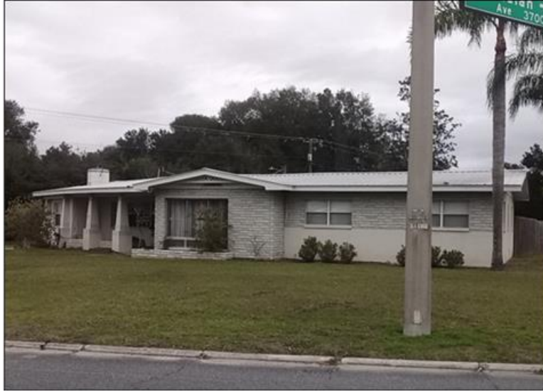
Figure 7.29: 37009 Meridian Avenue (8PA03685), facing north.
