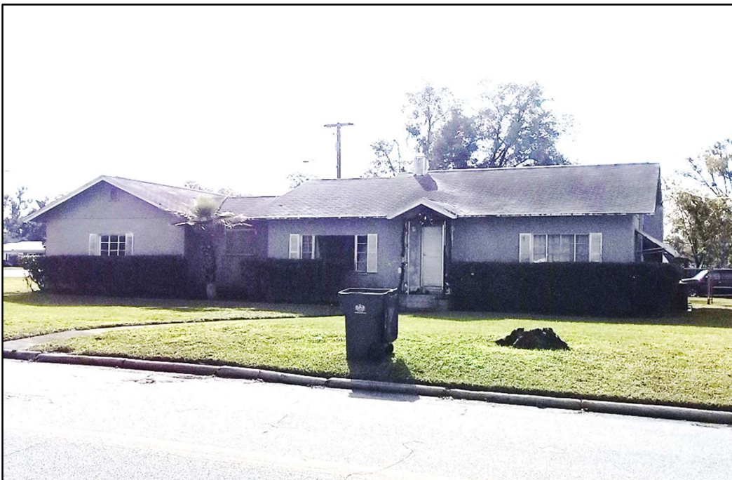
Figure 3: 36946 Suwanee Way (8PA03689). facing southeast.
