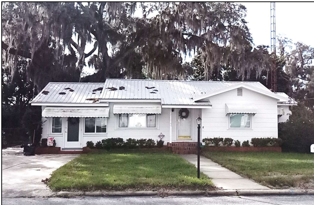
Figure 1: Davis Home (8PA03691), 36926 Suwanee Way, front elevation, facing south.
