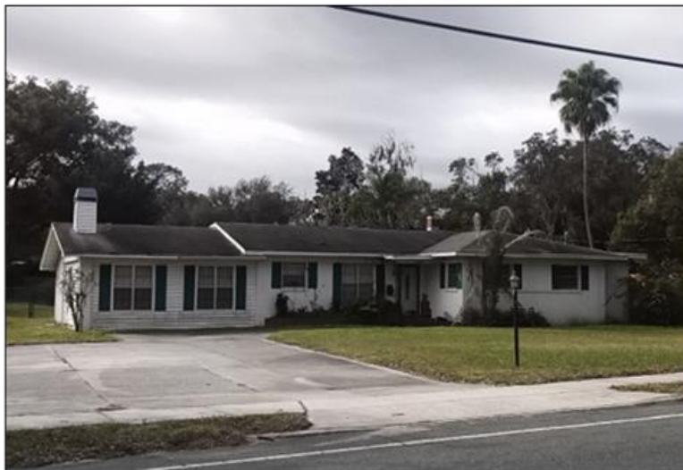
Figure 7.24: 37108 Meridian Avenue (8PA03651), facing southwest.
