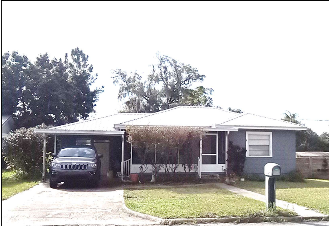
Figure 1: 36918 Suwanee Way (8PA03692), front elevation, facing south.
