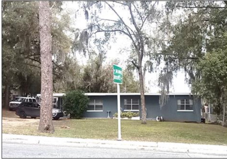
Figure 7.26: 37041 Meridian Avenue (8PA03682), facing north.
