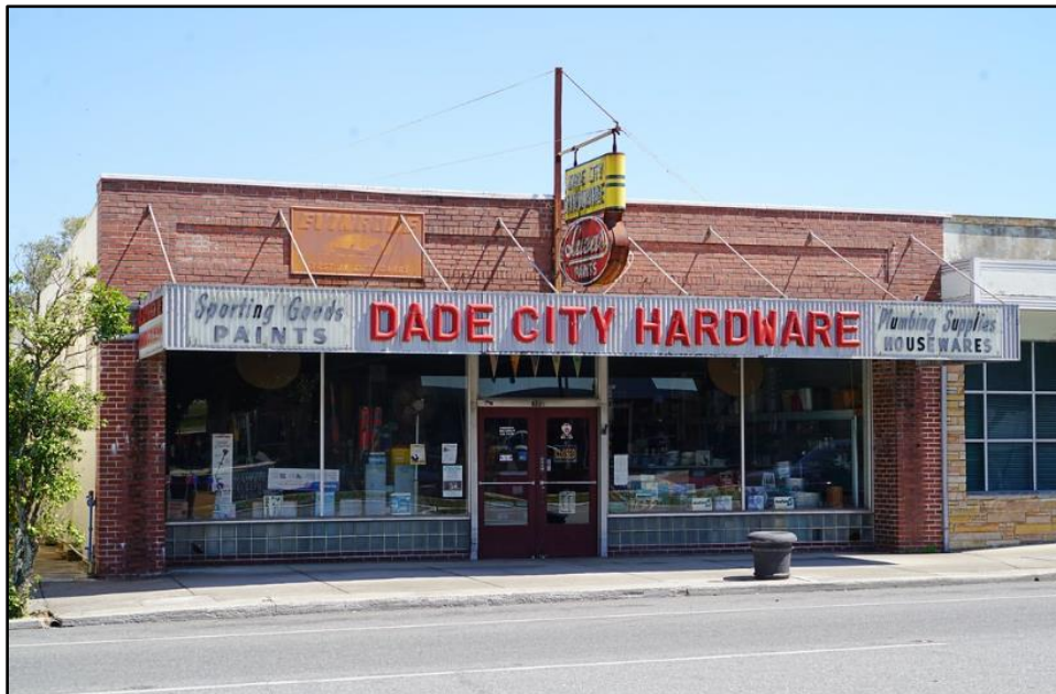
Figure 7.35: Photograph of Dade City Hardware shortly before its closure (Miller 2017).
