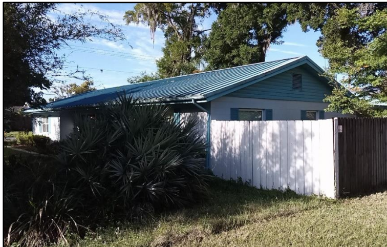
Figure 7.30: 14235 21 st Street (8PA03688), facing southeast.
