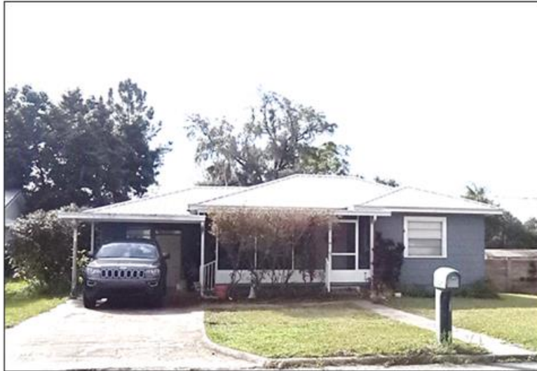
Figure 7.36: 36918 Suwanee Way (8PA03692), facing south.
