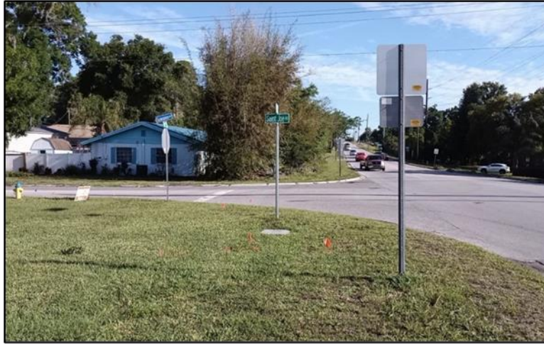
Figure 7.9: Buried utilities along western ROW of intersection of CR 52/21 st Street and Suwanee Way/St. Joe Road, facing north.
