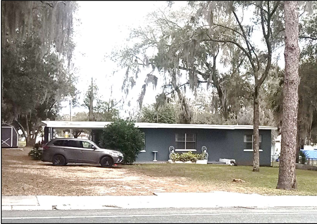
Figure 3: 37041 Meridian Avenue (8PA03682), facing northeast.
