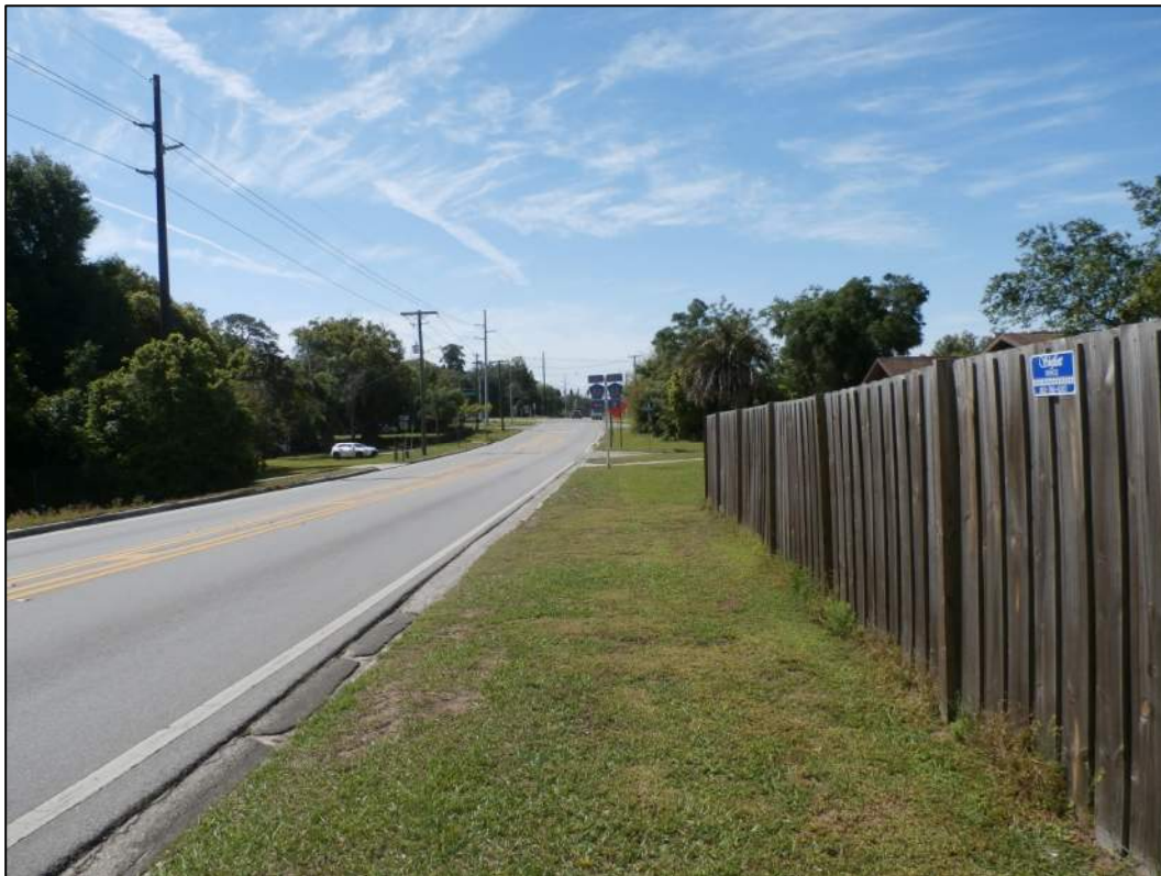
Photo 4: View south along 21 st Street north of Virginia Avenue
