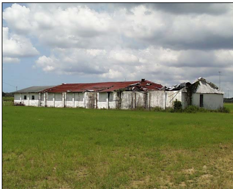
FIGURE 9-20 SITE 8HE410 C.R. 578 CONCRETE BARN, FACING NORTHWEST
