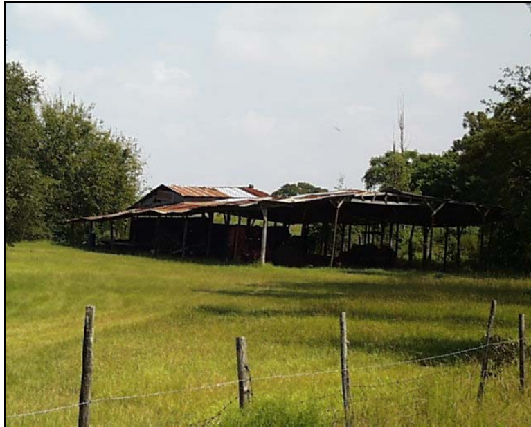
FIGURE 9-16 SITE 8HE408 C.R. 578 POLE BARN, FACING NORTH
