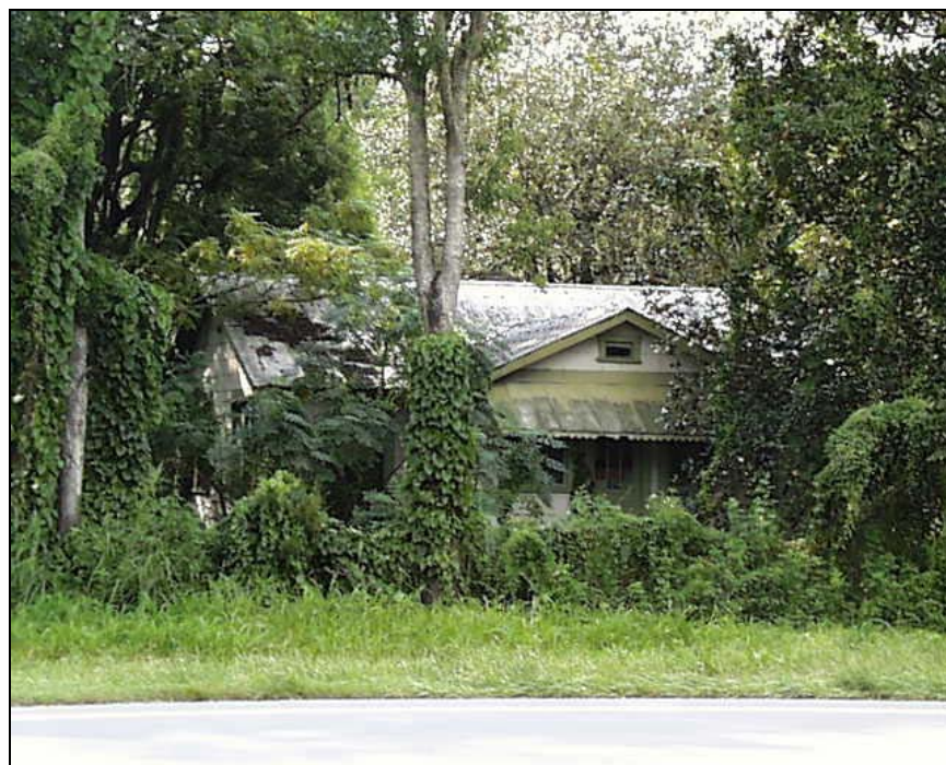
FIGURE 9-30 SITE 8HE384 1219 U.S. 41, FACING NORTHWEST
