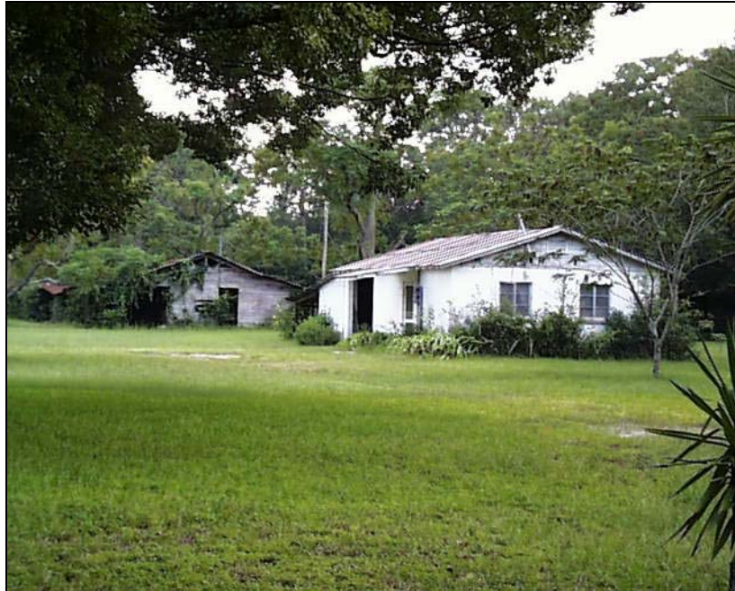
FIGURE 9-27 8PA1300 21220 C.R. 578, FACING SOUTHWEST
