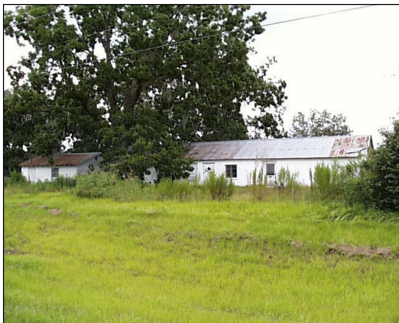
FIGURE 9-21 SITE 8HE411 C.R. 578 MASONRY BUILDING, FACING NORTHWEST
