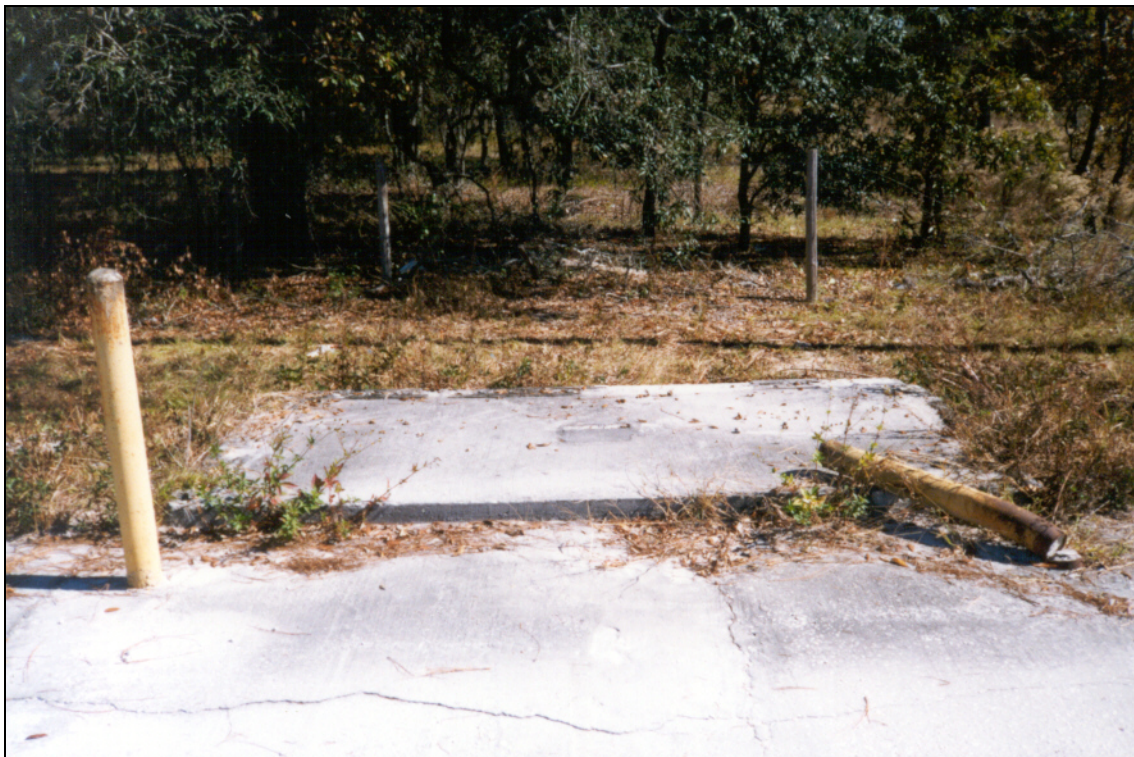
Site No. 26 – Keys Concrete Industries, Inc. – (Former Fuel Pump Stand)
