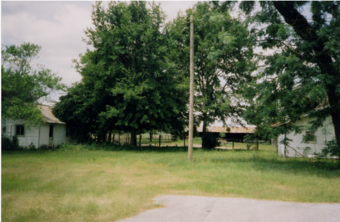
11515 County Line Road Wood Frame Barn and Wood Frame Garage; Pole Barn in Rear
