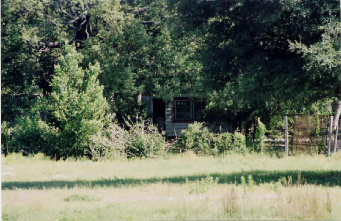
527 Jackson Avenue (Hernando County) Wood Frame House
