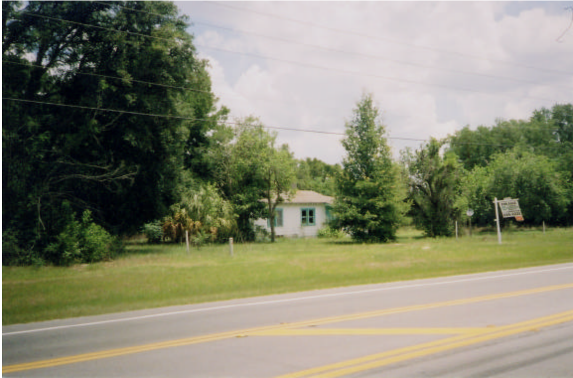
15165 County Line Road - Wood Frame House
