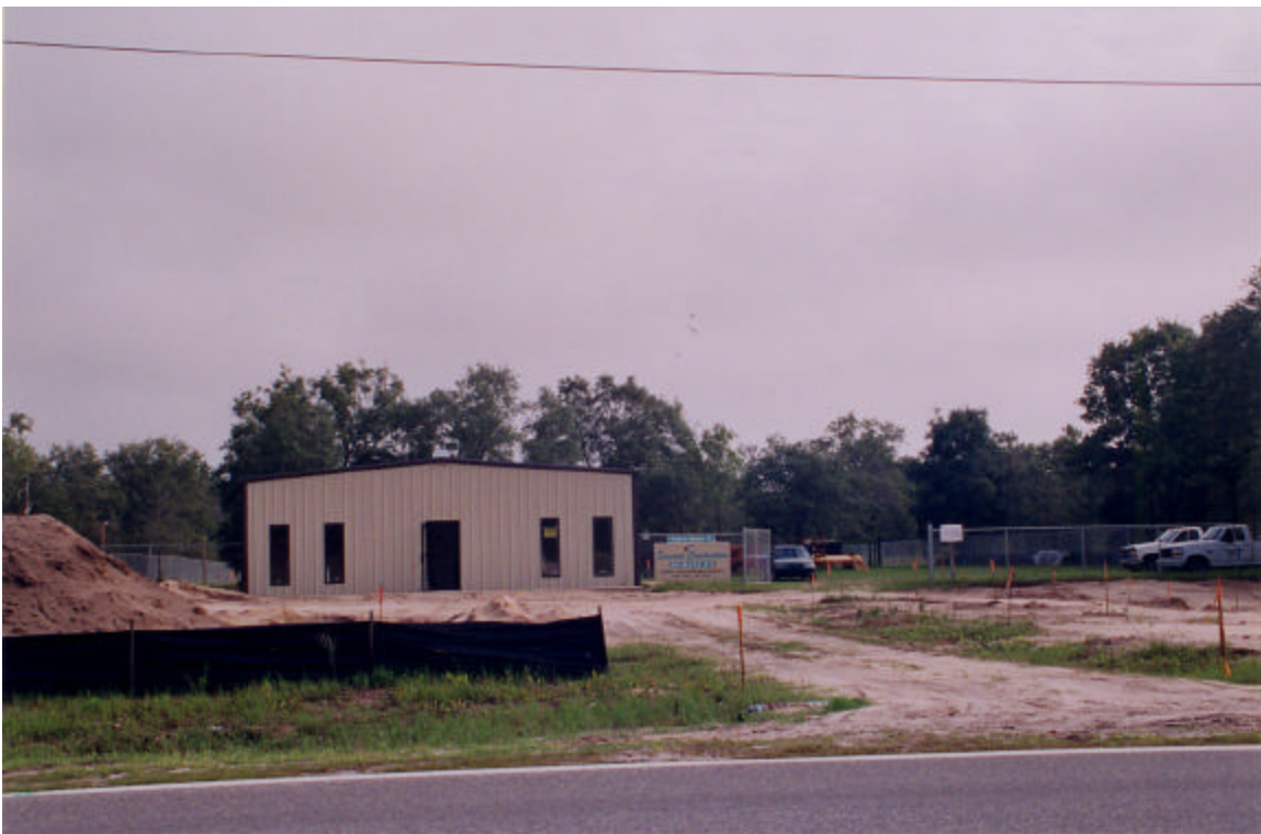
9067 County Line Road (Hernando County) Suncoast Construction Services; Metal Building
