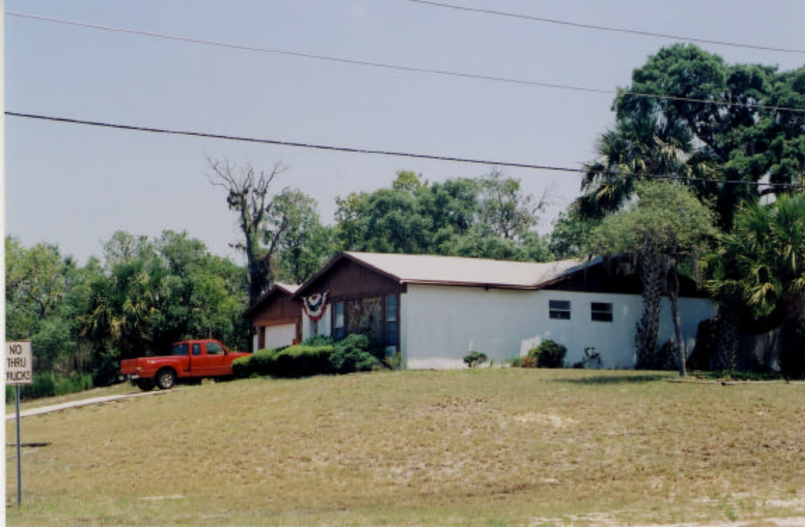
102 Darcoca Avenue (Hernando County) Block House
