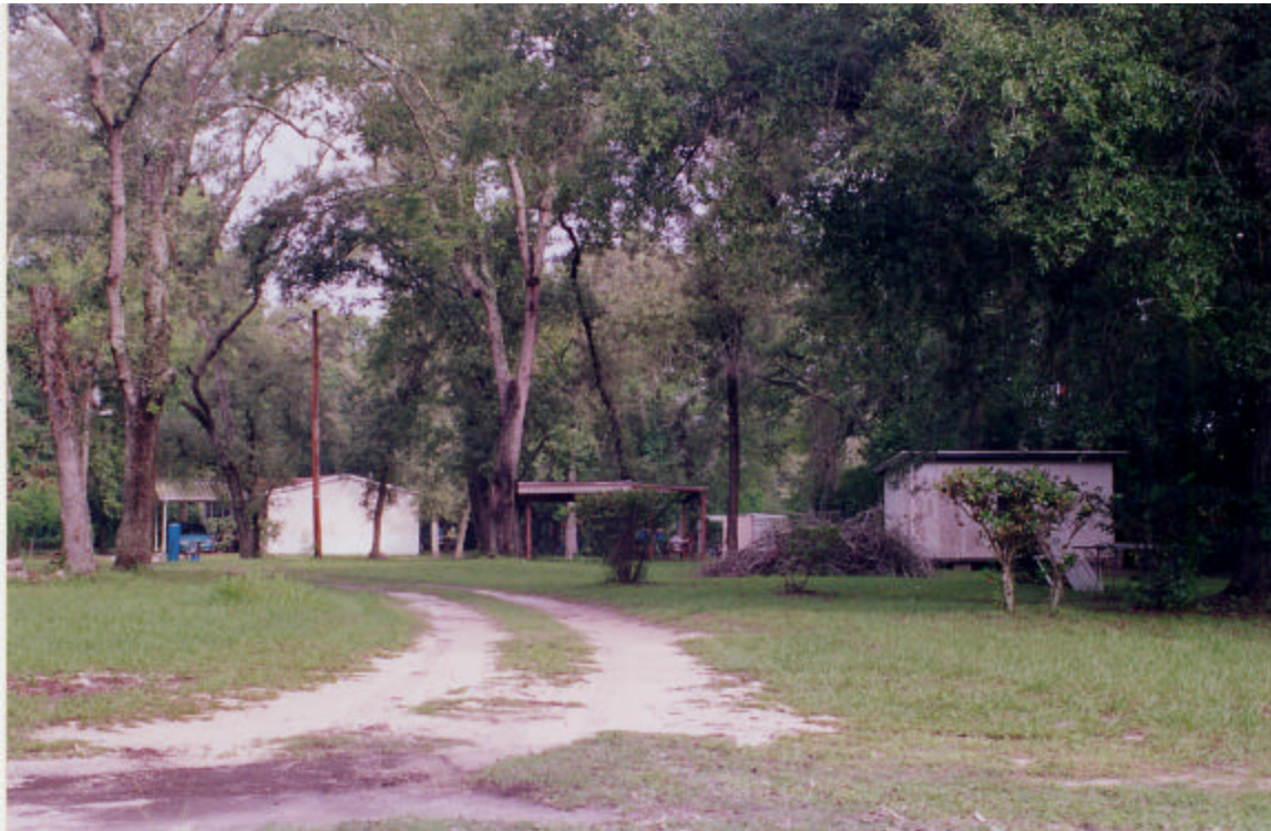
387 Jackson Avenue (Hernando, County) Mobile Home, Storage Unit, and Open Sided Structure
