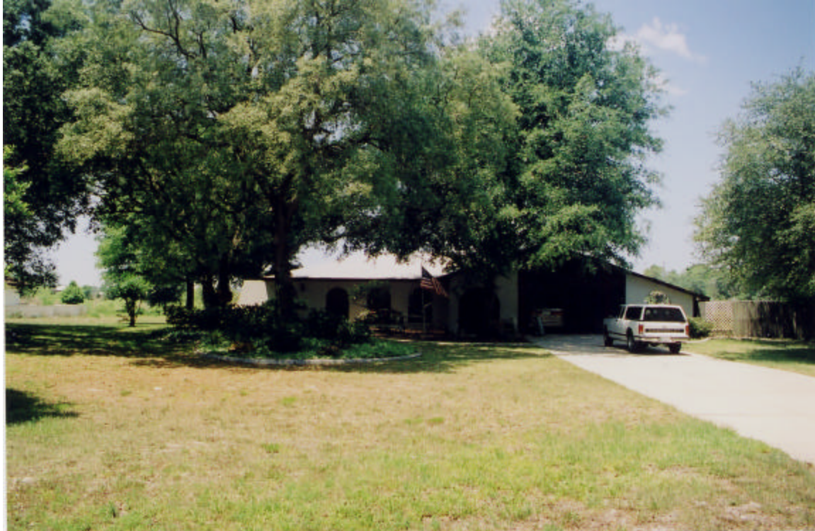
18937 Rolling Rock Drive (Pasco County) Front View Block House
