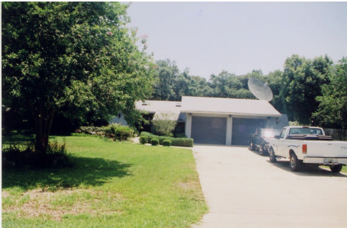
18936 Rolling Rock Drive (Pasco County) Block House
