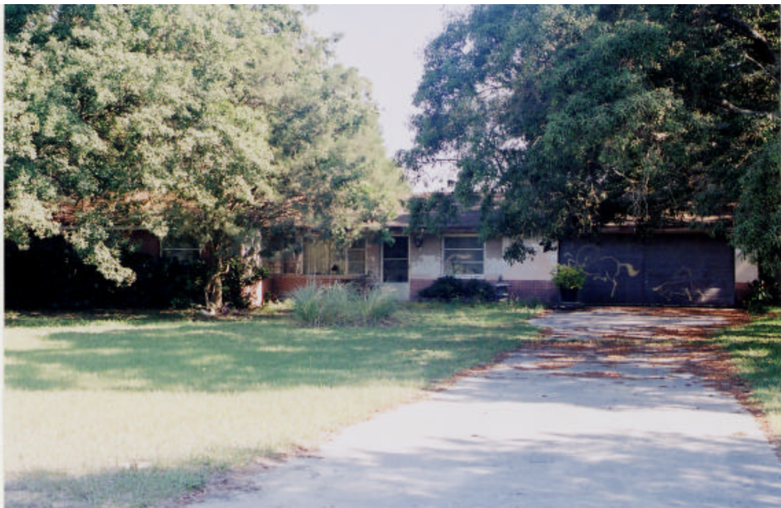
260 Korbus Road (Hernando County) Block House
