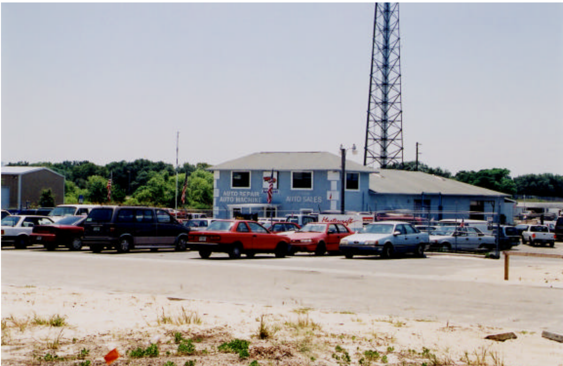
12426 Ramfis Road (Pasco County) Auto Sales & Repair - Potential Contamination Site
