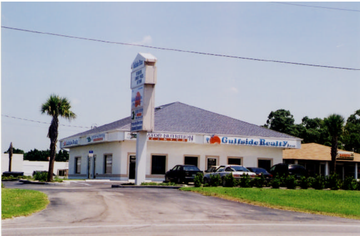
4475 County Line Road (Hernando County) Realty Office/Nutrition Center
