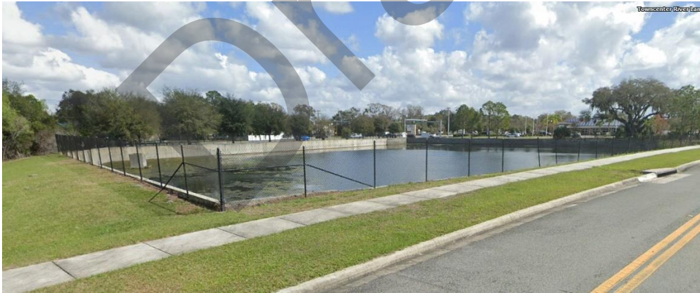
5. OSW-6 facing northeast, located along Town Center River Lane.
