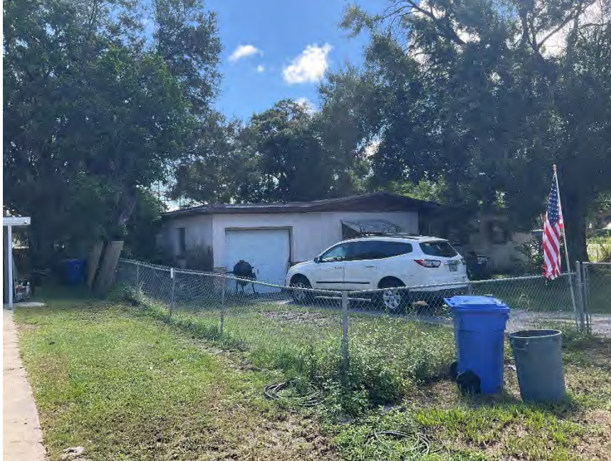
Figure 62. Photograph of 8HI15559-1, facing southeast.
