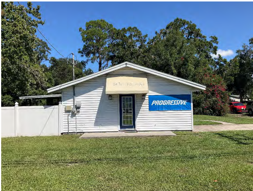
Figure 44. Photograph of 8HI15554-3, facing north.
