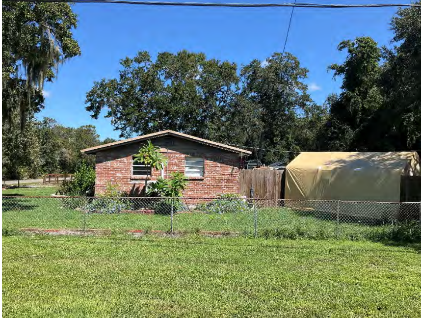
Figure 40. Photograph of 8HI15553-4, facing north.
