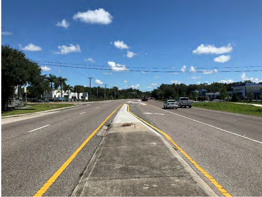
Figure 24. Photograph of 8HI15513- 1, at Water Works Lane, facing northeast.
