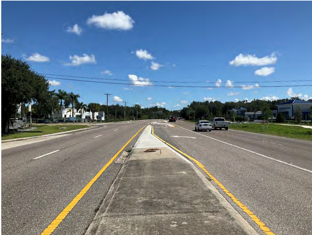
Figure 5. Overview from the western end of the APE facing northeast along Gibsonton Drive.
