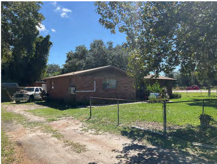
Figure 39. Photograph of 8HI15553-3, facing southeast.
