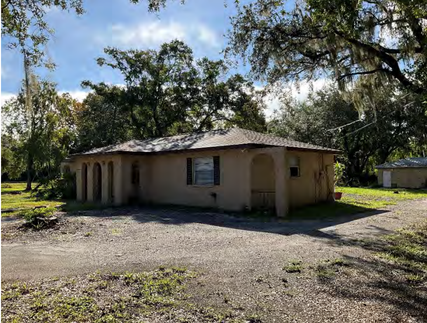
Figure 33. Photograph of 8HI15552-2, facing southeast.
