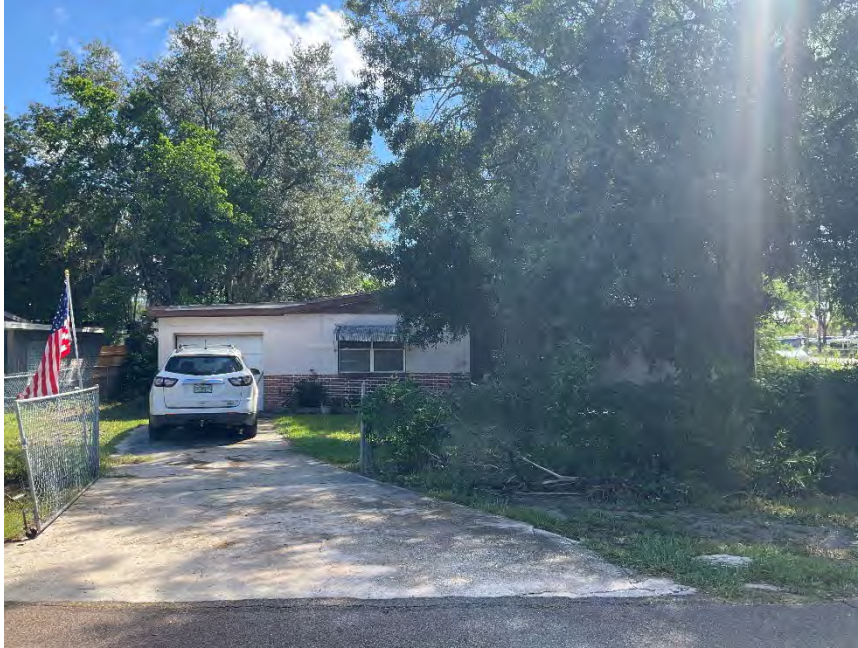
Figure 64. Photograph of 8H115559-3, facing east.
