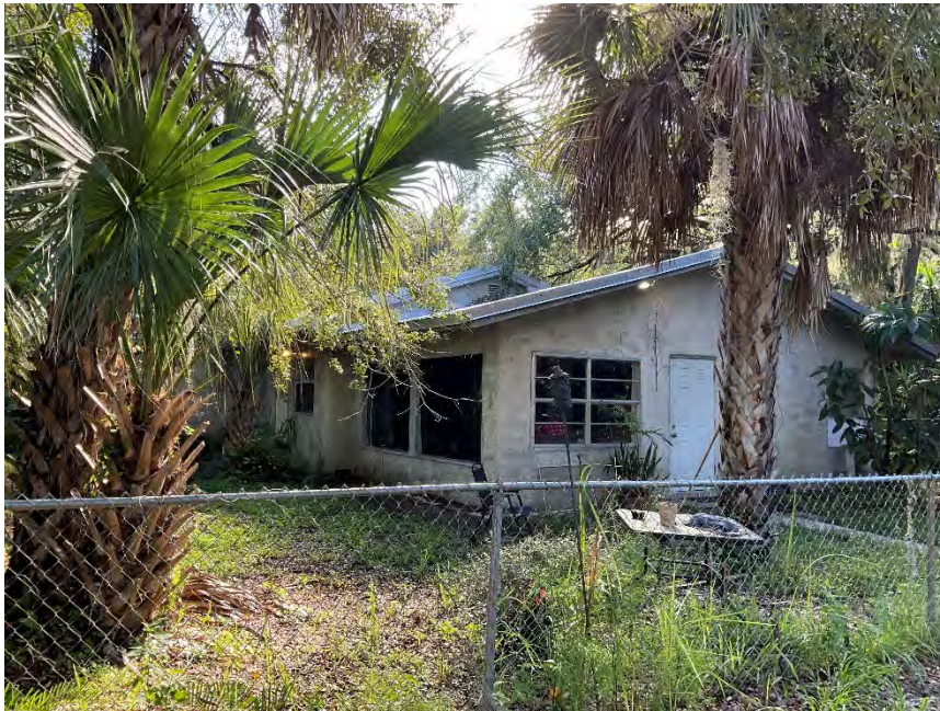
Figure 27. Photograph of 8HI15551–1, facing southeast.
