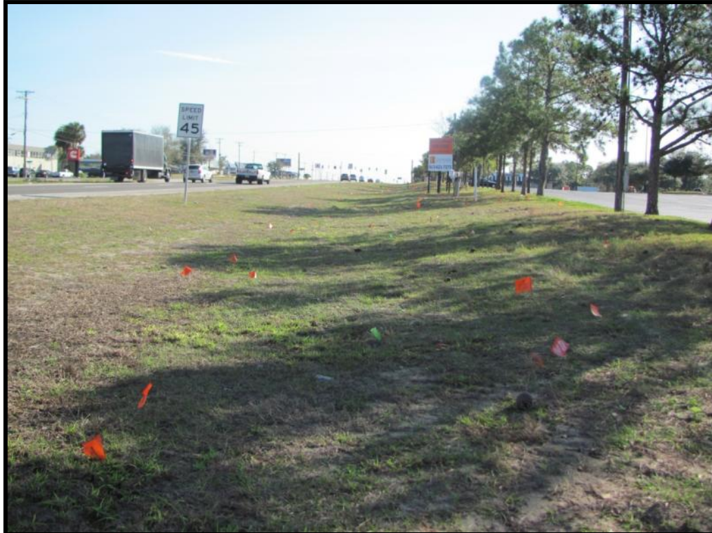
Photo 5.2. Existing conditions along the north side of Hillsborough Avenue. Note placement of utility lines.
