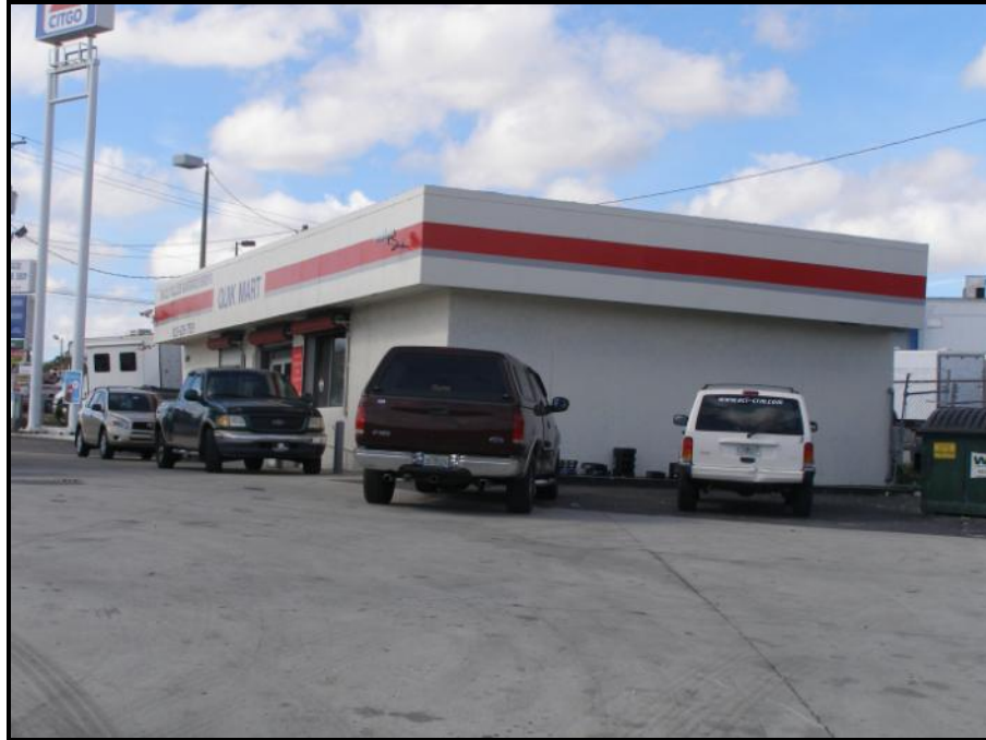
Photo 5.21. North and east elevations of 8HI11680 at 6208 East Hillsborough Avenue.
