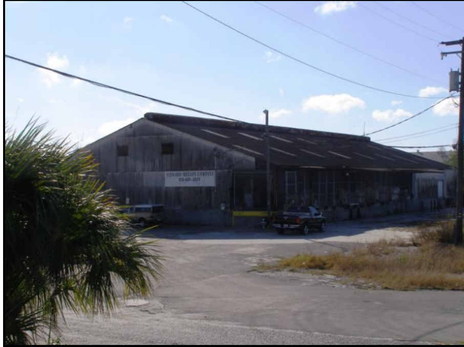
Photo 5.7. North and west elevations of Building 2 (8HI11670) of the Steward-Mellon Company Resource Group (8HI11684) at 5101 East Hillsborough Avenue.
