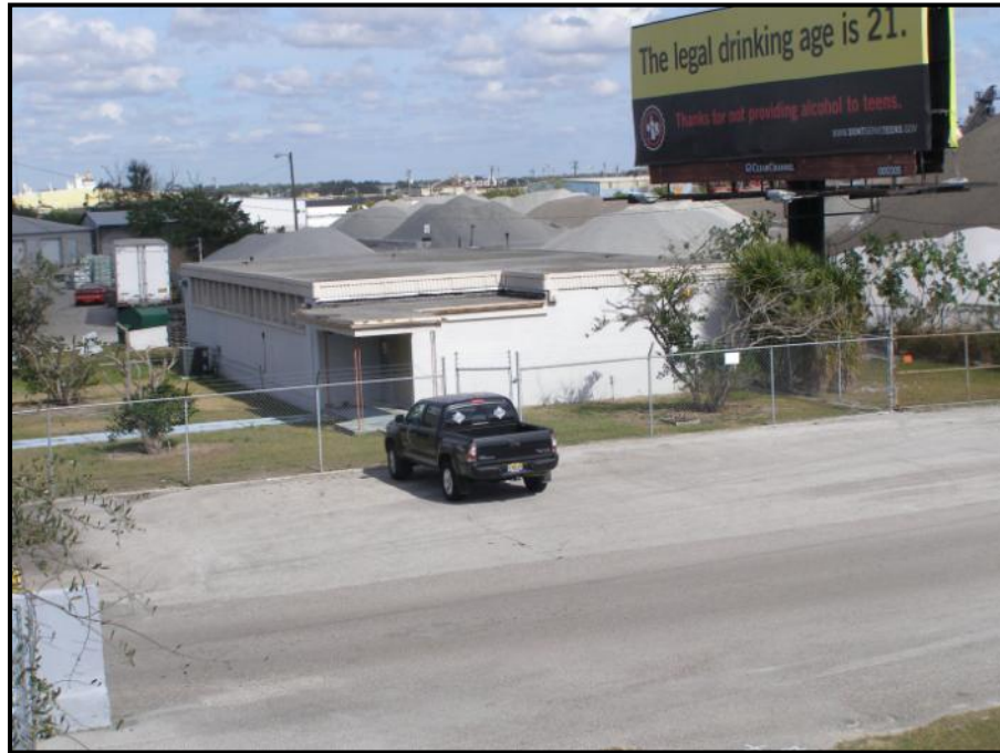
Photo 5.17. South and west elevations of Building 3 (8HI11676) of the Builders Insulation Inc. Resource Group at 5226 East Hillsborough Avenue.
