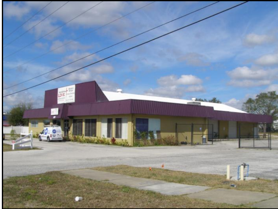
Photo 5.19. South and east elevations of 8HI11678 at 5808 East Hillsborough Avenue.
