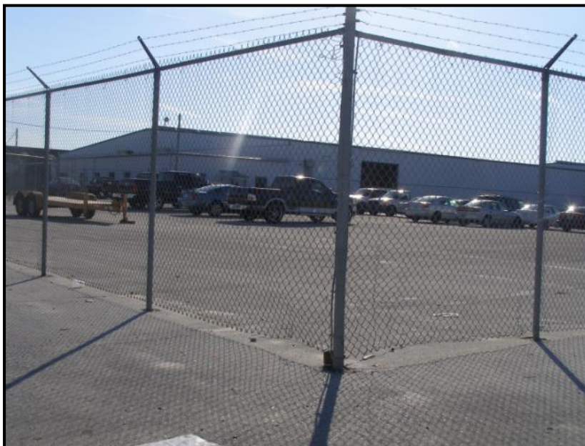
Photo 5.4. East half of the south elevation of 5015 East Hillsborough Avenue, 8HI11668.
