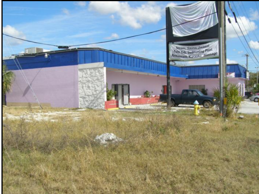
Photo 5.18. South and west elevations of 8HI11677 at 5636 East Hillsborough Avenue.
