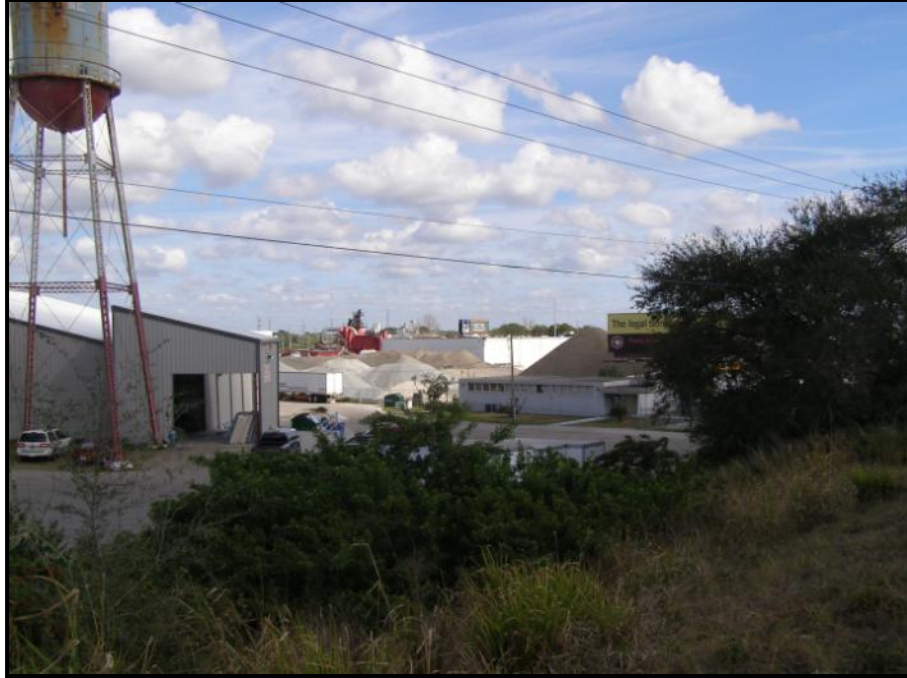
Photo 5.13. General view of the Builders Insulation Inc. Resource Group (8HI11685) at 5226 East Hillsborough Avenue, looking northeast.
