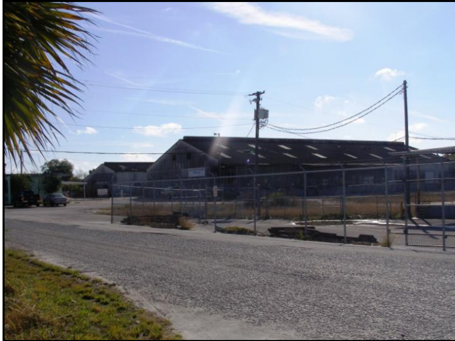
Photo 5.5. General view of the Steward-Mellon Company Resource Group, 8HI11684, at 5101 East Hillsborough Avenue, looking southwest.
