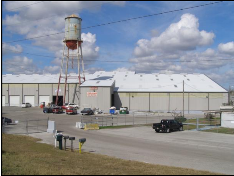
Photo 5.15. North half of the southeast elevation of Building 2 of the Builders Insulation Inc. Resource Group at 5226 East Hillsborough Avenue (8HI11675).
