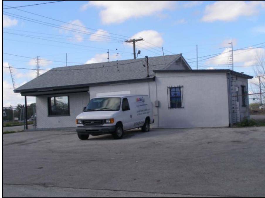
Photo 5.22. North and east elevations of 8HI11681 at 7440 East Hillsborough Avenue.
