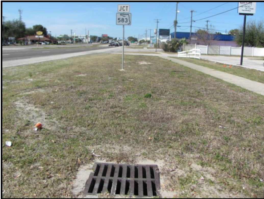
Photo 5.1. Existing conditions along the south side of Hillsborough Avenue. Note sidewalk, driveways, and drainage improvements.
