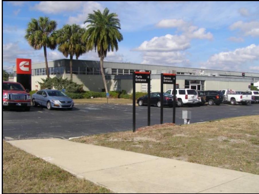
Photo 5.20. South and east elevations of 8HI11679 at 5910 East Hillsborough Avenue.
