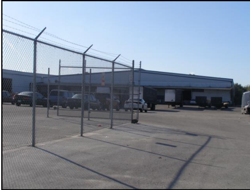
Photo 5.3. West half of south elevation of 5015 East Hillsborough Avenue, 8HI11668.
