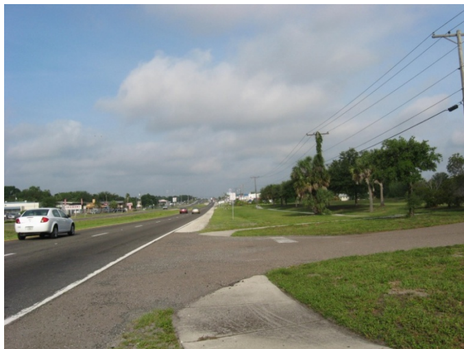
Approximately 0.30 miles west of Orient Road, facing west
