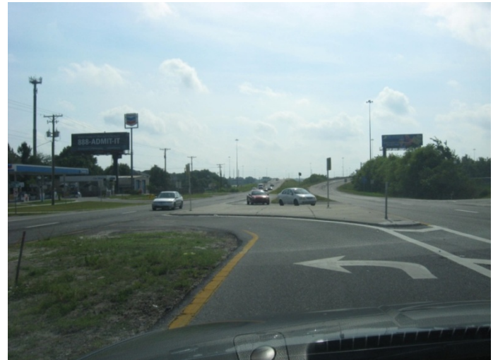
East of Orient Road, looking east towards the ramps to I-4 Ramps
