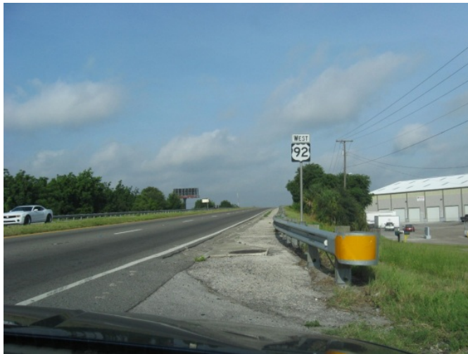
Westbound approach to the bridge, facing west
