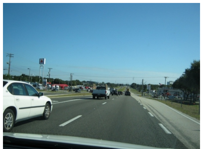
Approximately 350 feet west of Harney Road, facing east
