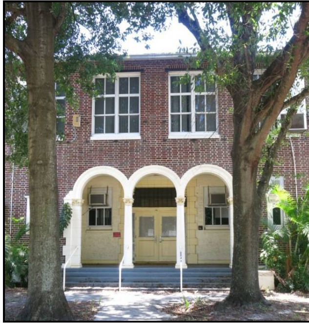
Photo 4.13. The Norwood School (8PI00714) at 2154 27th Ave. N., facing south
