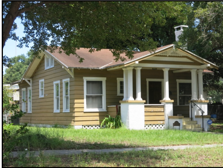
Photo 4.3. The residence at 1911 Burlington Ave. N. (8PI07272), facing northeast.
