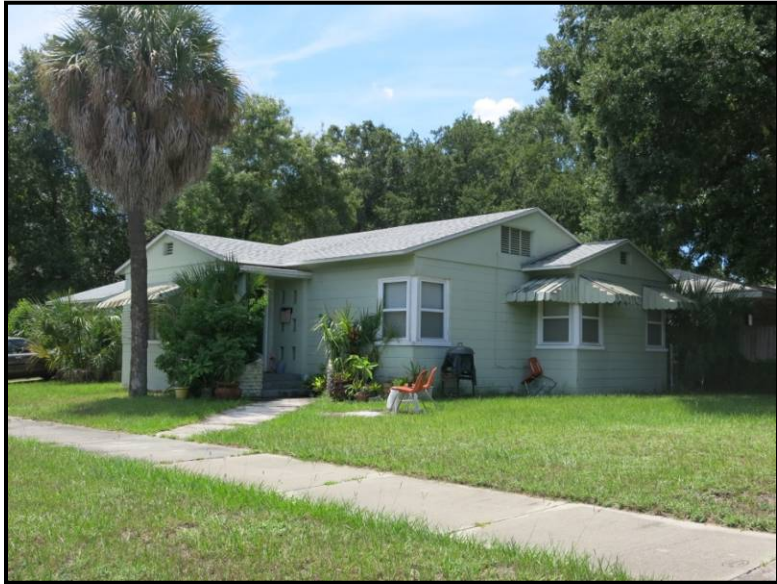
Photo 4.9. The residence at 230 19th St. N. (8PI11102), facing southwest.
