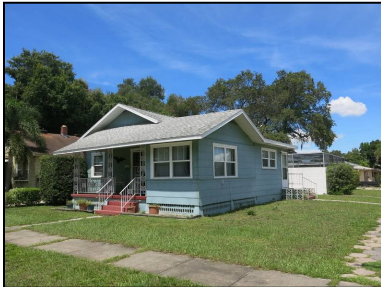
Photo 4.4. The residence at 7105 7th Ave. N. (8PI07410), facing northwest.
