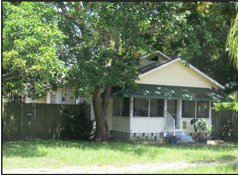
Photo 4.5. The residence at 2101 8th Ave. N. (8PI07502), facing northwest.
