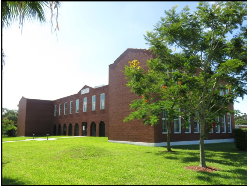
Photo 4.12. Jordan Park Elementary School (8PI06901) at 2390 9th Ave. S., facing southeast.
