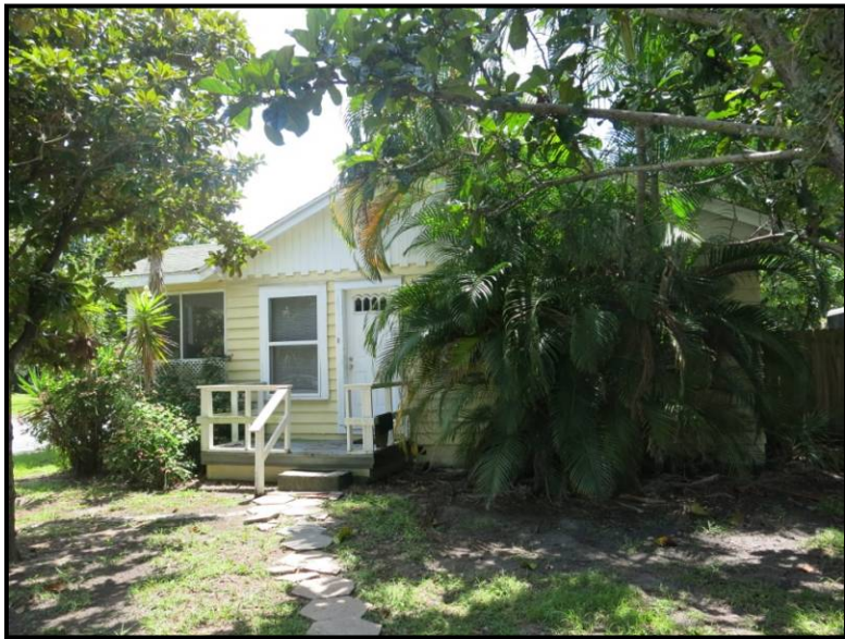
Photo 4.10. The duplex at 430 20th St. N. (8PI11108), facing southeast.
