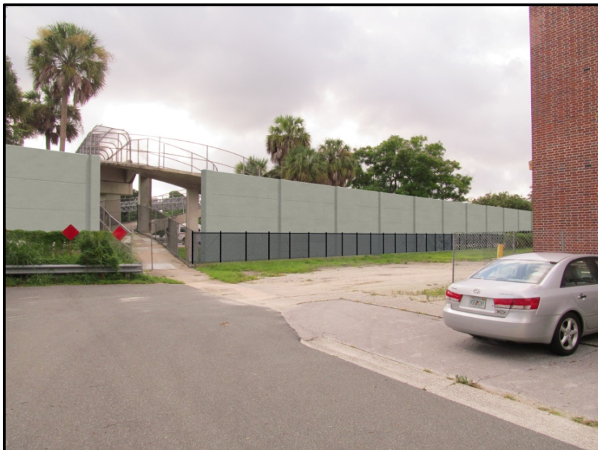
Figure 6.6. Norwood School: proposed changes in the view shed along 27th Avenue North with the installation of recommended noise barriers within the highway's right-of-way, looking east
