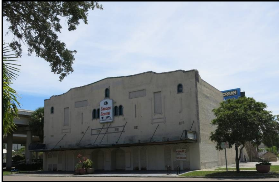
Photo 4.15. The building at 1850 Central Ave. (8PI00726), facing southeast
