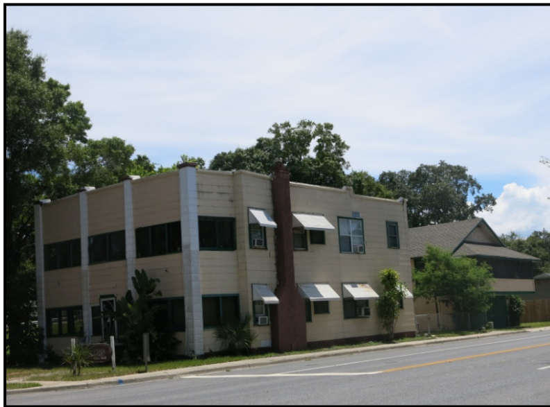
Photo 4.8. The apartment building at 1960 4th Ave. N. (8PI07970), facing southeast.
