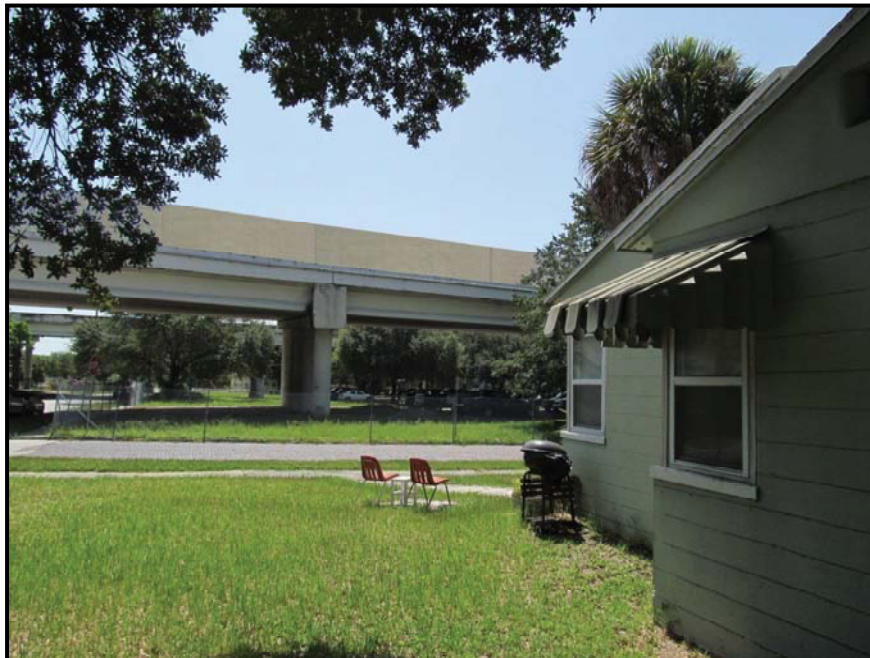
Figure 6.4 Kenwood Historic District: proposed view shed from the southwest corner of Burlington Avenue North and 19th Street North depicting a true to scale eight-foot noise barrier on the elevated highway, looking east
