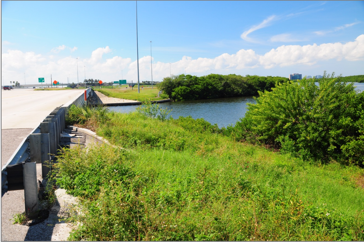
Big Island Gap Bridge – I-275 southbound (view looking south)
