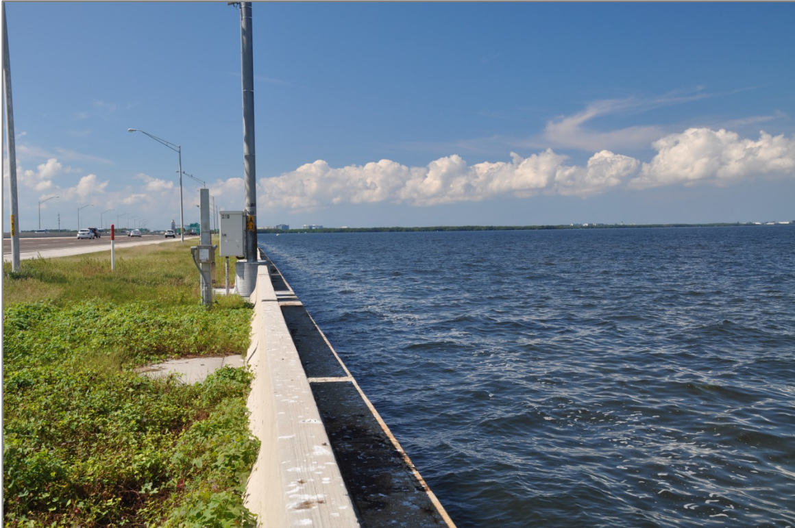
Howard Frankland Causeway – I-275 southbound (view looking east along seawall)
