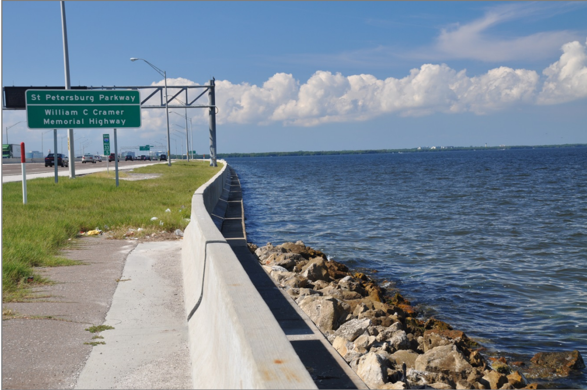
Howard Frankland Causeway – I-275 southbound (view looking west along seawall)
