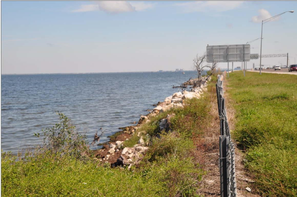
Howard Frankland Causeway – I-275 southbound (view looking east)
