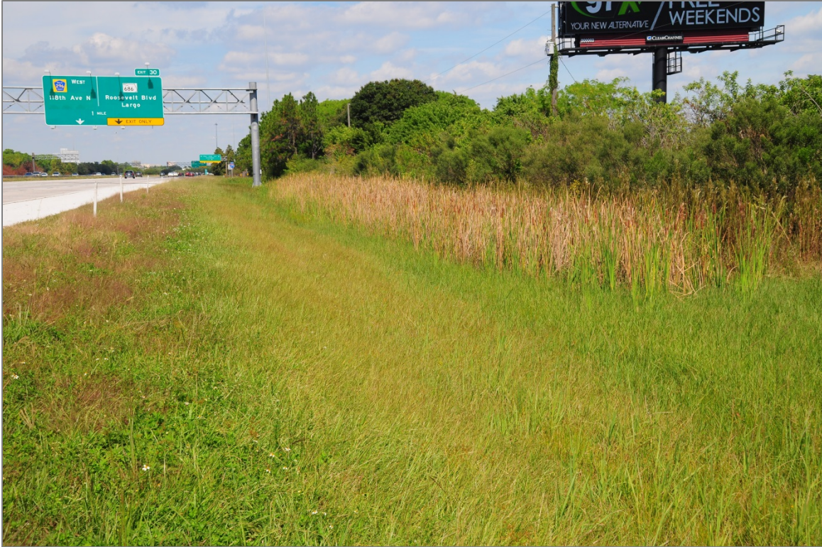
I-275 northbound south of Roosevelt Blvd. (view looking north) – Surface Water
