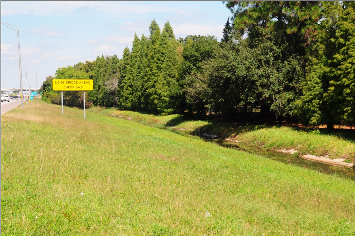
I-275 northbound south of Gandy Blvd. (view looking north) – Surface Water
