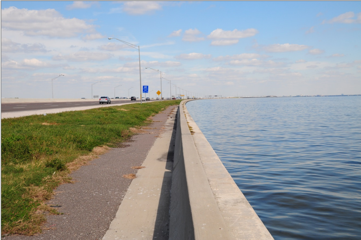
I-275 northbound (view looking northeast) – Howard Frankland Causeway
