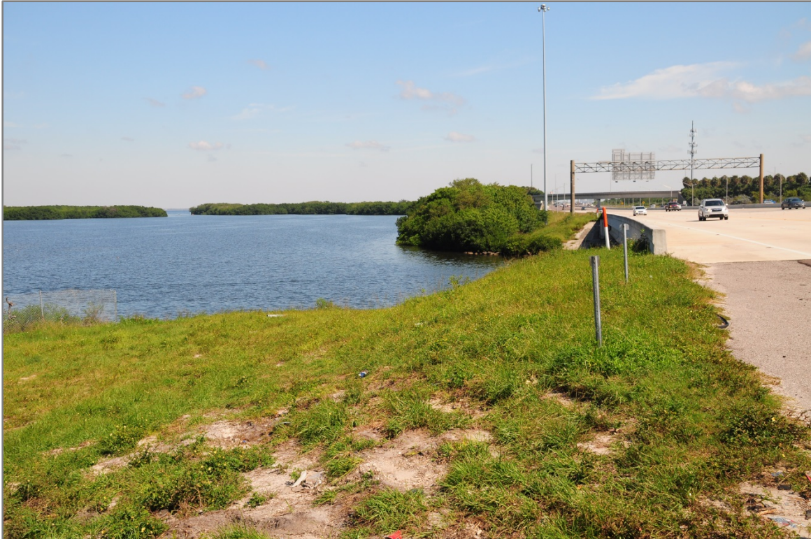
Big Island Gap Bridge – I-275 southbound (view looking north)
