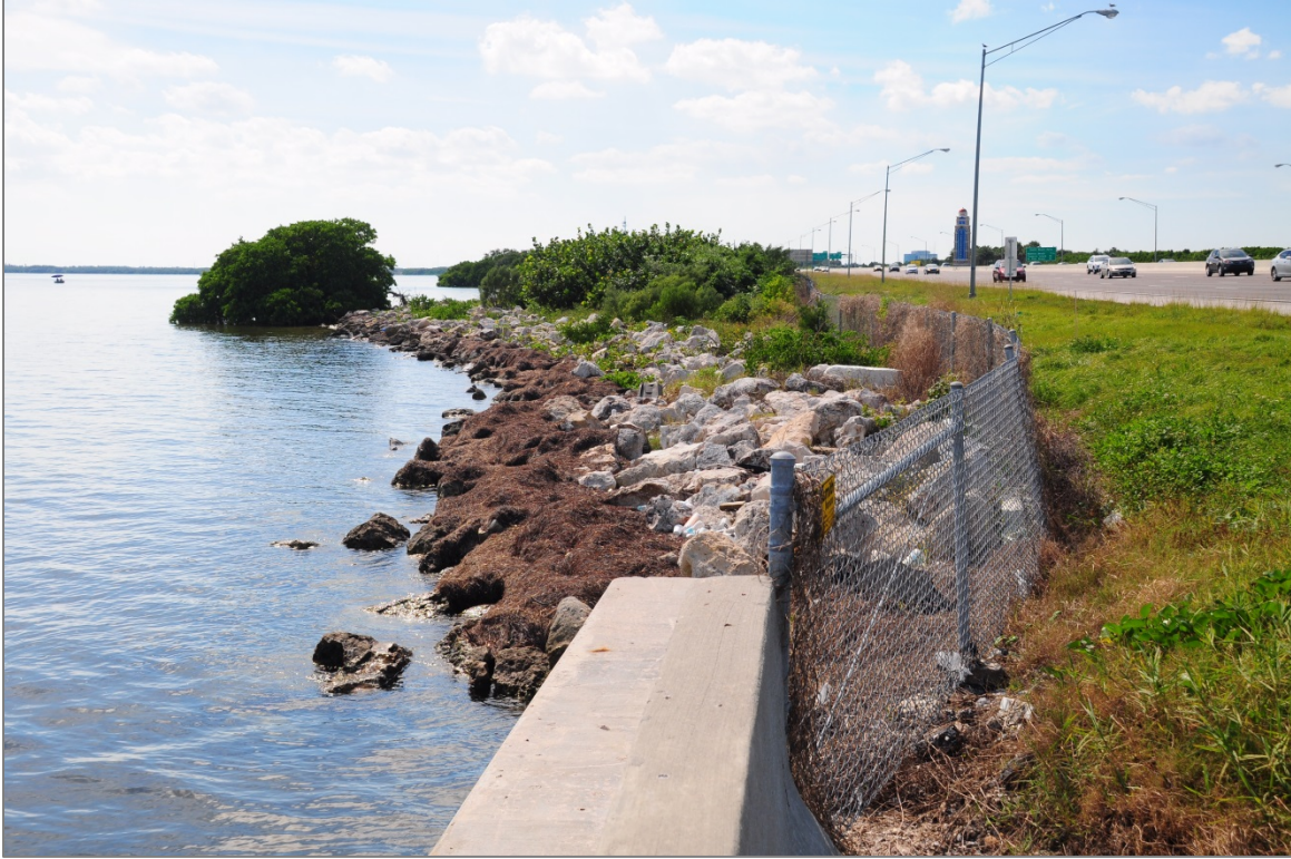
I-275 northbound (view looking southwest) – Howard Frankland Causeway
