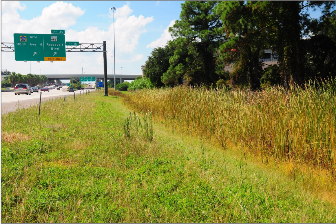
I-275 southbound (view looking south near Roosevelt Blvd.) - Surface Water Impact Area
