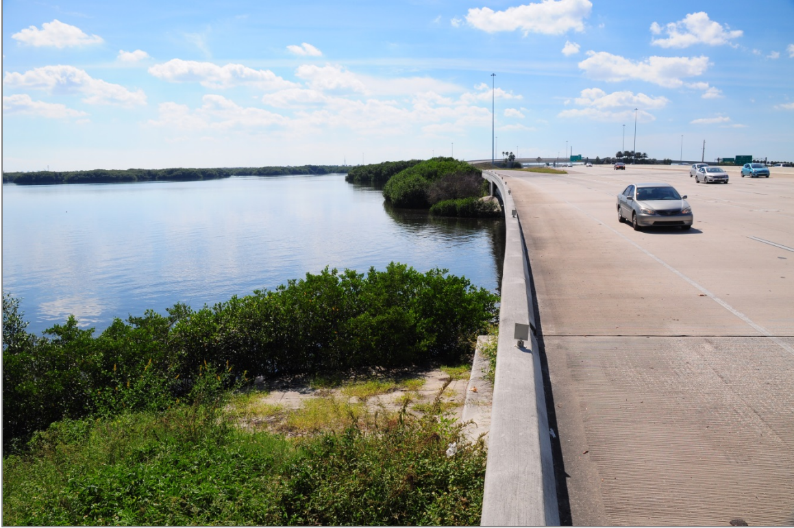
Big Island Gap Bridge – I-275 northbound (view looking south)
