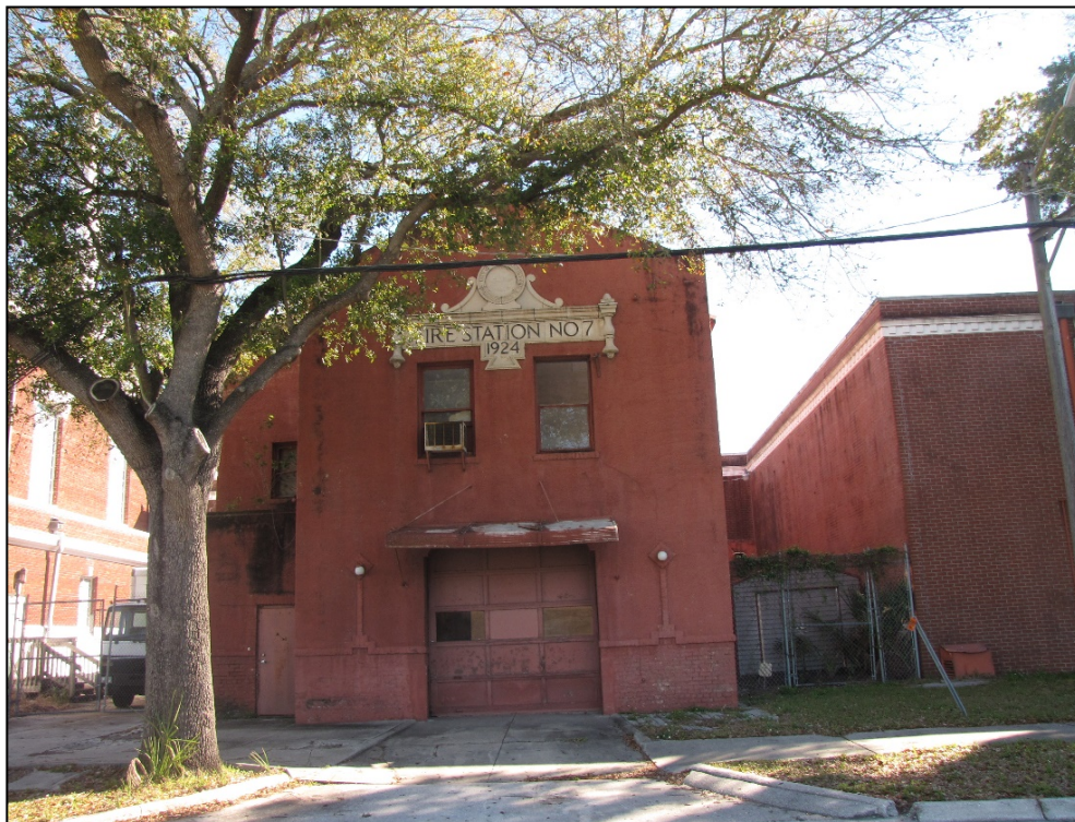
Figure 30: The West Façade of the City Fire Department Engine Company No. 7/5315 N Taliaferro Ave (8H12472), facing East
