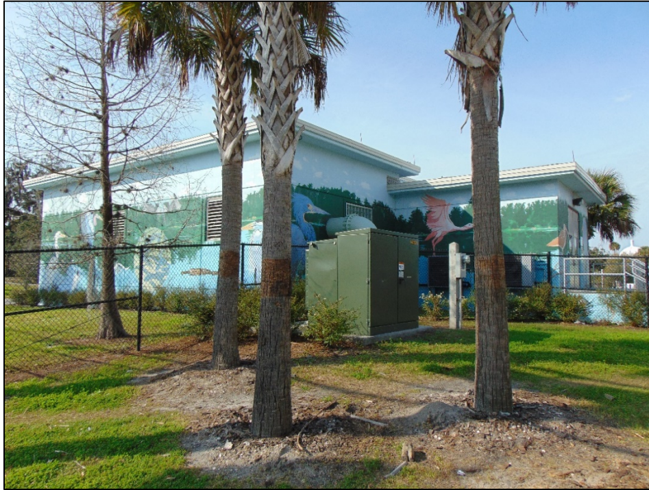
Figure 20: The Contributing circa-1953 Utility Building, facing Southwest
