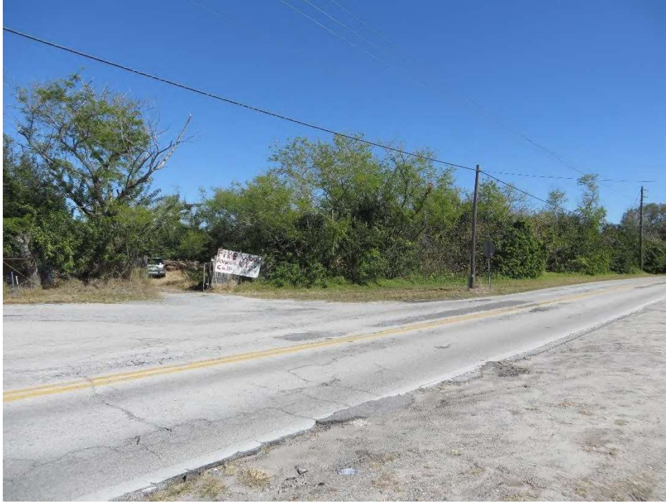
Figure 7: Project Setting for Proposed SMF 15B, Looking Northeast Toward Parcel from Sinclair Hills Road (Note: Heavy vegetation surrounding the parcel)
