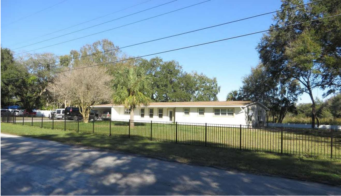
Figure 13: 148 April Lane, Looking Northwest
