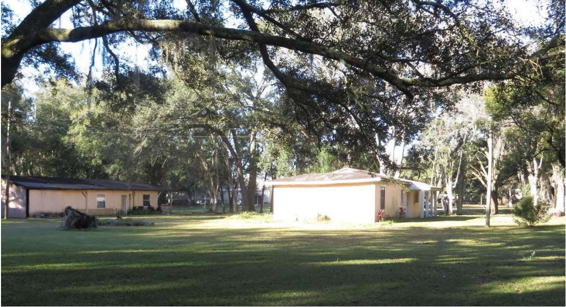
Figure 11: 131 April Lane, Looking Southwest
