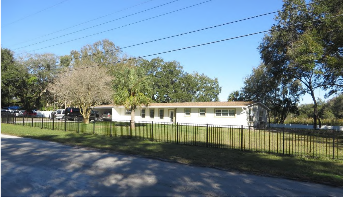
Figure 13: 148 April Lane, Looking Northwest
