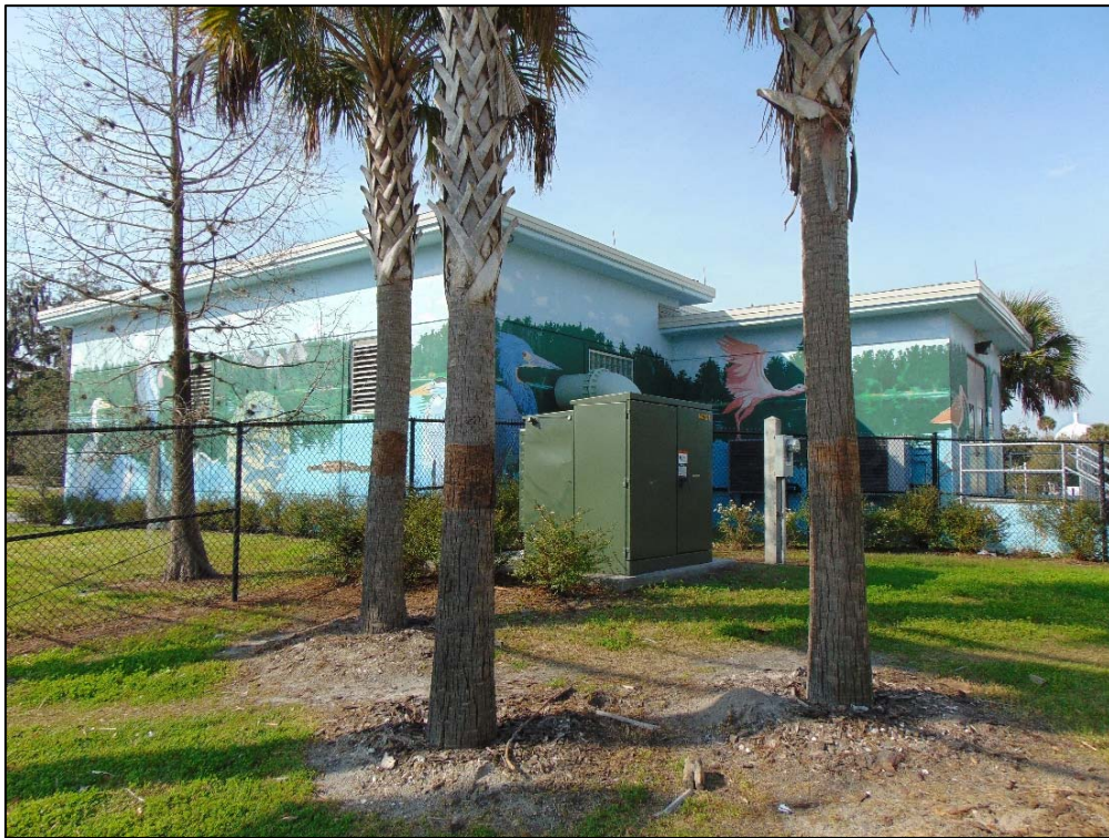
Figure 76: The Contributing circa-1953 Utility Building, facing Southwest
