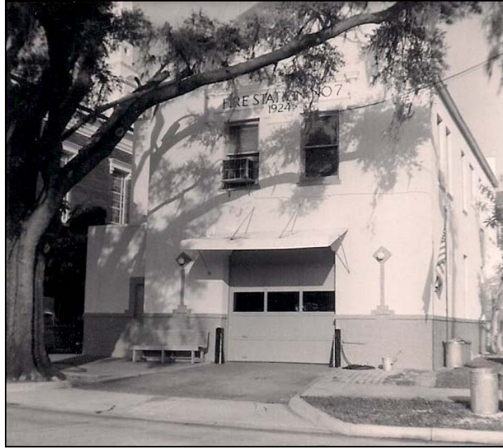
Figure 128: A circa-1971 Photograph of City Fire Department Engine Company No. 7/5315 N Taliaferro Avenue
