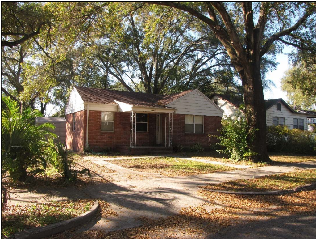
Figure 149: 5806 Osceola Place (8HI12504), c. 1950, facing Northwest
