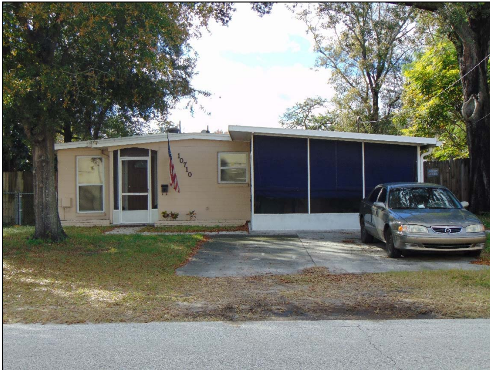
Figure 40: Example of an altered residence at 10710 N Central Avenue (8HI12815) within the APE in the East Forest Hills Neighborhood, facing West
