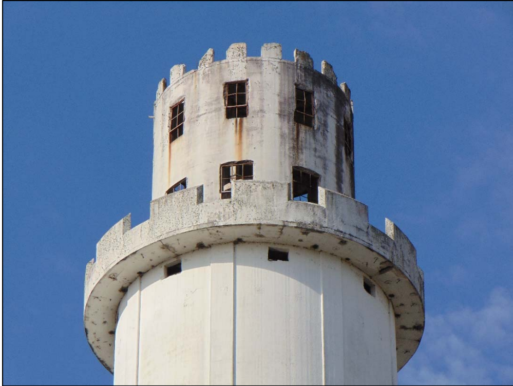
Figure 60: The Embattlements and Crenellated Parapet Walls at the Top of the Tower Holding Tank, facing Southwest
