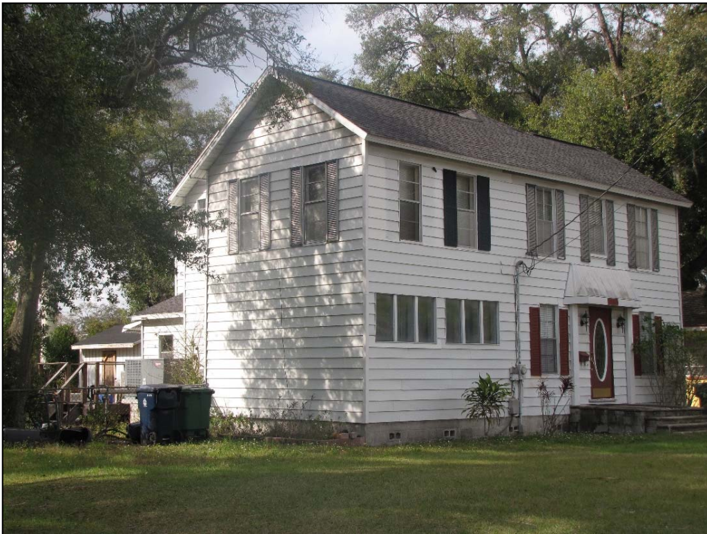
Figure 161: 6706 N Harer Street (8H112590), c. 1928, facing Northwest
