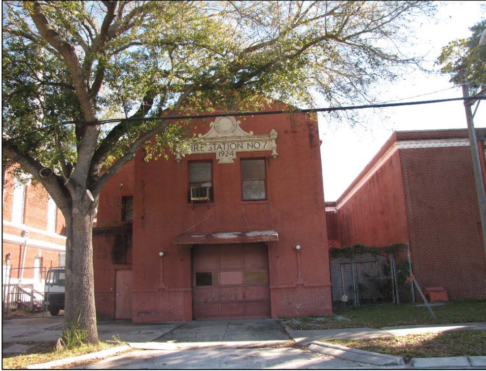
Figure 121: The West Façade of the City Fire Department Engine Company No. 7/5315 N Taliaferro Ave (8HI12472), facing East
