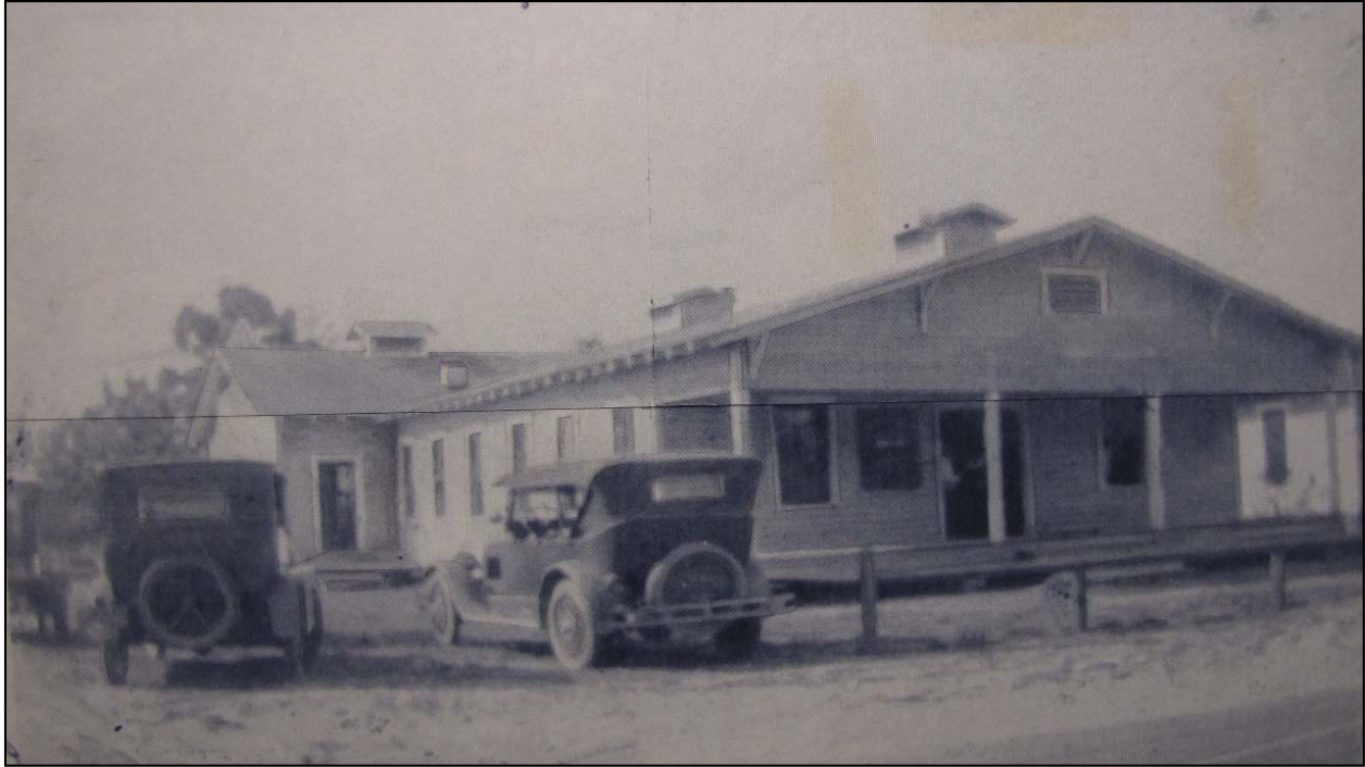
Figure 120: A Photograph of the Original Building Utilized by the Seminole Heights Baptist Church, taken circa-1922
