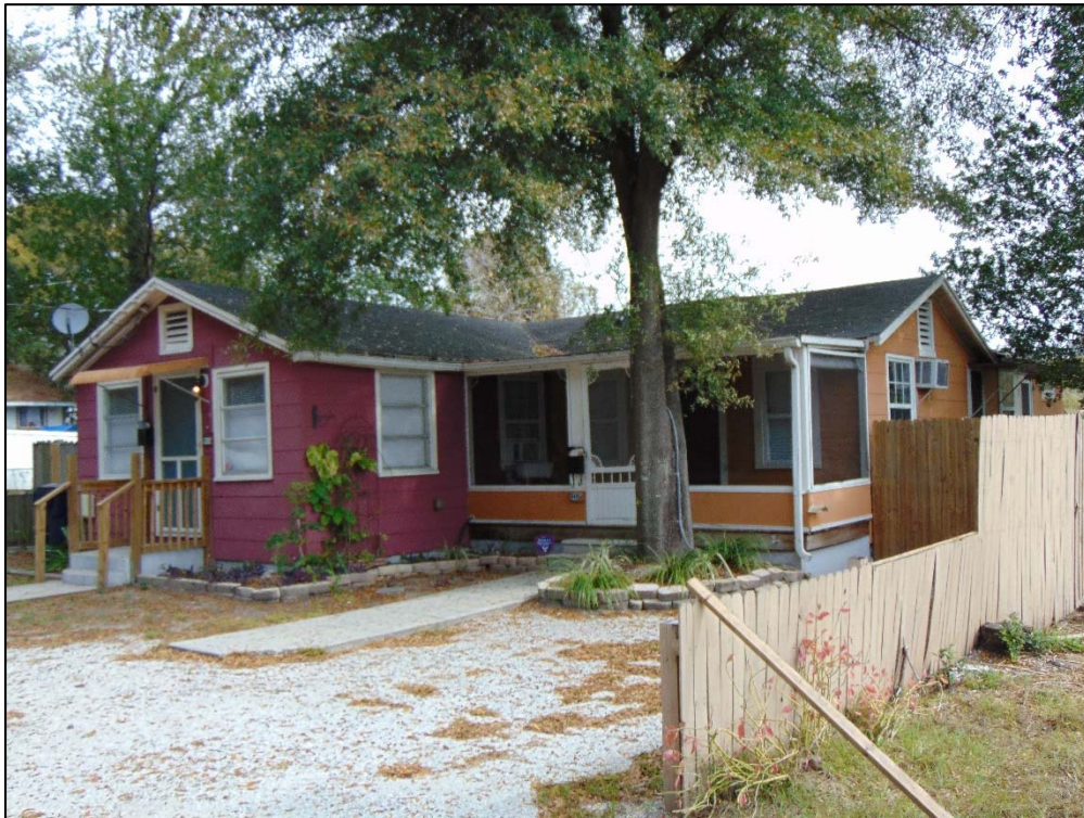
Figure 32: Example of an altered residence at 8415 N Seminole Avenue (8HI12723) within the APE in the Sulphur Springs Neighborhood, facing Northeast
