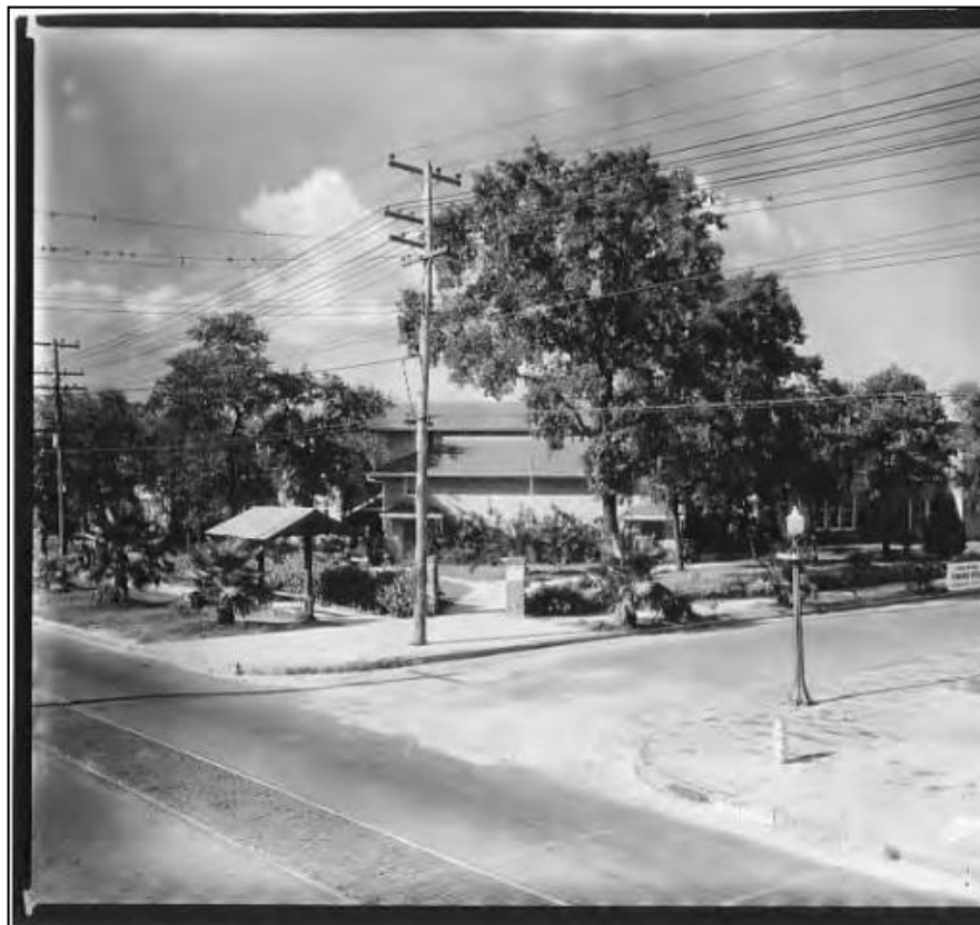
Figure 134: A Historic circa-1936 Photograph of Seminole Heights Elementary School/6201 N Central Avenue
