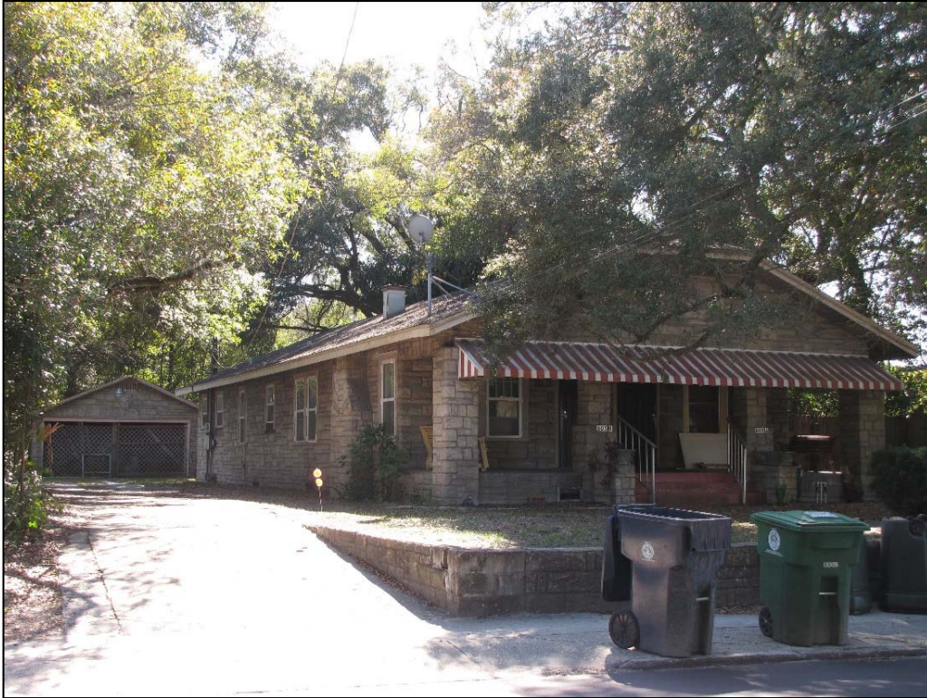
Figure 154: 805 E Hanna Avenue (8HI12535), c. 1925, facing Southwest
