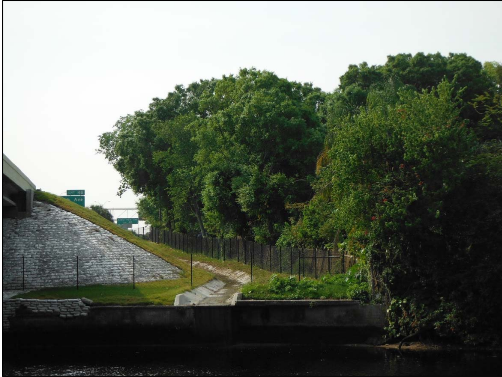
Bridge Berm and Drainage Features adjacent to the Hillsborough River, facing South
