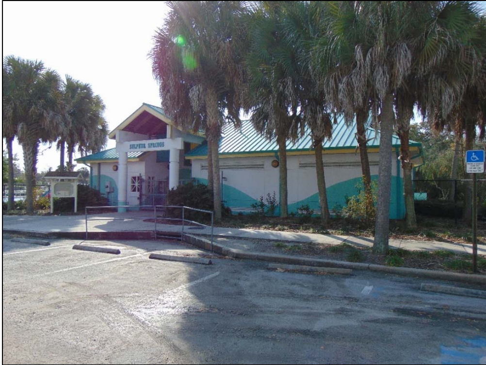
Figure 81: The Non-contributing circa-2001 Sulphur Springs Park Main Building, facing southeast
