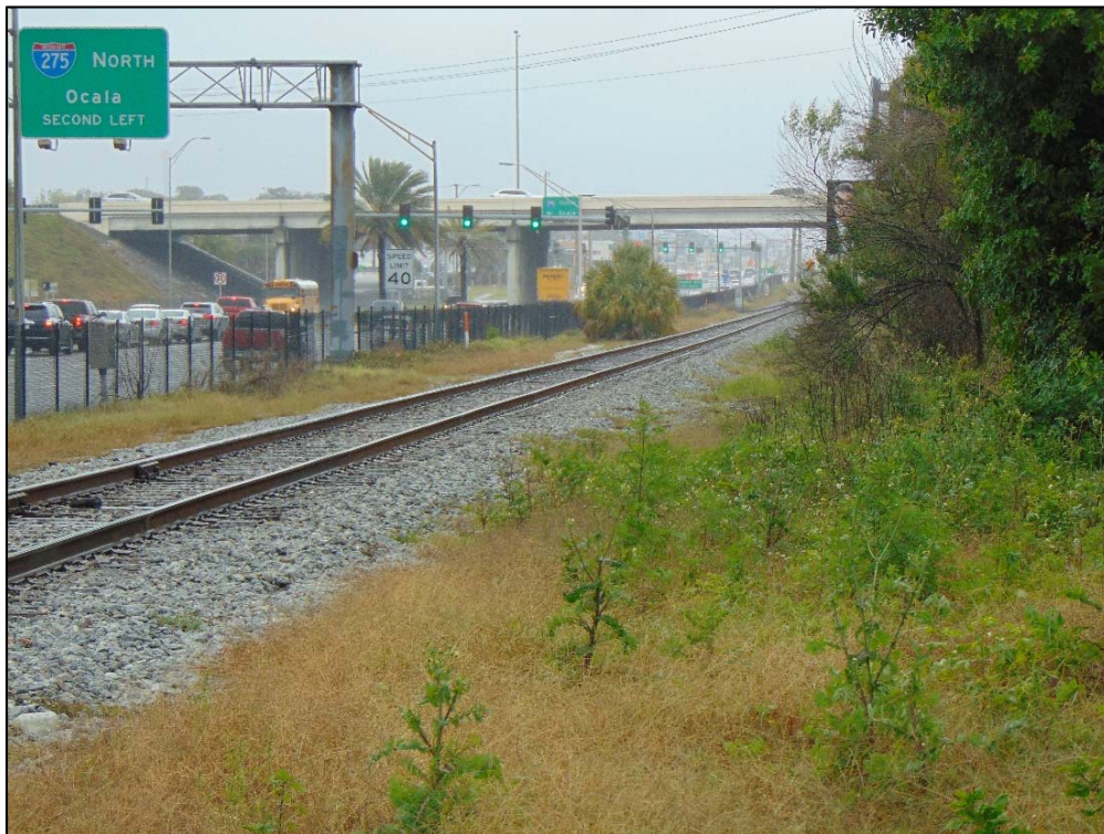
Figure 104: Tampa and Gulf Coast Railroad/CSX Railroad within the APE, looking towards I-275, facing northeast
