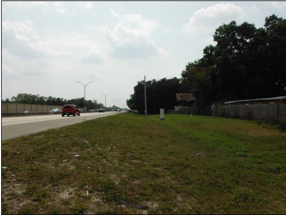
Road Berm and Buried Utilities near April Lane, facing South
