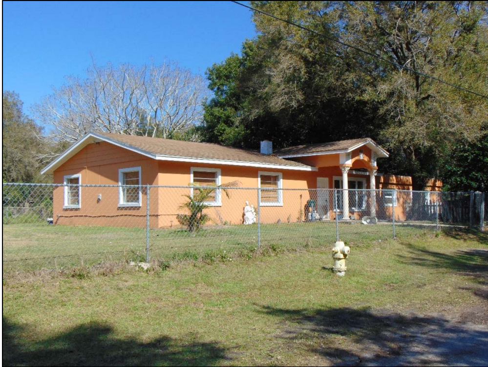
Figure 49: Example of an altered residence at 14901 Laurie Lane, just outside the APE in Lake Magdalene, facing Northeast
