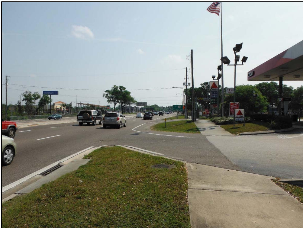
Buried Utilities along Bearss Avenue, facing East
