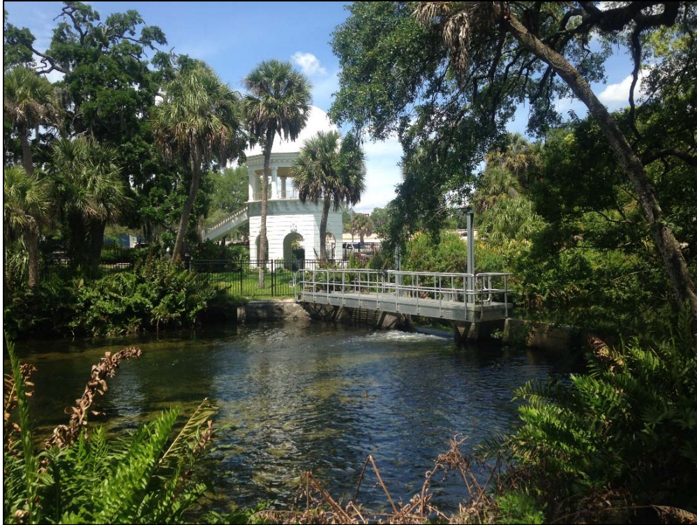
Figure 83: The Non-contributing circa-2000s Steel Bridge which Rests on the Western Lock of the Meandering Spring Pool, facing Northeast
