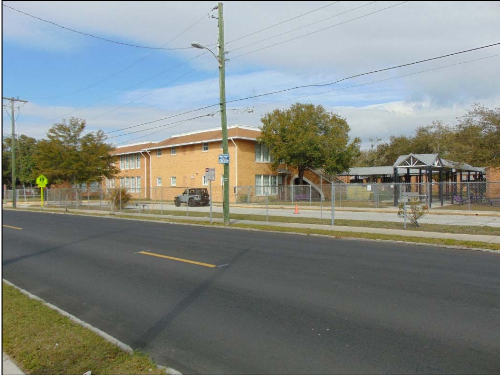
Figure 131: South Wing of Seminole Heights Elementary School/6201 N Central Avenue (8HI12539), from E Hanna Avenue, facing Northwest
