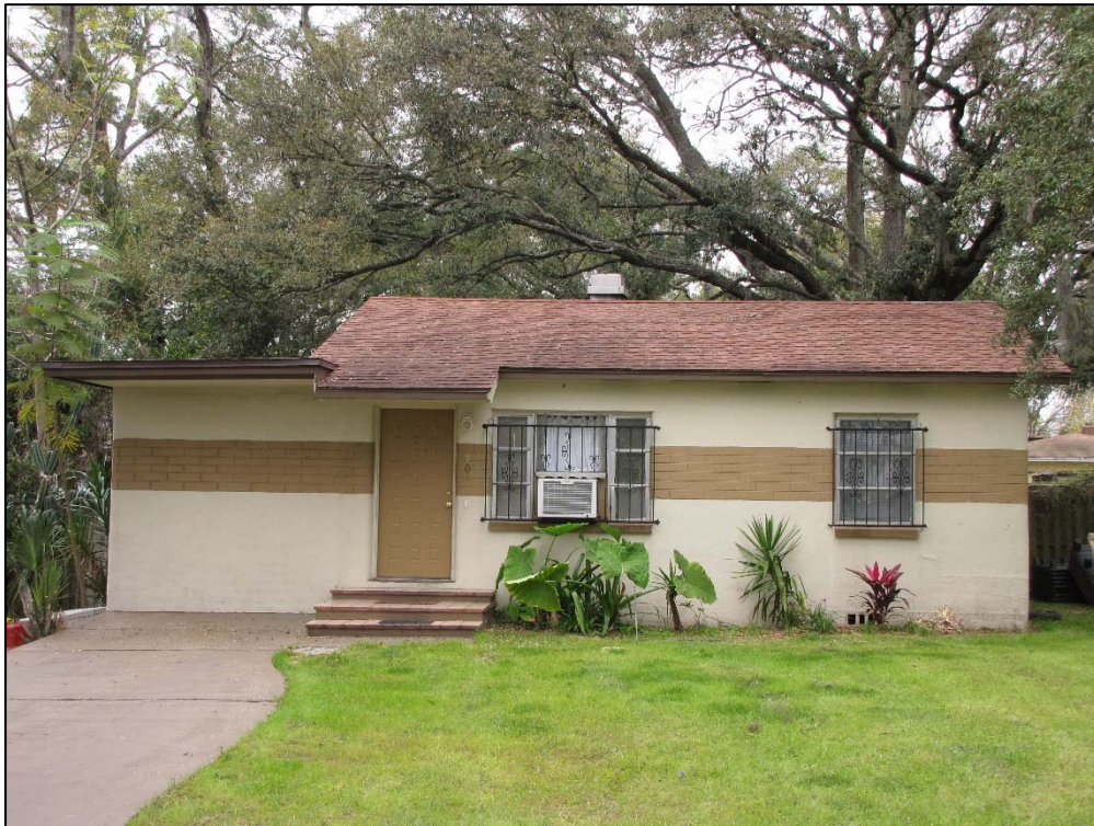
Figure 43: Example of an altered residence at 704 E Richmere Street, just outside the APE in North Tampa, facing North
