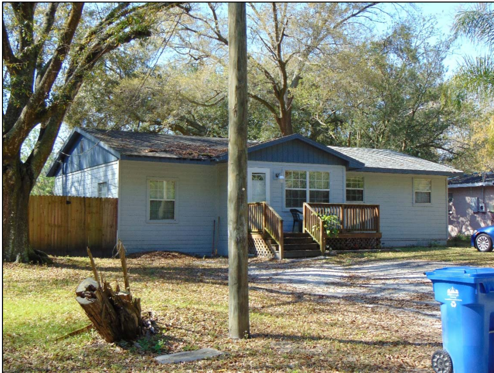
Figure 50: Example of an altered residence at 14916 Laurie Lane (8HI12913) within the APE in Lake Magdalene, facing Northwest
