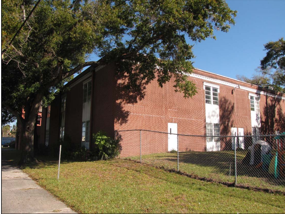
Figure 119: The Mid-1970s Flat Roof Addition of the Seminole Heights Baptist Church/801 E Hillsborough Avenue (8HI12470), facing Northeast
