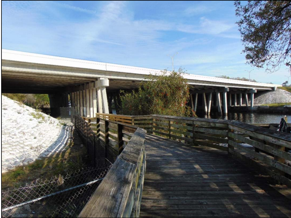
Figure 85: The Non-contributing and Non-historic I-275 Overpass Pathway and Bridge, facing southeast
