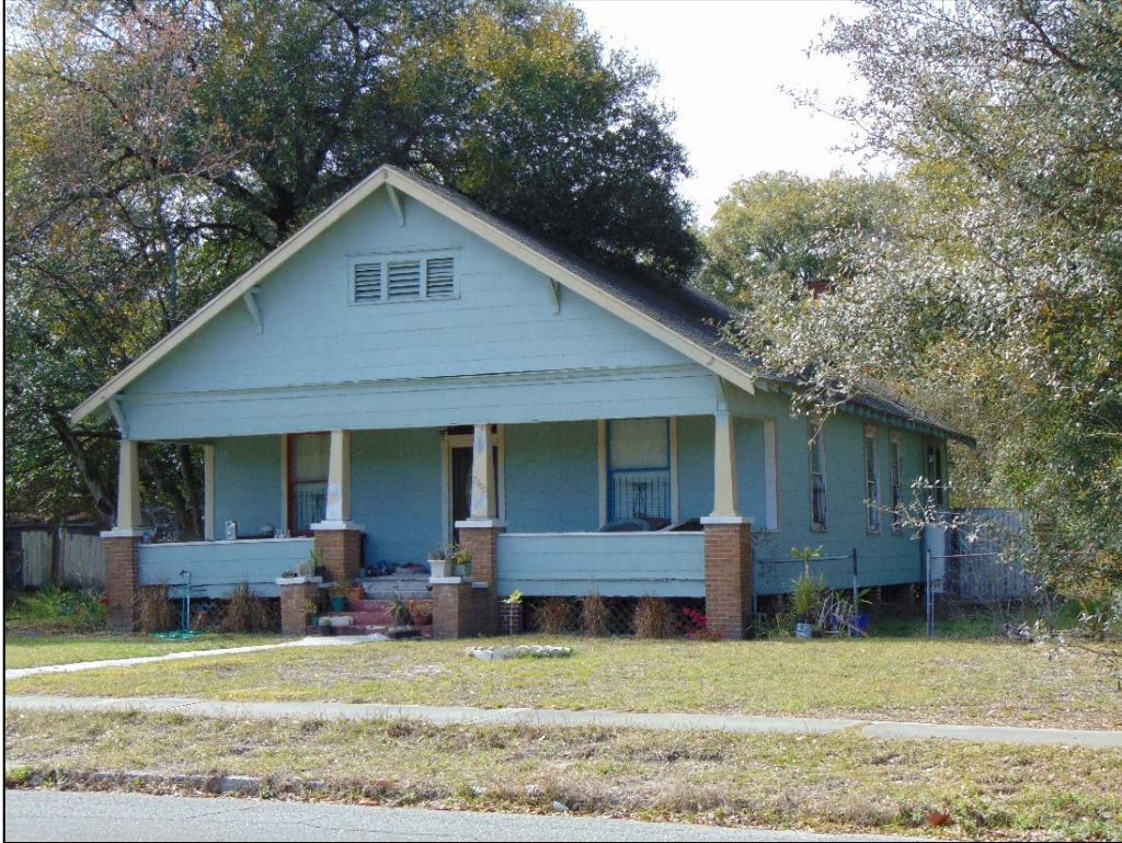
Figure 168: 7300 N Central Avenue (8HI12670), c. 1918, facing Southwest
