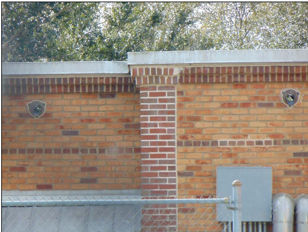
Figure 132: Polychromy and Pilasters of Seminole Heights Elementary School/6201 N Central Avenue (8HI12539), facing South
