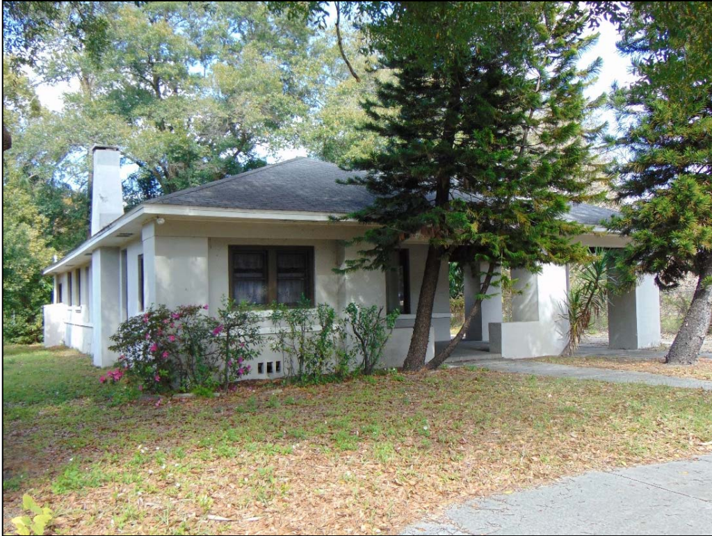
Figure 144: 510 E Frierson Avenue (8H112460), c. 1918, facing Northeast
