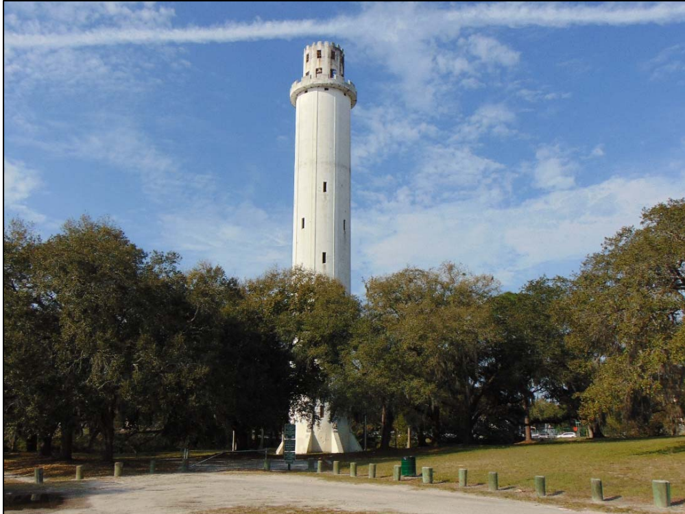
Figure 58: The Contributing Gothic Inspired Water Tower within the Sulphur Springs Park Resource Group (8H1609), facing Southwest
