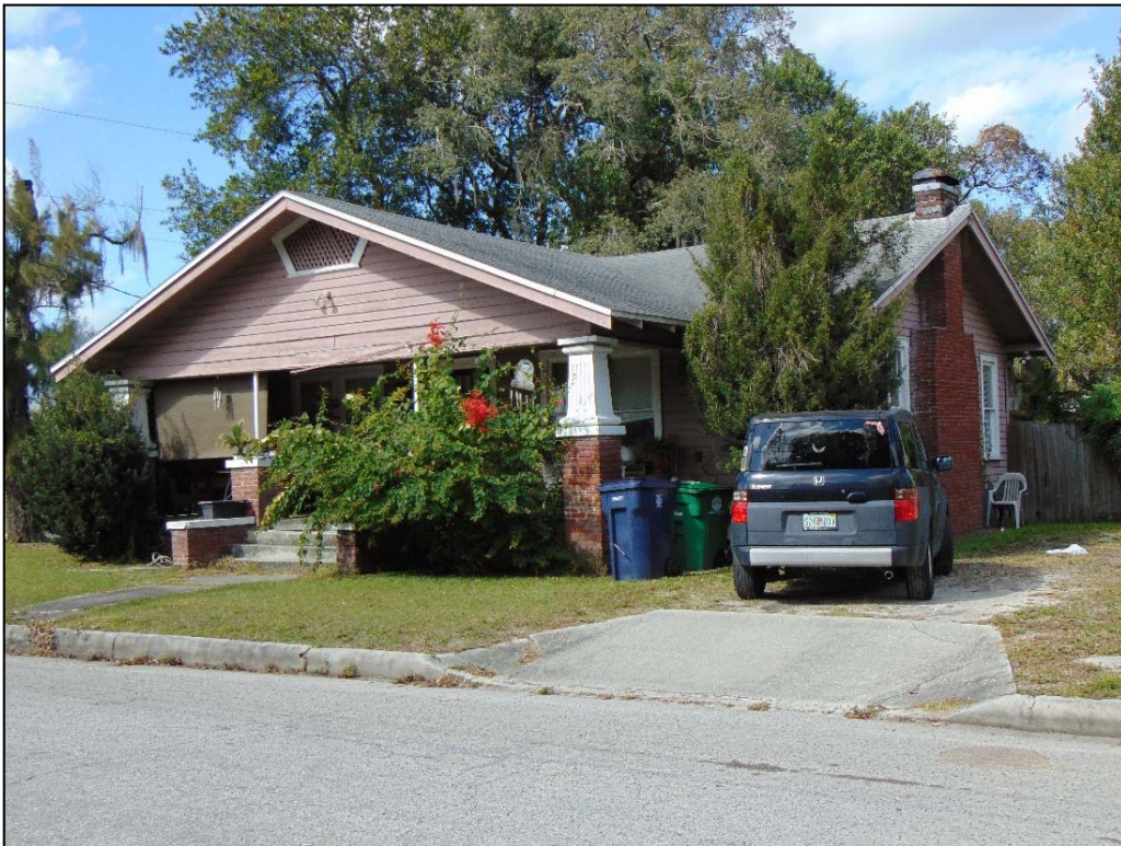
Figure 143: 800 E New Orleans Avenue (8HI12402), c. 1925, facing Northwest
