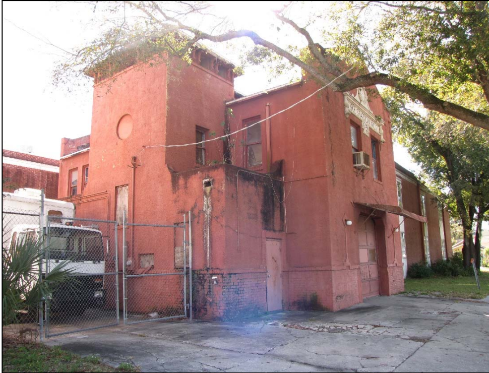
Figure 122: The North and West Elevations of City Fire Department Engine Company No. 7/5315 N Taliaferro Avenue (8H112472), facing Southeast
