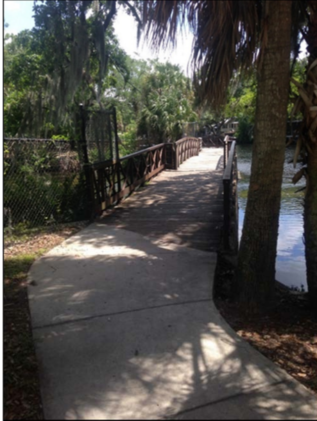
Figure 68: The Contributing circa-1950s Wooden Bridge, facing Southeast
