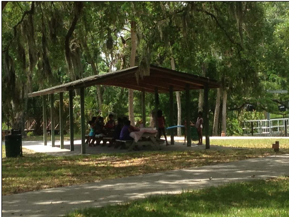
Figure 69: The Contributing circa-1953 Pavilion, facing Southeast
