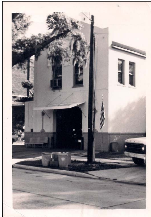
Figure 127: A Photograph of City Fire Department Engine Company No. 7/5315 N Taliaferro Avenue, taken prior to 1971
