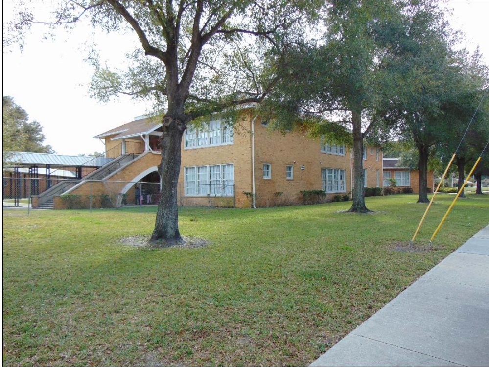
Figure 135: The Concrete Exterior Stairs of the North Wing of Seminole Heights Elementary School/6201 N Central Avenue (8HI12539), facing Southwest
