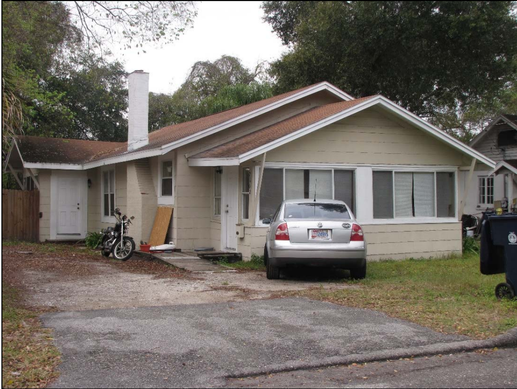
Figure 166: 7102 N Taliaferro Avenue (8HI12641), c. 1946, facing Northwest
