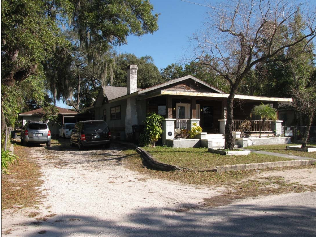
Figure 156: 6305 N King Street (8HI12541), c. 1927, facing Southeast
