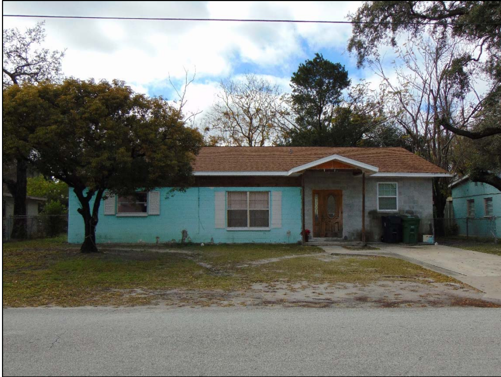
Figure 39: Example of an altered residence at 10704 N Central Avenue (8HI12812) within the APE in the East Forest Hills Neighborhood, facing West
