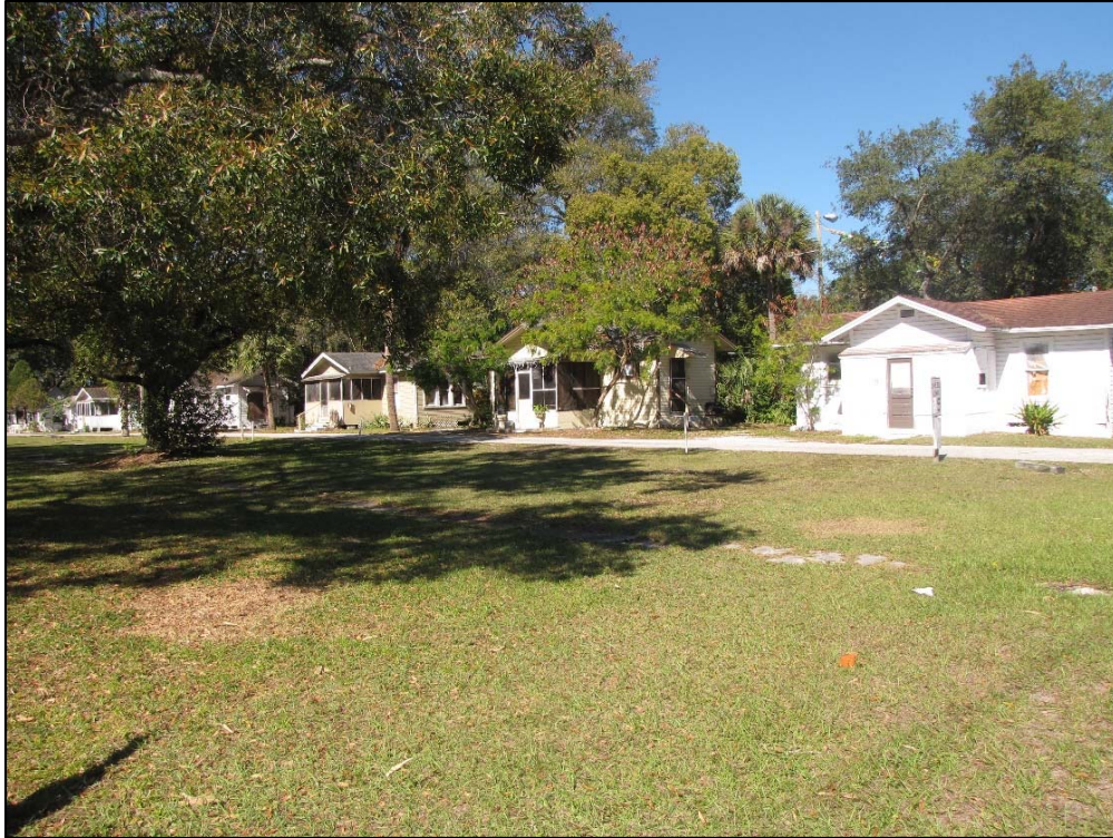
Figure 98: Harding's Court/5912 N Nebraska Avenue (8HI6132), from N Nebraska Avenue, facing northwest
