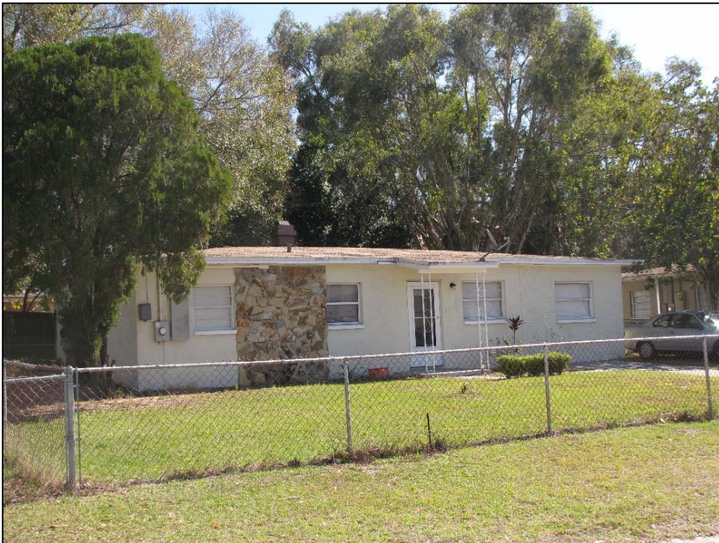
Figure 177: 10919 N Florence Avenue (8H112826), c. 1959, facing Southeast
