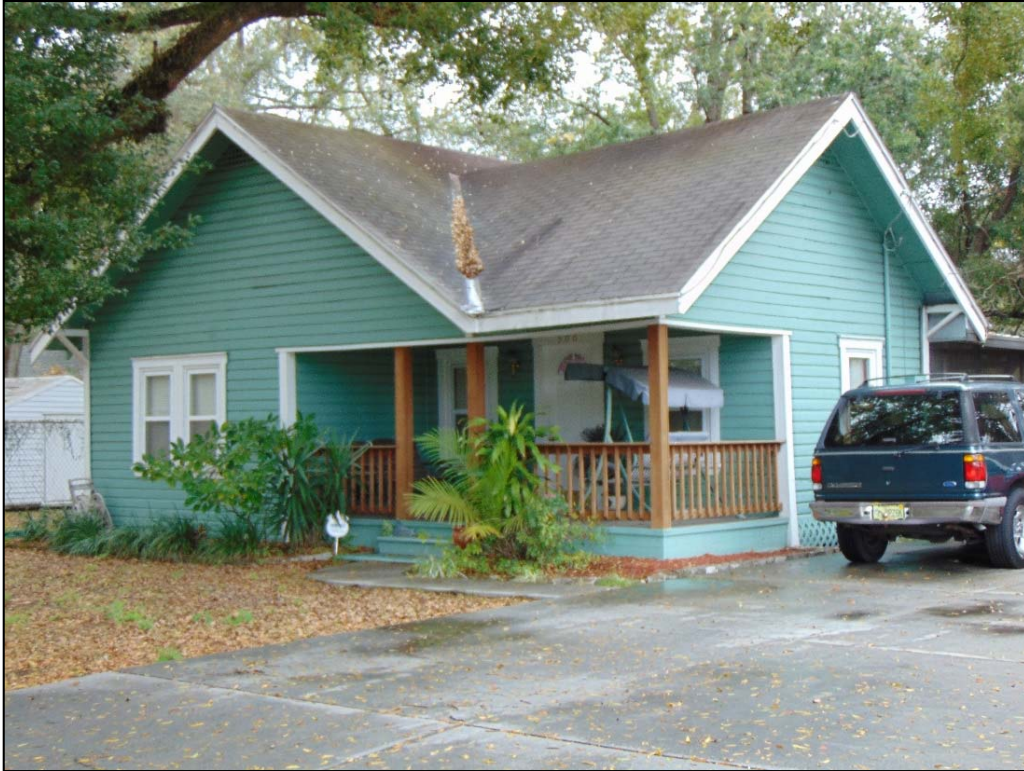
Figure 164: 506 E Elm Street (8HI12613), c. 1928, facing Northwest
