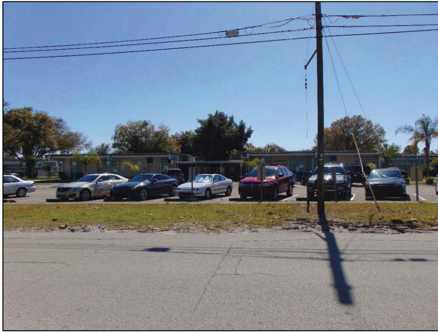
Figure 4: The circa-1962 Office Building Fronting E 124 th Avenue, facing South
