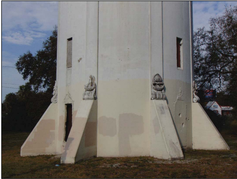
Figure 3: The Concrete Buttresses of the Water Tower with Foliated Shell Motif Embellishment, facing Northwest
