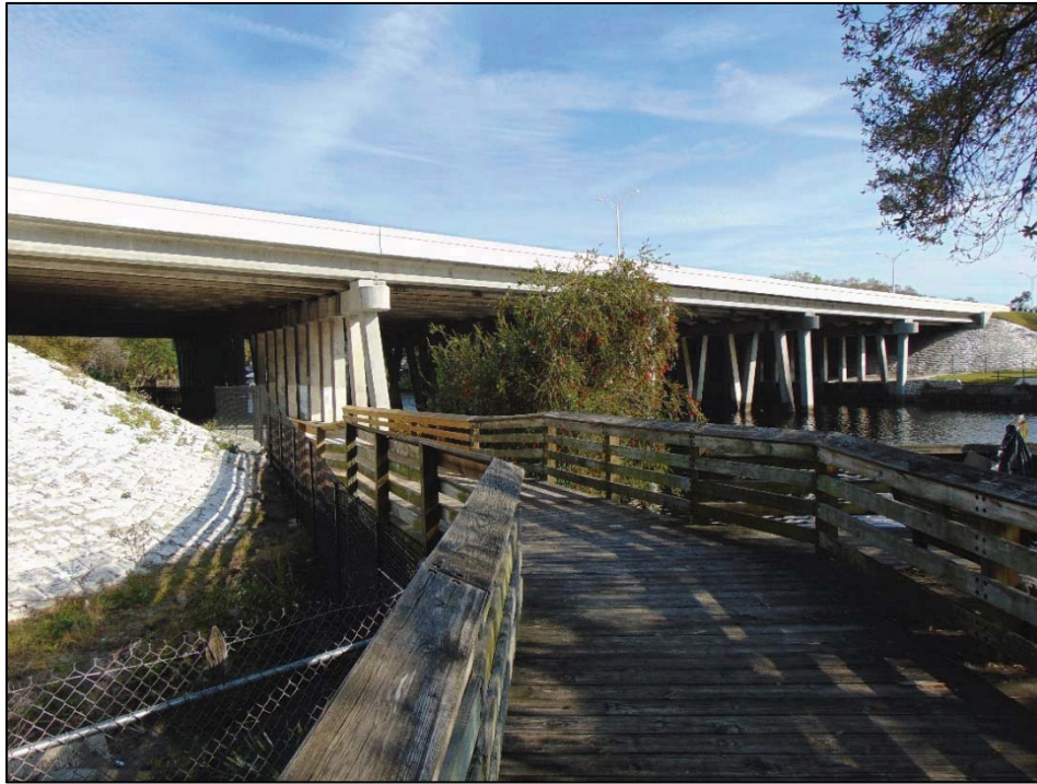
Figure 29: The Non-contributing and Non-historic I-275 Overpass Pathway and Bridge, facing southeast
