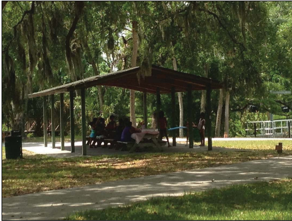
Figure 13: The Contributing circa-1953 Pavilion, facing Southeast
