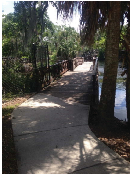
Figure 12: The Contributing circa-1950s Wooden Bridge, facing Southeast
