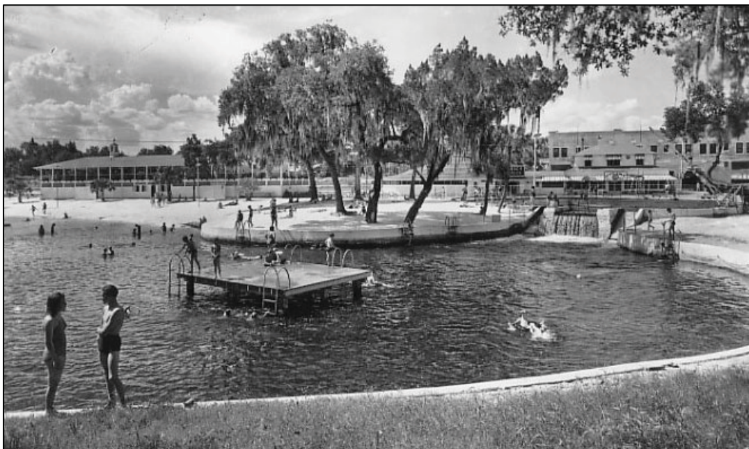
Figure 19: A Historic circa-1935 Photograph of the Contributing Meandering Sulphur Springs Pool, note the waters of the contributing circular concrete retaining wall pool flowing into the secondary "bathing pool"
