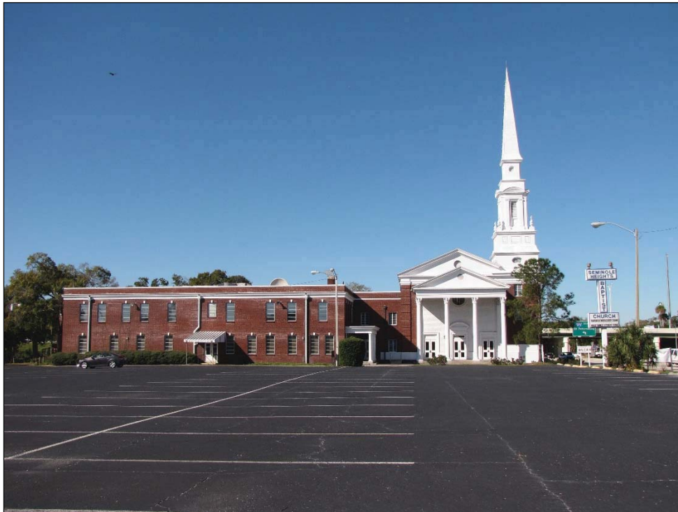
Figure 1: West Façade of Seminole Heights Baptist Church/801 E Hillsborough Avenue (8HI12470), facing West
