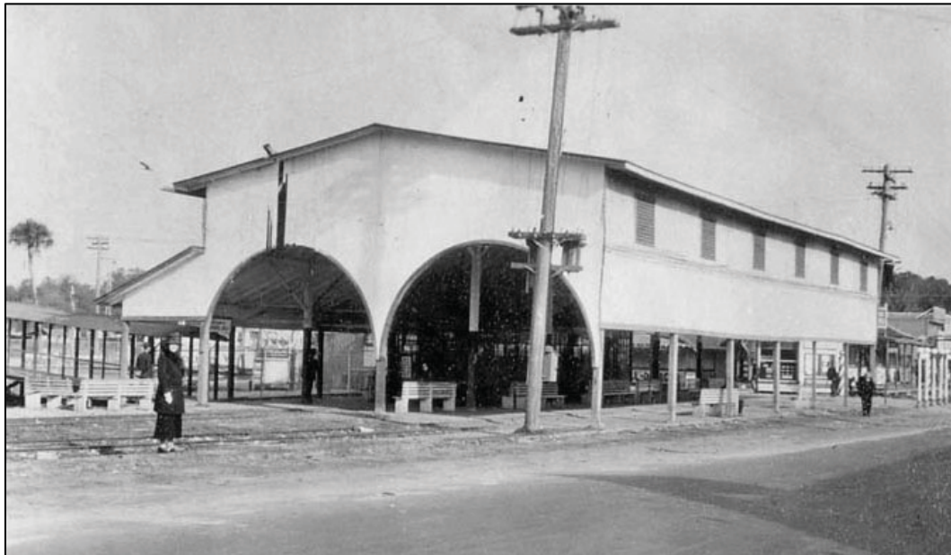
Figure 34: A 1920 Photograph of the Electric Train Shed (Courtesy of www.tampapix.com )
