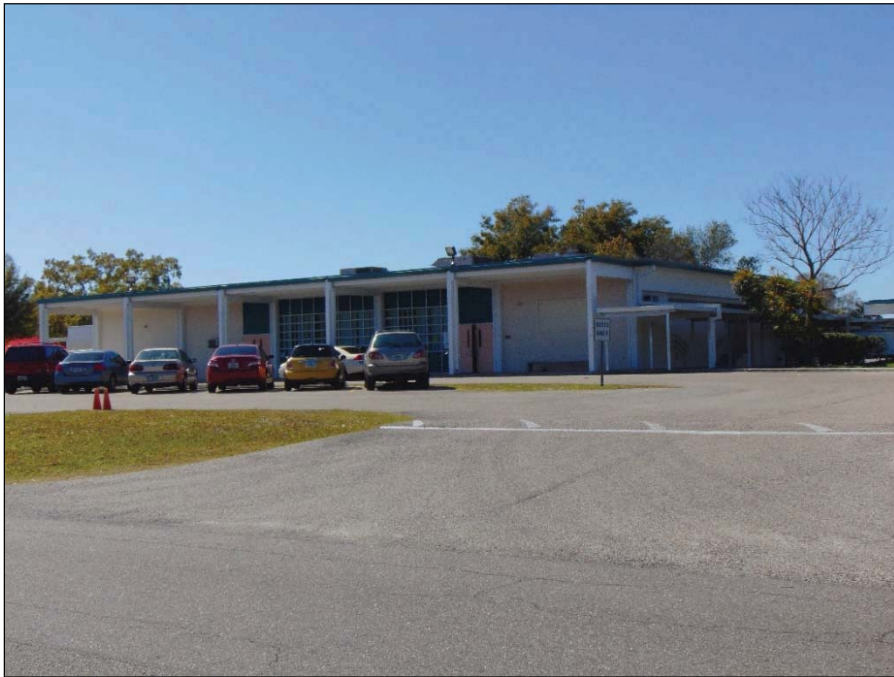
Figure 3: The East Building Within the Miles Elementary School Resource Group which is within the Current Project APE, facing Southwest
