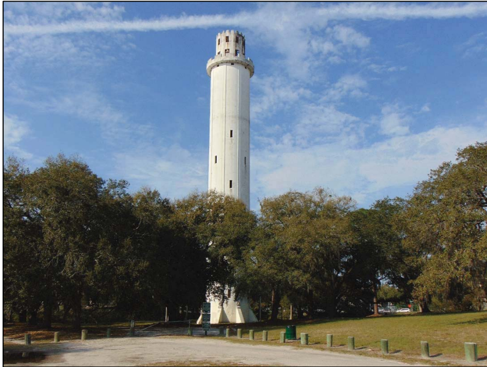
Figure 2: The Contributing Gothic Inspired Water Tower within the Sulphur Springs Park Resource Group (8HI609), facing Southwest
