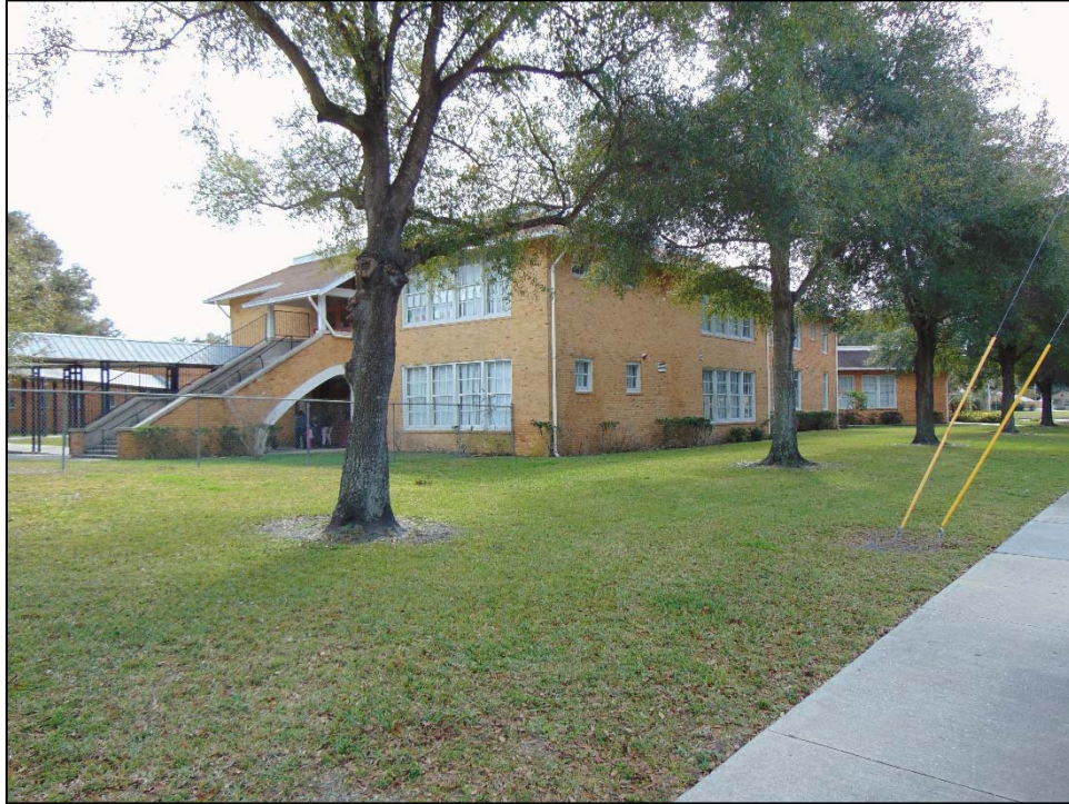
Figure 6: The Concrete Exterior Stairs of the North Wing of Seminole Heights Elementary School/6201 N Central Avenue (8HI12539), facing southwest
