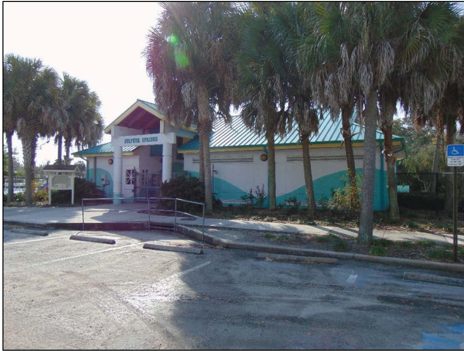
Figure 25: The Non-contributing circa-2001 Sulphur Springs Park Main Building, facing southeast
