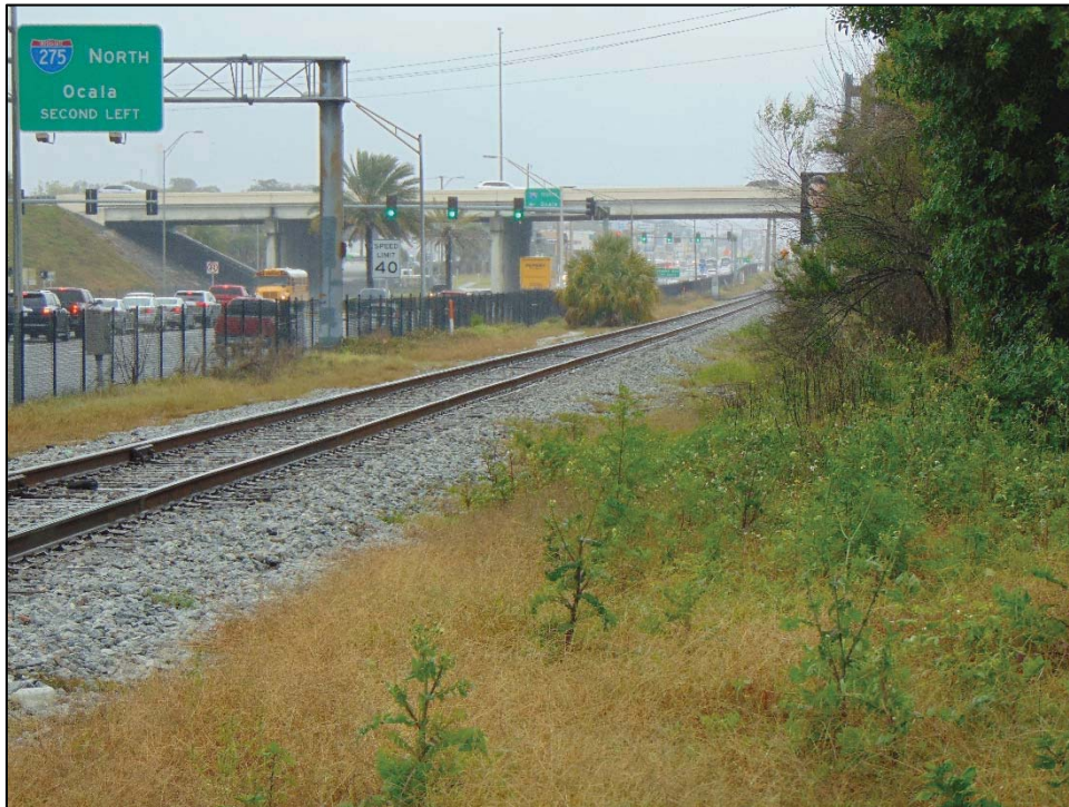
Figure 1: Tampa and Gulf Coast Railroad/CSX Railroad within the APE, looking towards I-275, facing northeast
