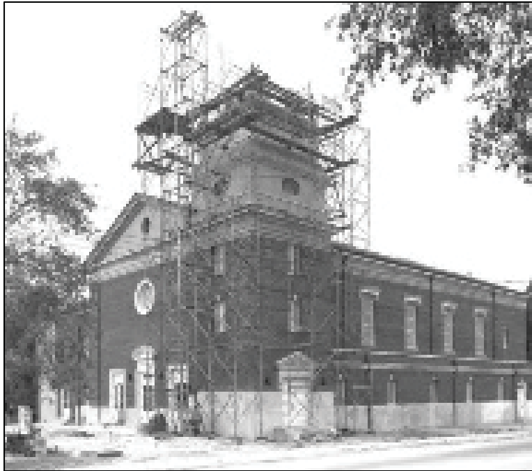
Figure 7: A 1949 Photograph of Seminole Heights Baptist Church During Construction of the Steeple (Photograph Courtesy of the Hillsborough Public Library Burgert Bros. Collection)
