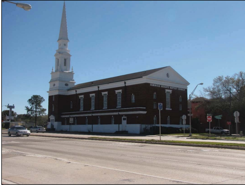
Figure 3: The Original Circa-1949 Sanctuary of the Seminole Heights Baptist Church/801 E Hillsborough Avenue (8HI12470), facing Southeast
