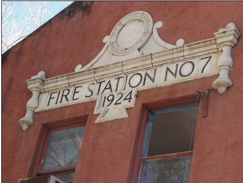
Figure 3: Historic Embossed Stucco Signage of City Fire Department Engine Company No. 7/5315 N Taliaferro Avenue (8HI12472), facing northeast
