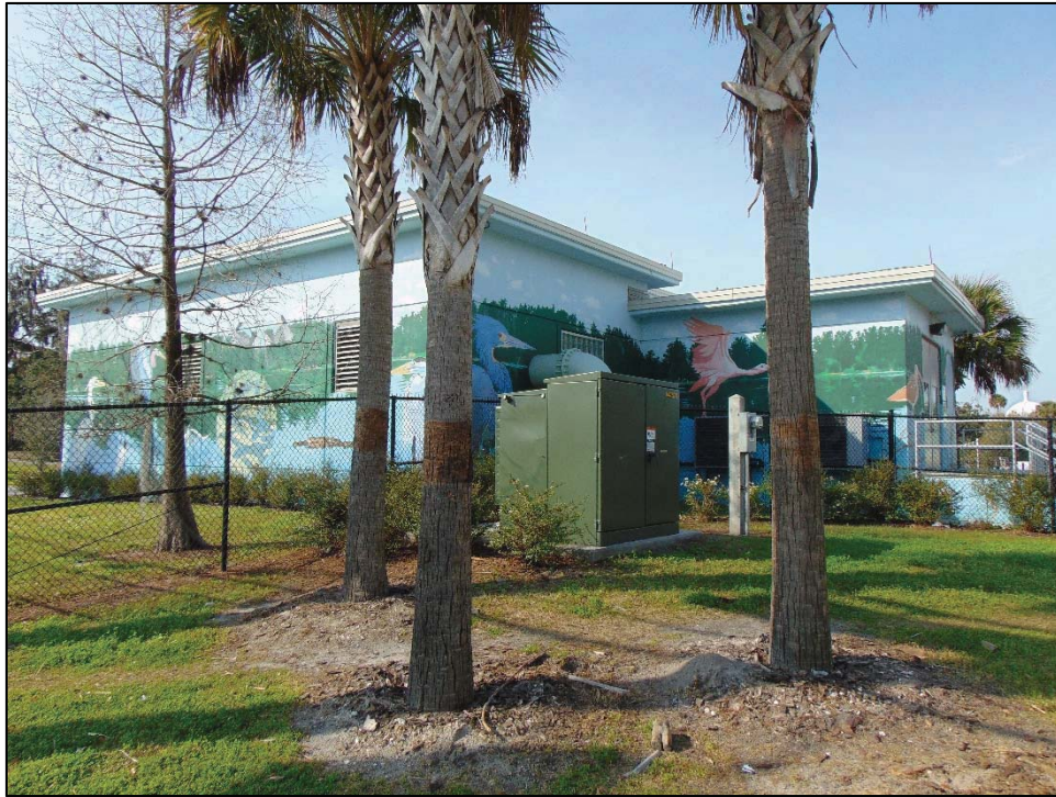
Figure 20: The Contributing circa-1953 Utility Building, facing Southwest
