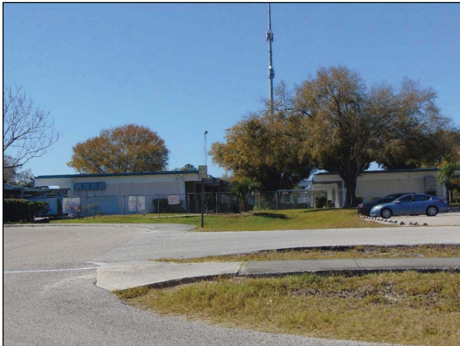
Figure 5: Circa-1962 Constructed Classroom Buildings of Miles Elementary School, facing West
