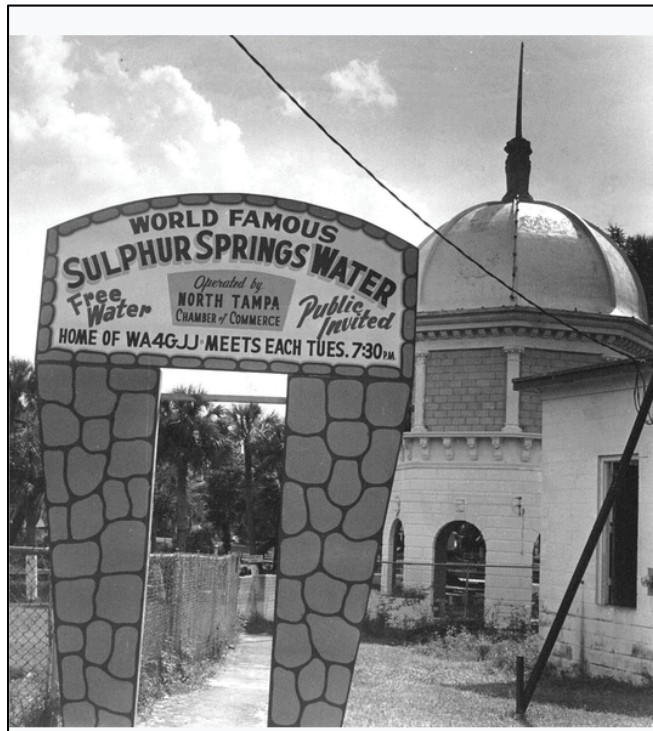
Figure 14: A 1962 Photograph of the Enclosed Gazebo (Courtesy of the Tampa Tribune)
