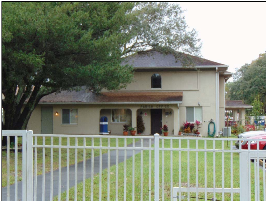
Figure 7: The Most Holy Redeemer Office/Dormitory Building, facing West
