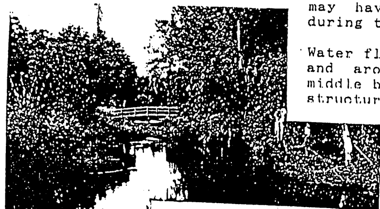
Middle drive bridge looking downstream from the southerly bridge on 9/20/88.
