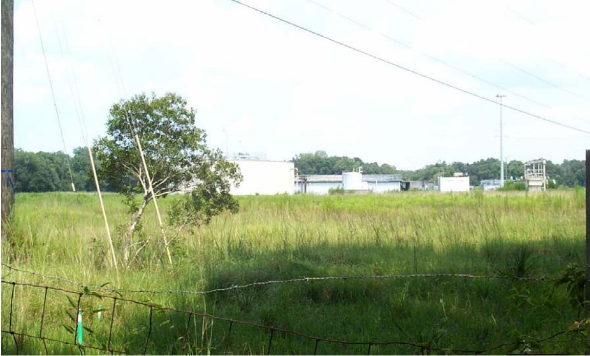
Site No. 16 – Old Wesley Chapel Waste Water Treatment Plant
