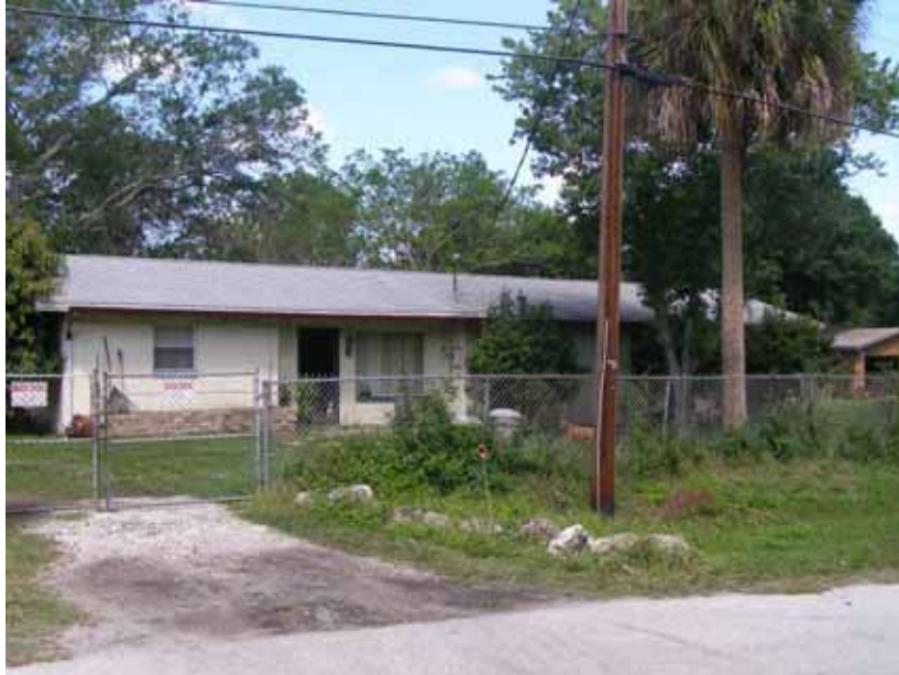
Photo 5-8: East elevation of 8007 Formby Street (8HI11302), looking west
