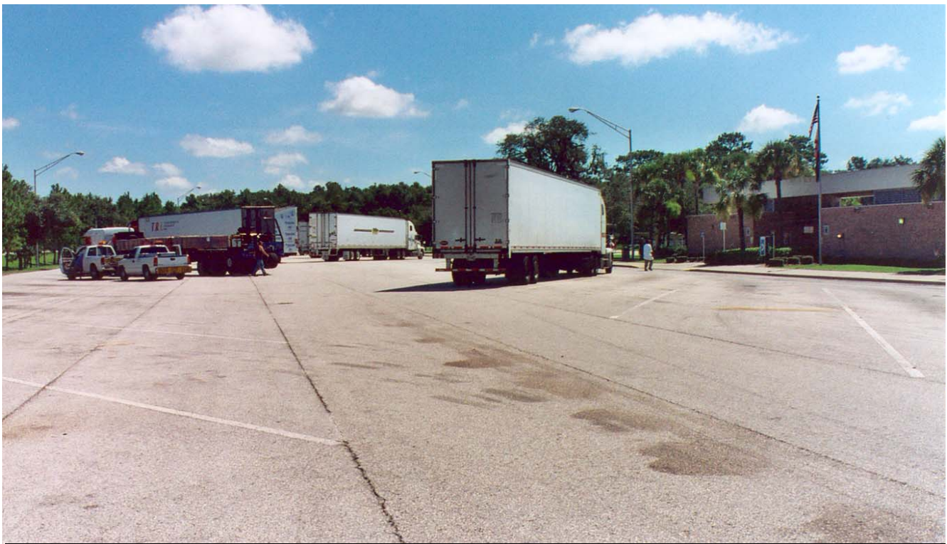
Site #8- northward view of NB I-75 rest stop showing truck area.
