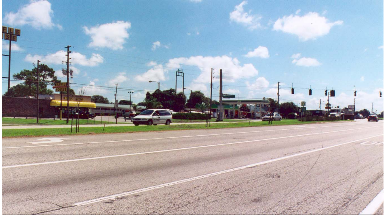
A BP retail fuel and service station east of the I-75 ROW.
