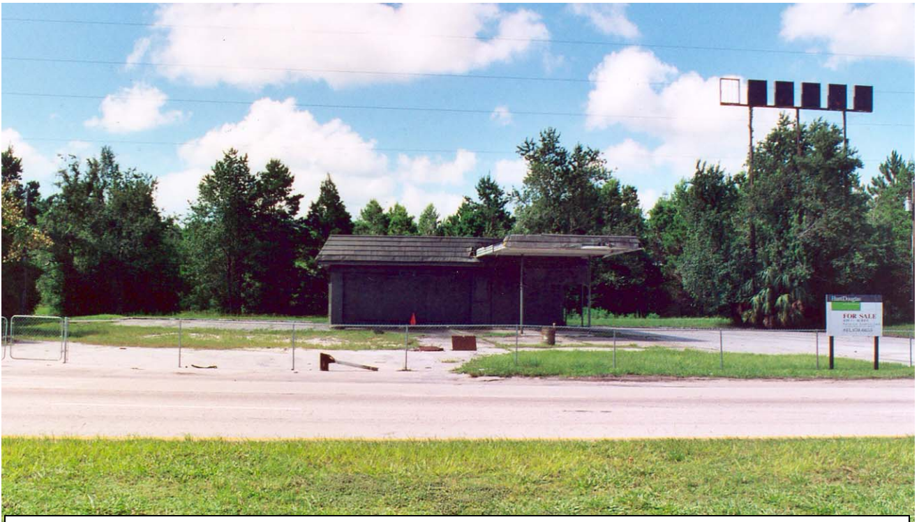
Site #3- south facing view of former Texaco #203-132 at 30436 Cortez Blvd (SR 50) east of the I-75 ROW. Rated MEDIUM
