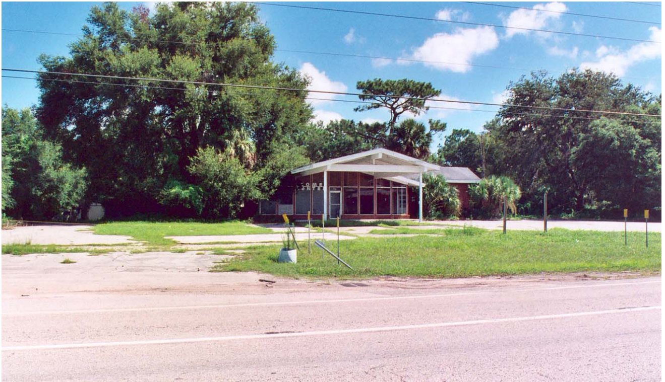
Site #2- former Exxon #5285 at 30435 Cortez Blvd (SR 50) and I-75. Air stripper located in trees to left (west) of building. Rated MEDIUM
