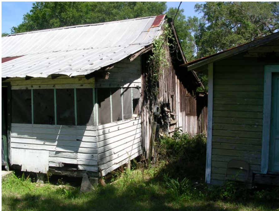
Photo 6.9. The St. Clair/O'Neal Homestead Residence (8HE554), south and east elevations.
