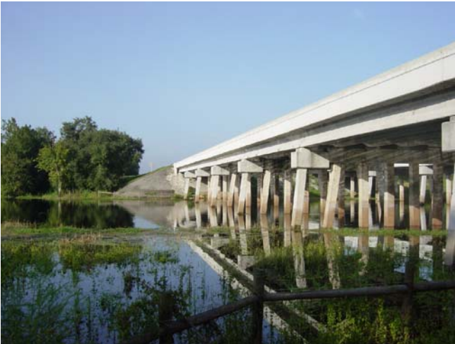
Southerly view of Withlacoochee River at the I-75 bridge crossing
