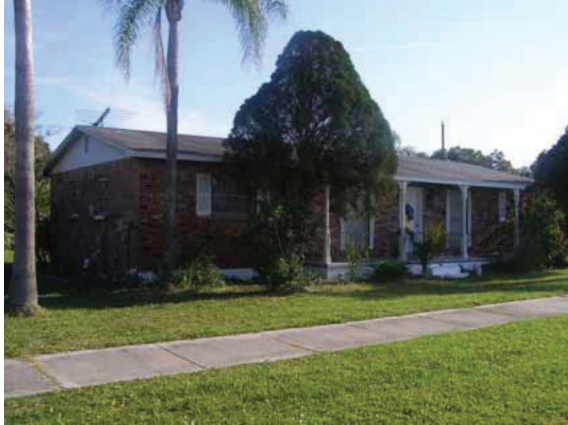
Photo 5-5: South and west elevations of 9208 Gibsonton Drive (8HI11299), looking northeast
