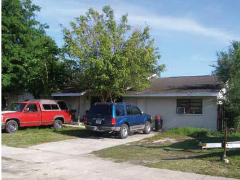
Photo 5-4: South elevation of 9002 Gibsonton Drive (8HI11298), looking northwest
