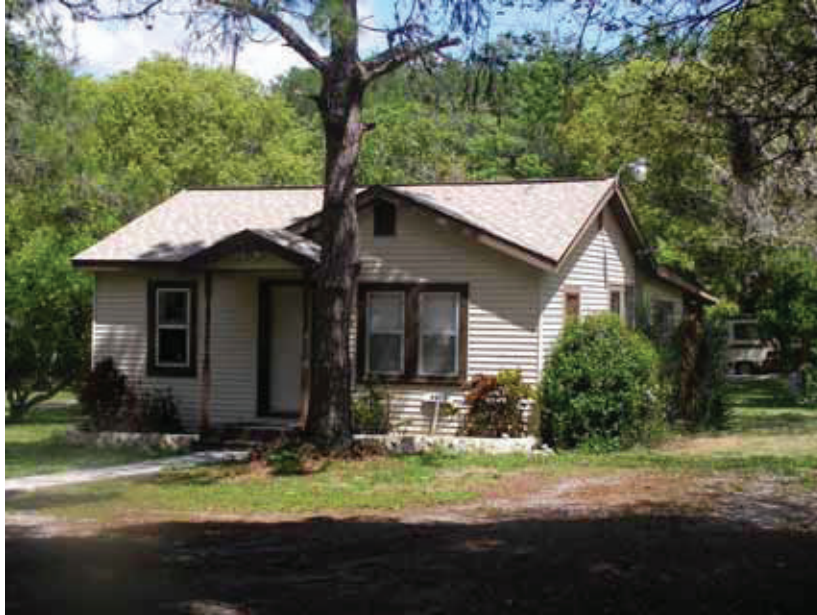
Photo 5-3: South and east elevations of 9922 Old Big Bend Road (8HI11297), looking northwest
