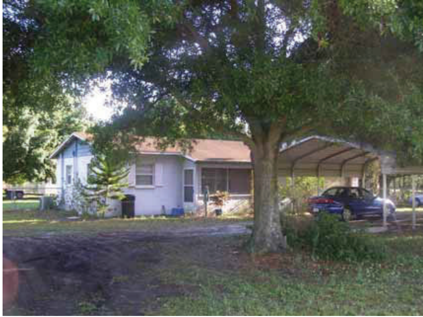
Photo 5-6: South and west elevations of 9212 Gibsonton Drive (8HI11300), looking northeast
