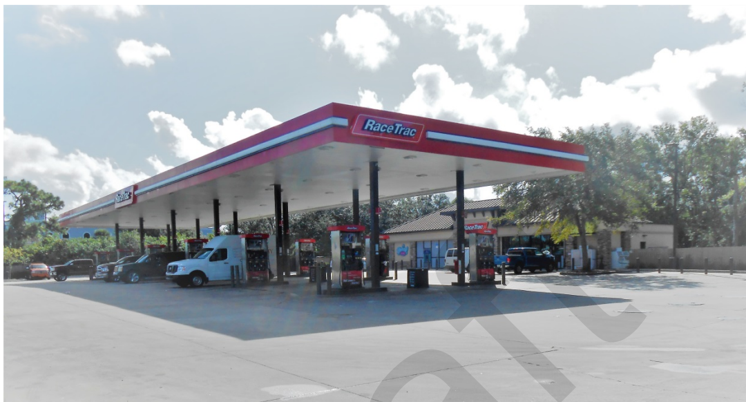
Site 8. Racetrac #631. Looking southeast. Photo taken on October 28, 2019.
