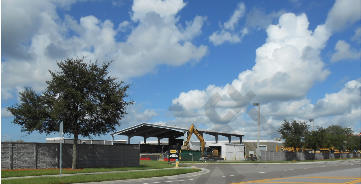
Site 20. Ring Power Corporation. Looking northwest. Photo taken October 28, 2019.
