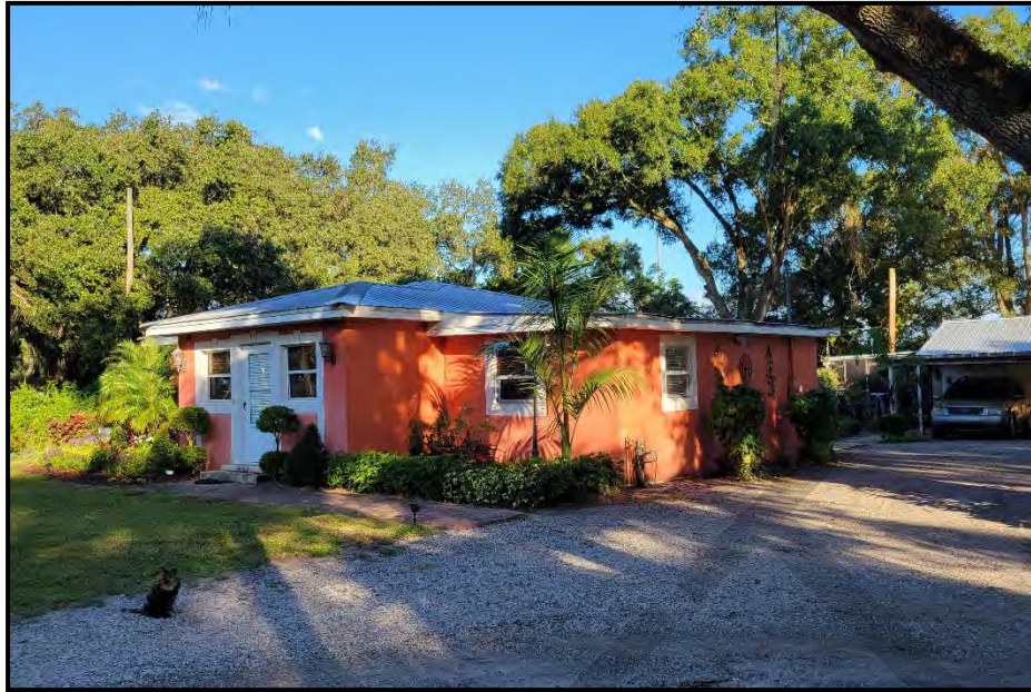
Photo 17. 10005 Hines Road (8HI15194), looking northwest.
