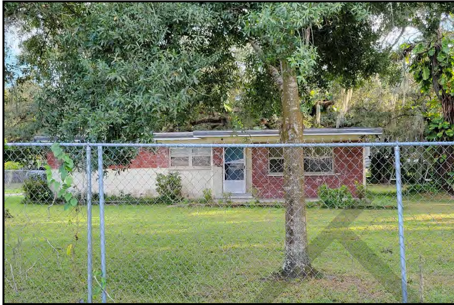
Photo 10. 5279 Eureka Springs Road (8HI15187), looking south.
