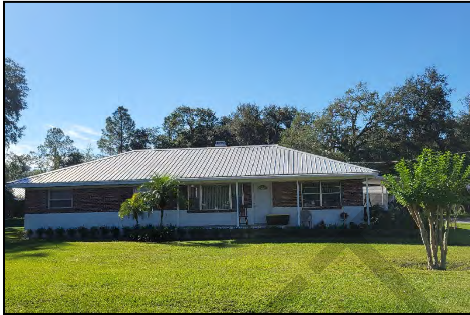
Photo 11. 5287 Eureka Springs Road (8HI15188), looking south.
