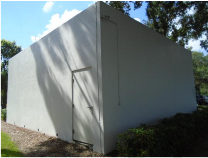
2018-08-16 Tank Containment Photo
