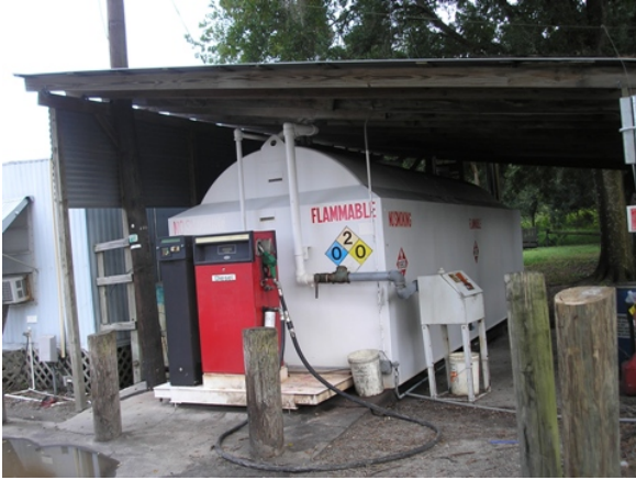
02. 2009-09-15 Facility Photo (Used Oil AST - west view)
