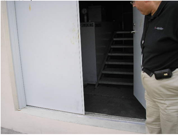
05. 2009-03-12 TCI (Spill bucket outside room)
