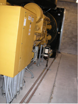
08. 2009-03-12 TCI (Piping from tank to generator room)
