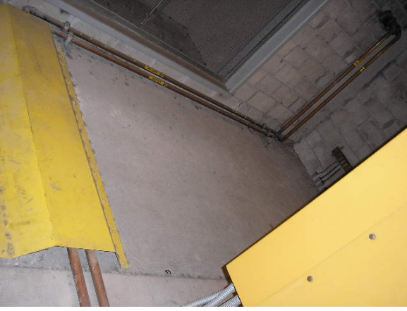
08. 2009-03-12 TCI (Piping from tank to generator room)
