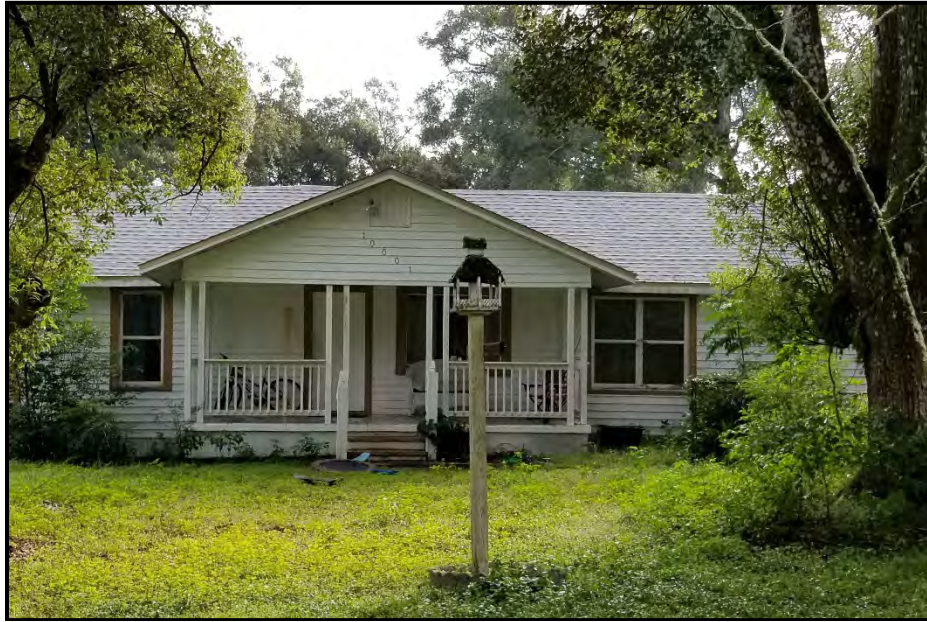
Photo 18. 10001 Morris Bridge Road (8HI14698), looking east.
