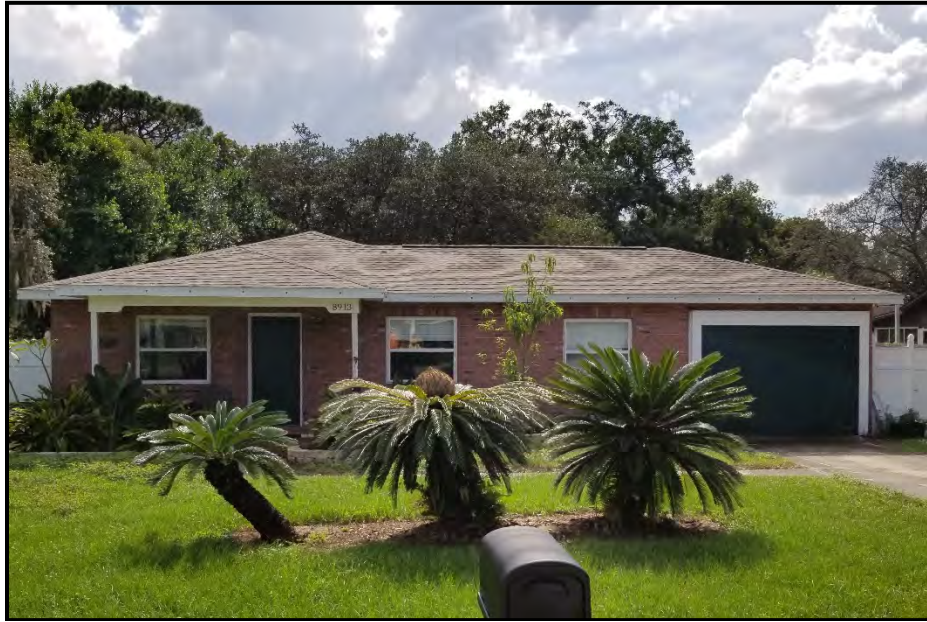
Photo 23. 8913 Navajo Avenue (8HI14703), looking south.
