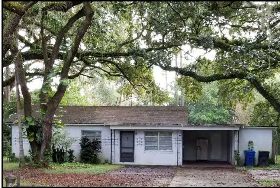
Photo 16. 9923 Morris Bridge Road (8HI14696), looking east.
