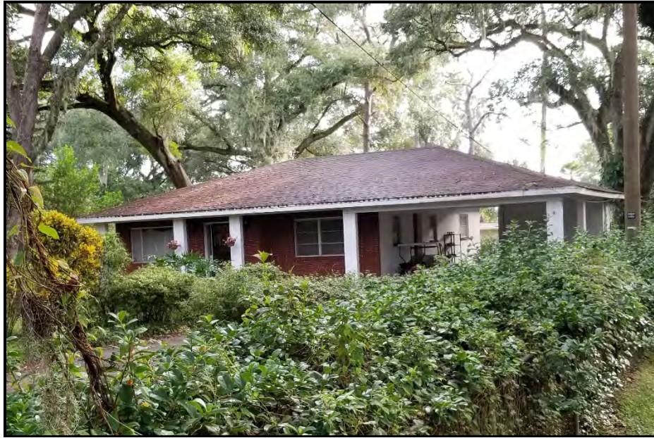
Photo 17. 9925 Morris Bridge Road (8HI14697), looking northeast.
