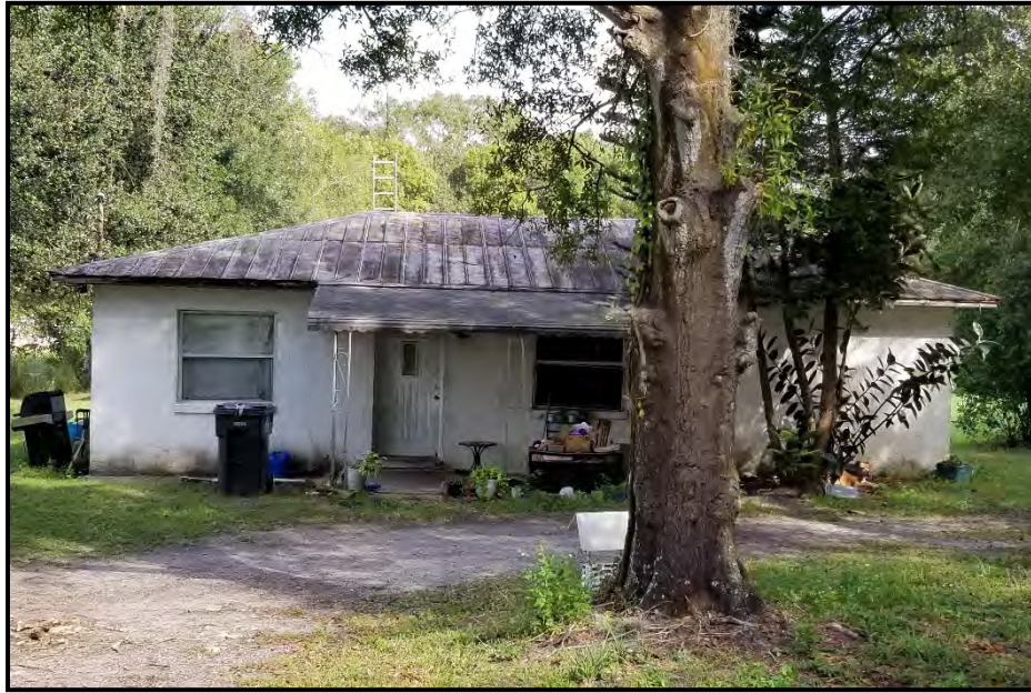
Photo 4. 2320 Fisher Avenue (8HI14686), looking north.
