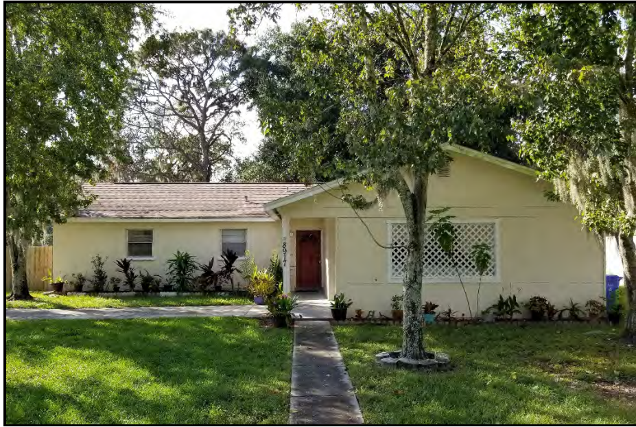
Photo 21. 8917 Navajo Avenue (8HI14701), looking south.
