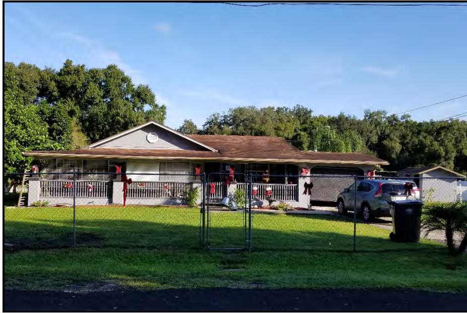
Photo 6. 2308 Fisher Avenue (8HI14688), looking north.
