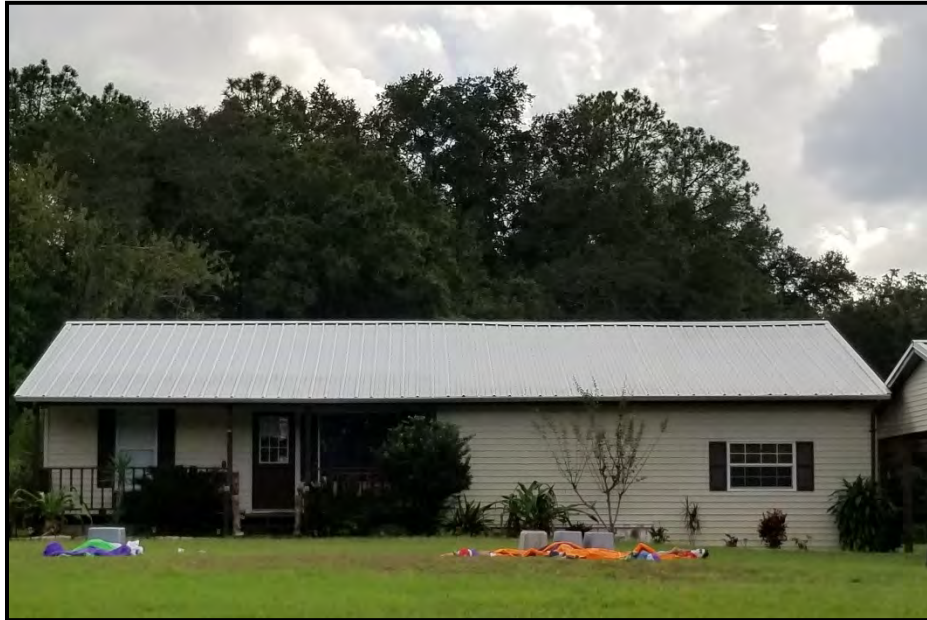
Photo 10. 9203 Harney Road (Building #1) (8HI14691), looking southeast.
