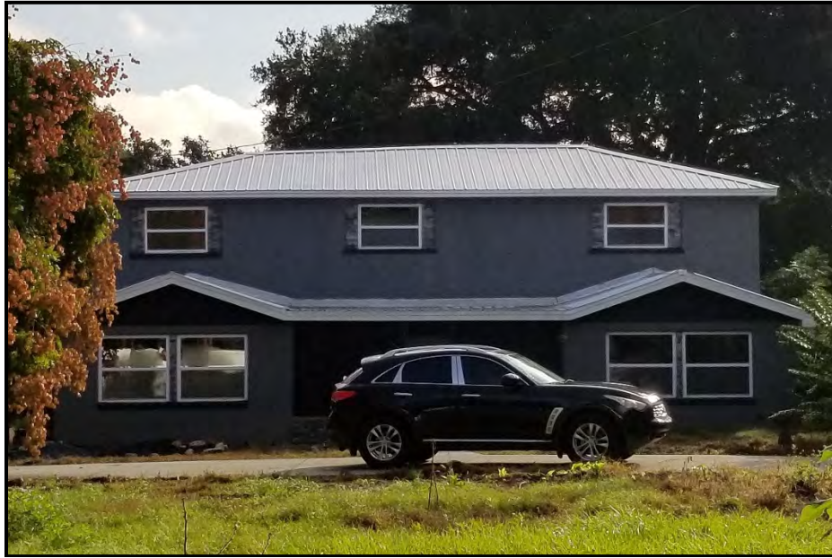
Photo 19. 10003 Morris Bridge Road (8HI14699), looking east.
