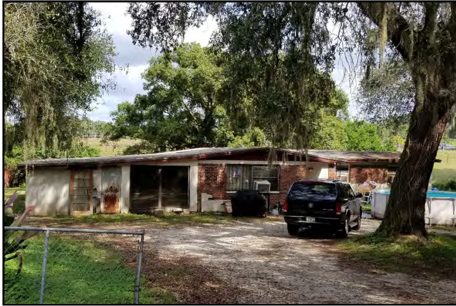
Photo 9. 9119 Bowles Road (8HI14690), looking northeast.
