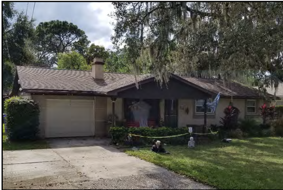
Photo 22. 8915 Navajo Avenue (8HI14702), looking southwest.
