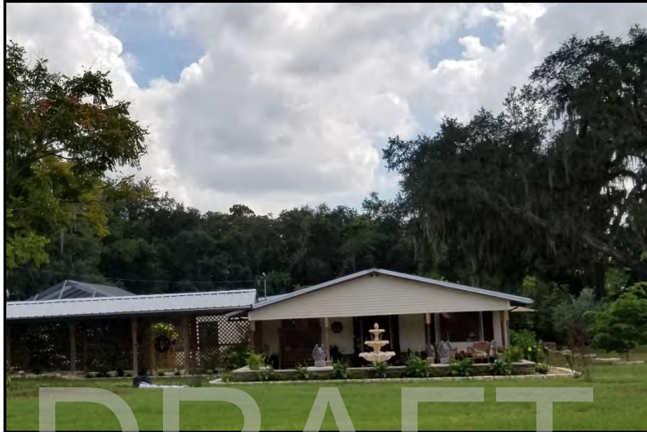
Photo 12. 9203 Harney Road (Building #2) (8HI14692), looking southeast.
