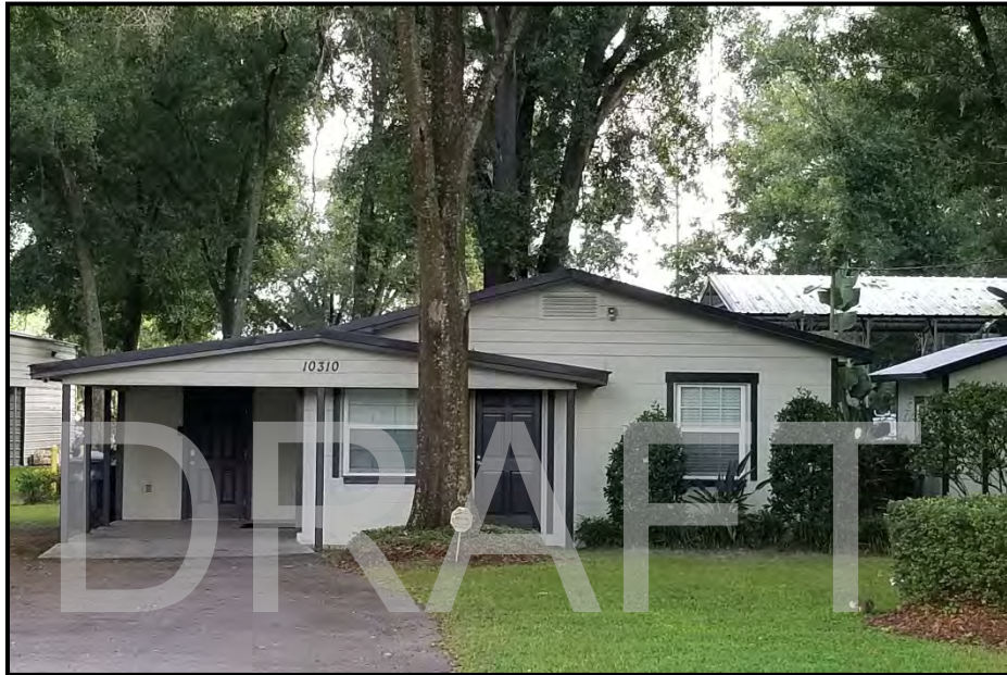
Photo 2. 10310 Woodberry Road (8HI14684), looking north.
