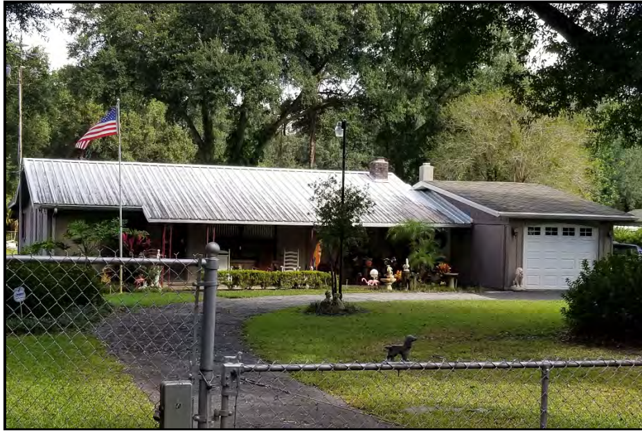
Photo 5. 2314 Fisher Avenue (8HI14687), looking north-northeast.
