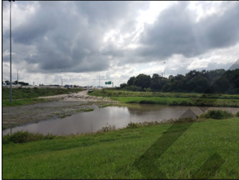
Photo 10. South view of SMF 9.
