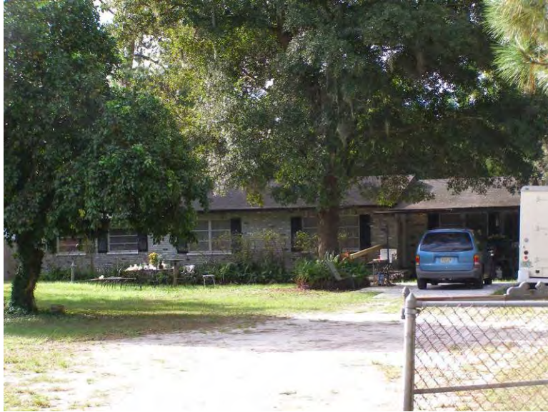
Photo 5-11 8HI11469 at 3911 McCartney Lane, looking south.
