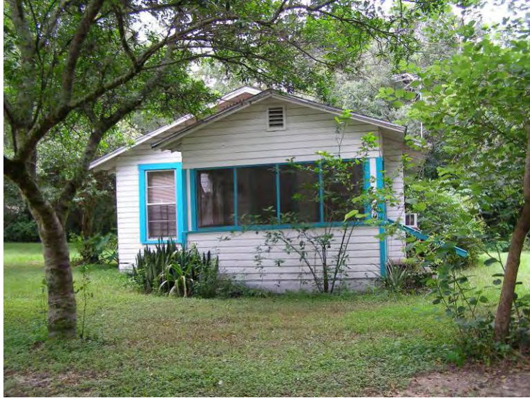
Photo 5-13 8HI7840 at 8709 Seahawk Lane, looking southwest.
