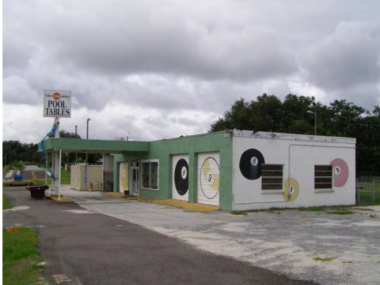
Photo 5-19 8HI11465 at 9204 U.S. Highway 301, looking south.
