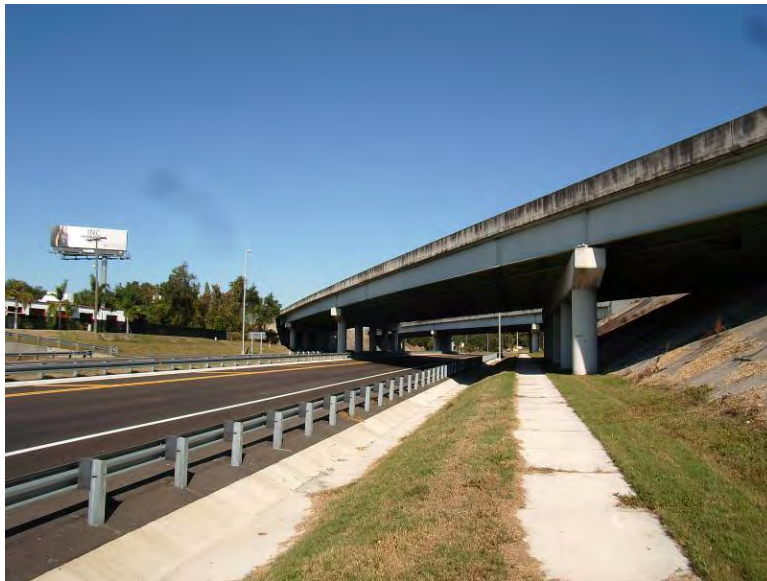
Photo 2-4 I-75 overpass at Harney Road, looking northeast.
