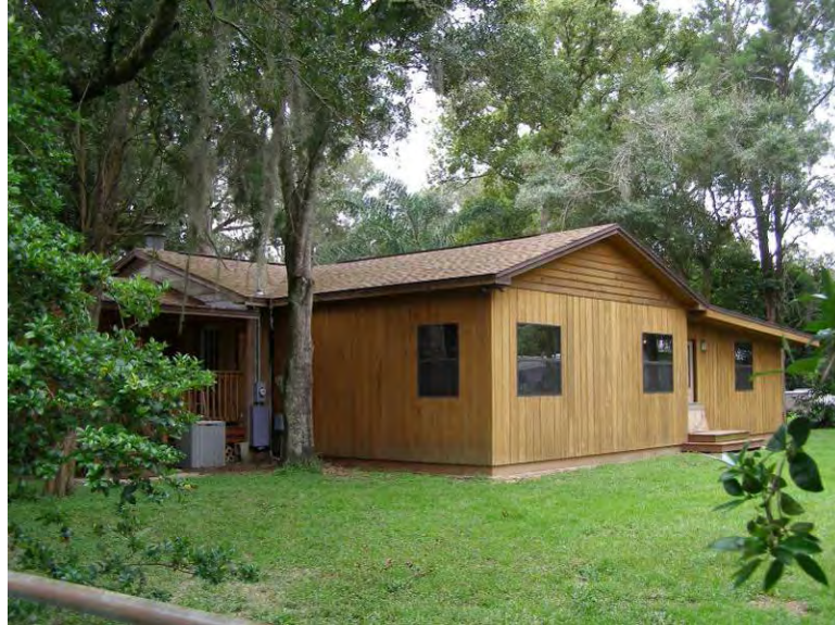
Photo 5-16 8HI11462 at 8903 McRae Road, looking southeast.
