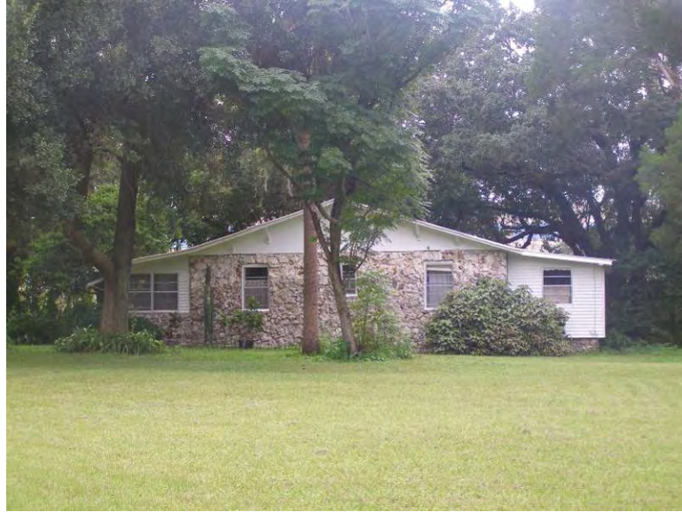
Photo 5-14 8HI11460 at 8707 127 th Avenue, looking north.
