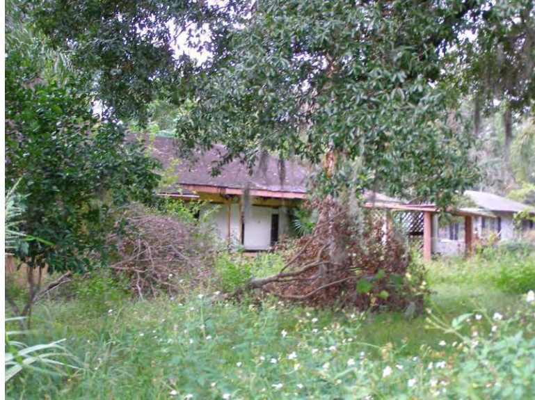
Photo 5-10 8HI11468 at 3917 McCartney Lane, looking southwest.
