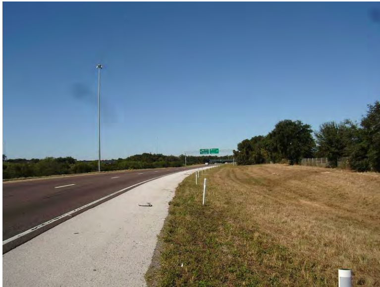
Photo 2-3 Approach to the I-4 interchange, looking northwest.
