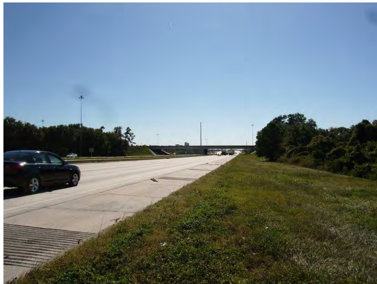
Photo 2-2 Approach to the MLK Boulevard interchange, looking south.
