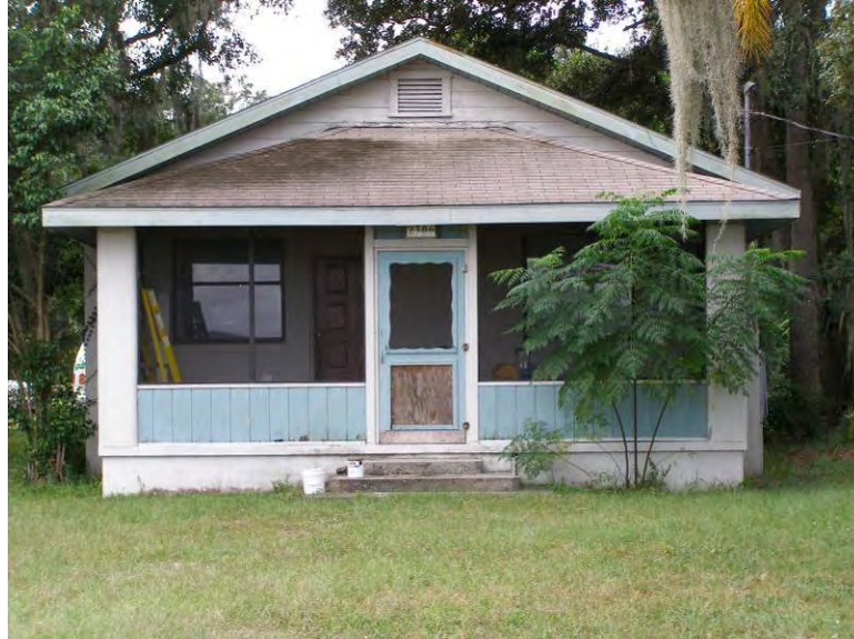
Photo 5-12 8HI11470 at 2306 Graves Road, looking south.
