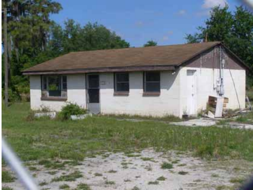
Photo 5-7: South and east elevations of 11010 Gibsonton Drive (8HI11301), looking northwest
