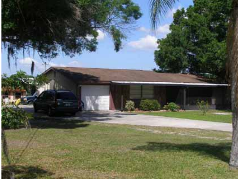
Photo 5-2: South and east elevations of 6908 Simmons Loop Road (8HI11296), looking northwest
