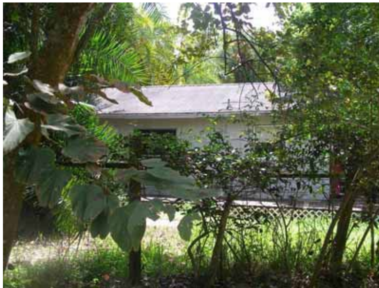
Photo 5-1: North elevation of 2201 18th Avenue SE (8HI11295), looking south
