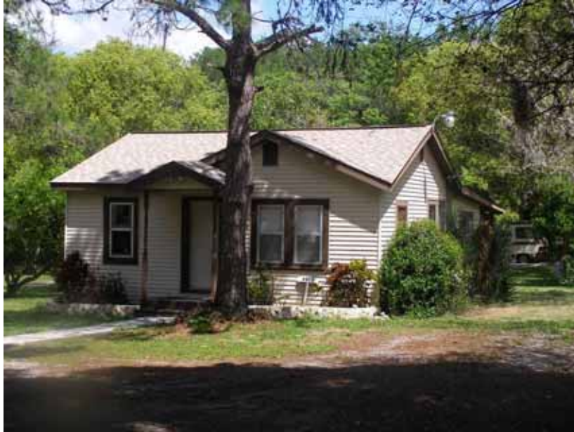
Photo 5-3: South and east elevations of 9922 Old Big Bend Road (8HI11297), looking northwest
