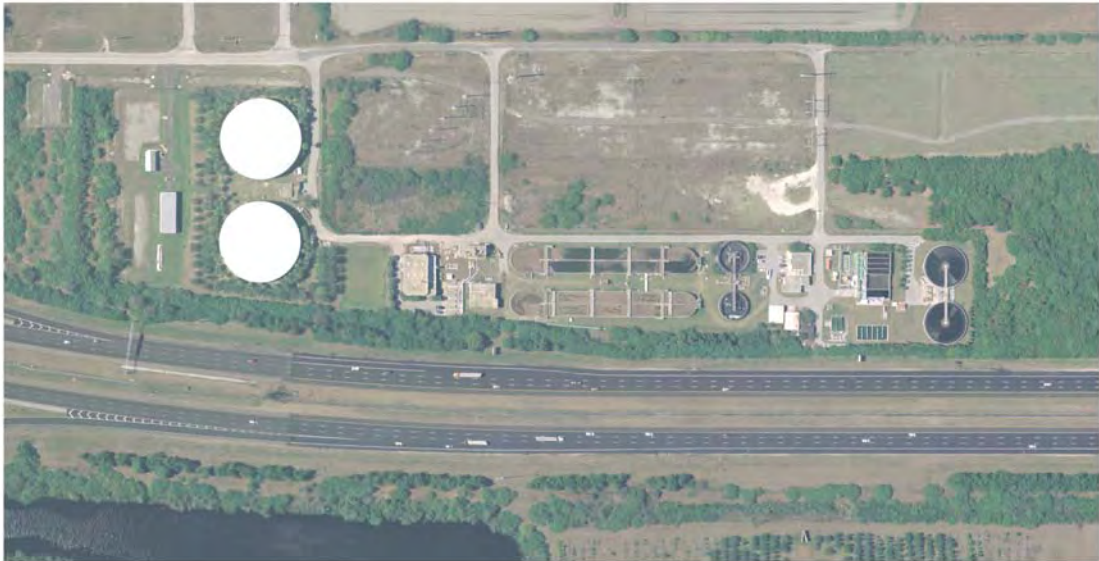
South County Regional Wastewater Treatment Plant
