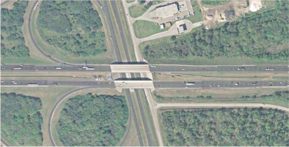
Phosphoric Acid Sludge Spill
