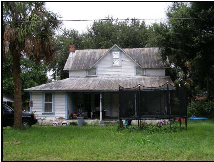
Photo 4-1. South elevation of the Tanner residence at 10426 Tanner Road, looking north.
