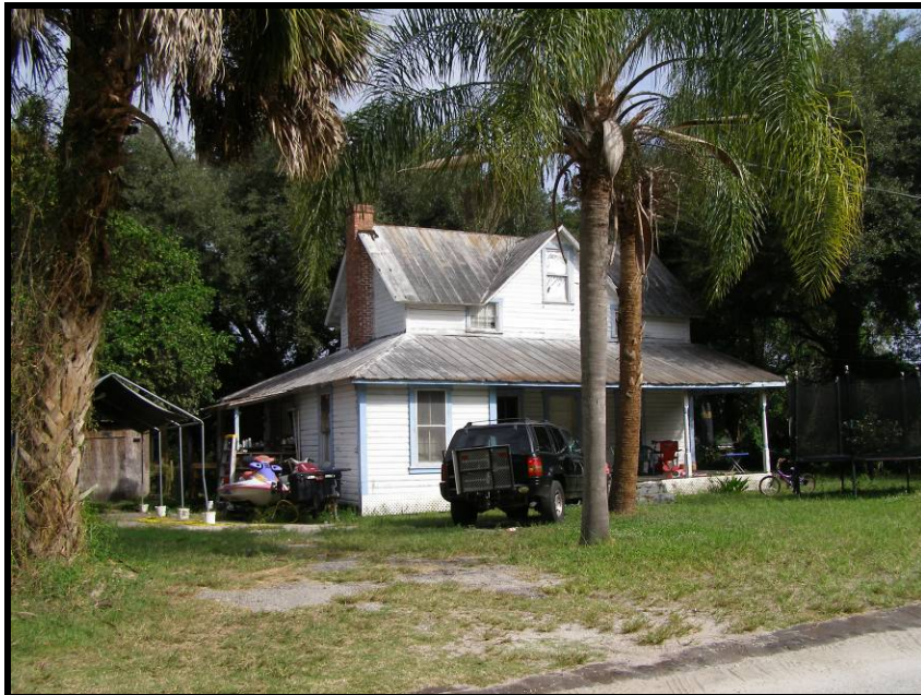
Photo 4-2. West and south elevations of the Tanner residence, looking northeast.
