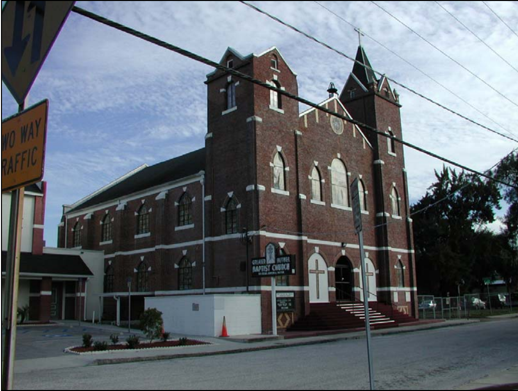
Photo 3-2 Greater Bethel Baptist Church, facing southeast
