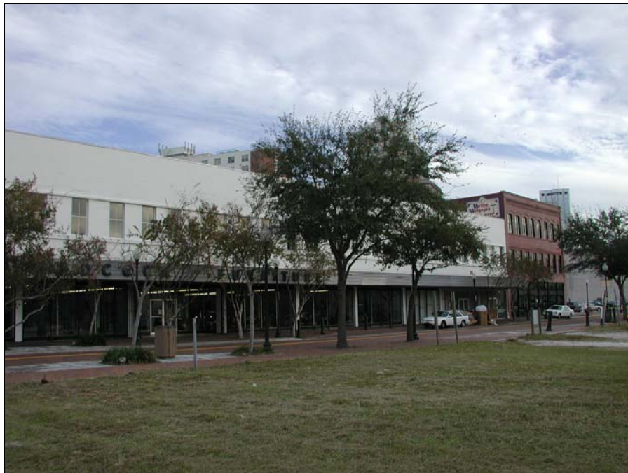
Photo 3-6 North Franklin Street Historic District, facing southeast
