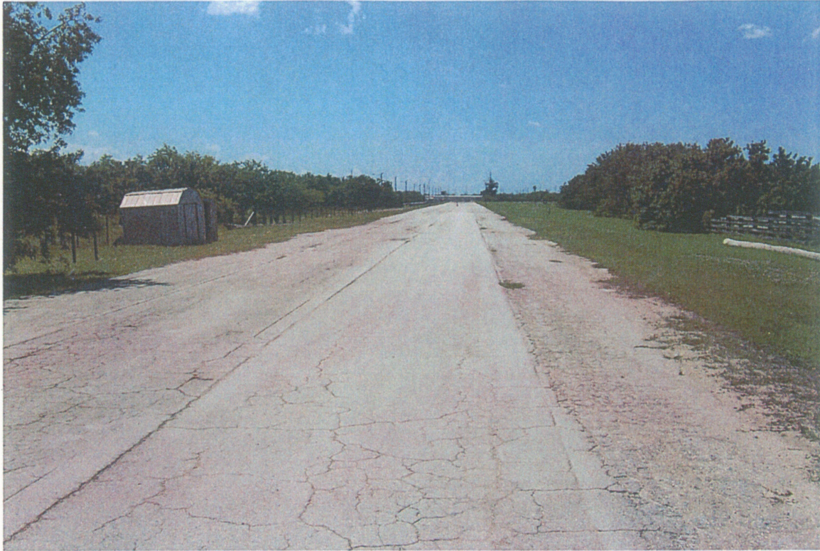
View looking south along entrance roadway to race track located on southern portion of project site.
