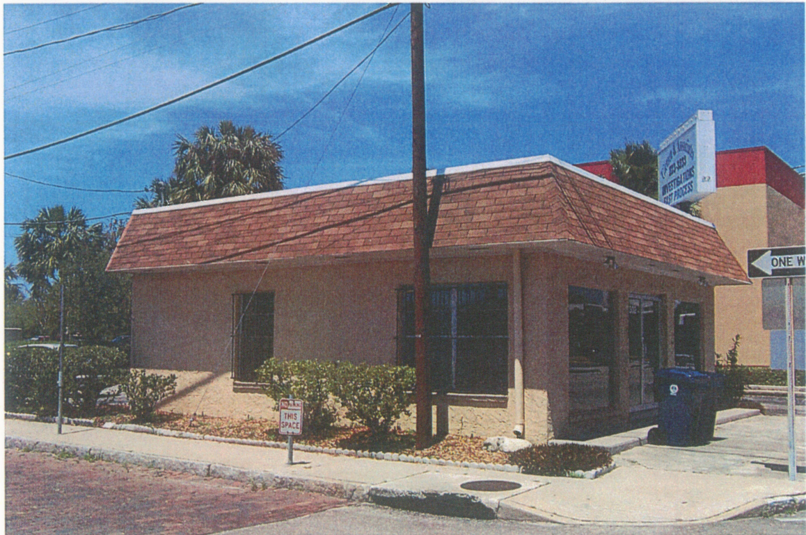
View of small office building located at 1302 N. Florida Avenue (on project site).
