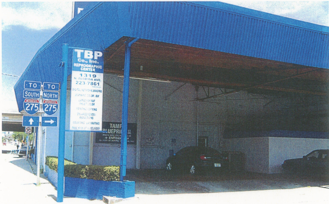
View of Tampa Blueprint facility located at 1319 N. Florida Avenue (on north central portion of project site).
