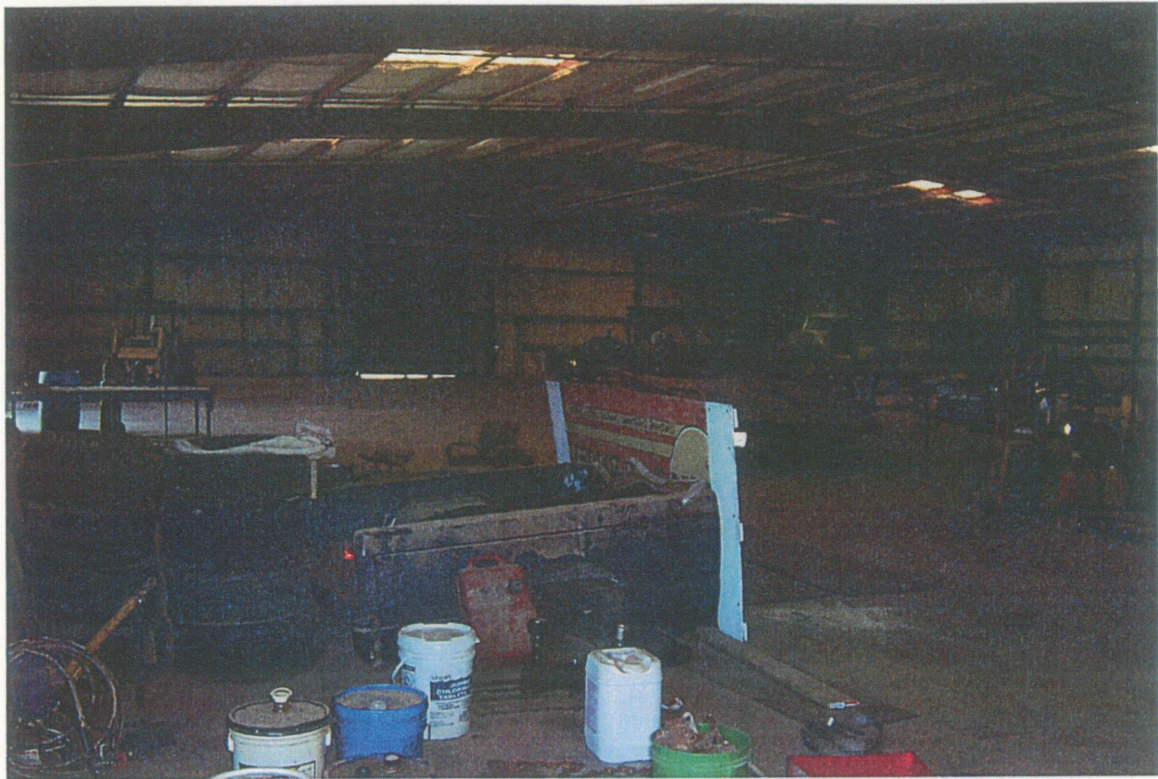
View of interior of steel storage shed located on southern portion of project site.
