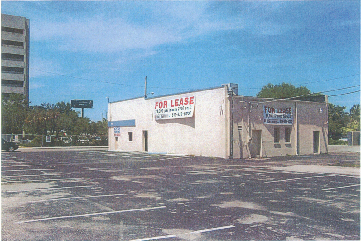
View of vacant building located at 1221 N. Florida Avenue (on central portion of project site).
