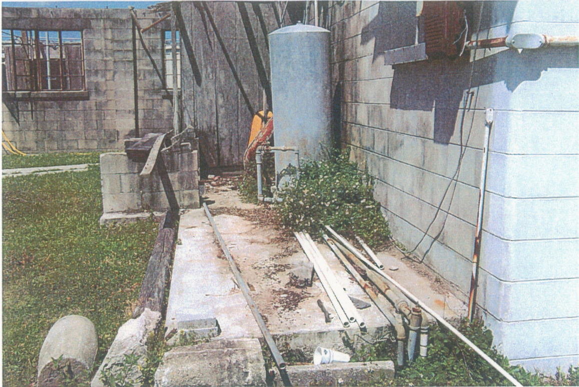
View of water well and tank located behind feed store on northern portion of project site. Concrete saddle for former water tank can be seen to the left of the onsite well.
