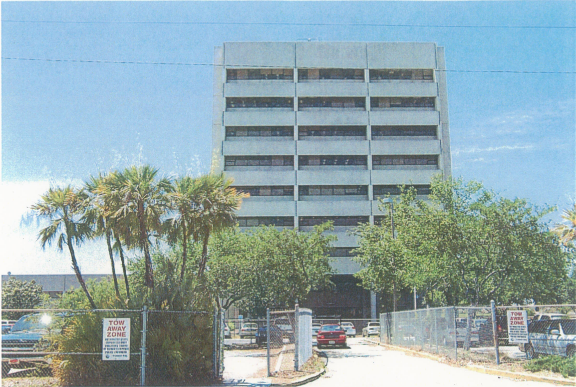
View of Park Trammell building located on western portion of project site.
