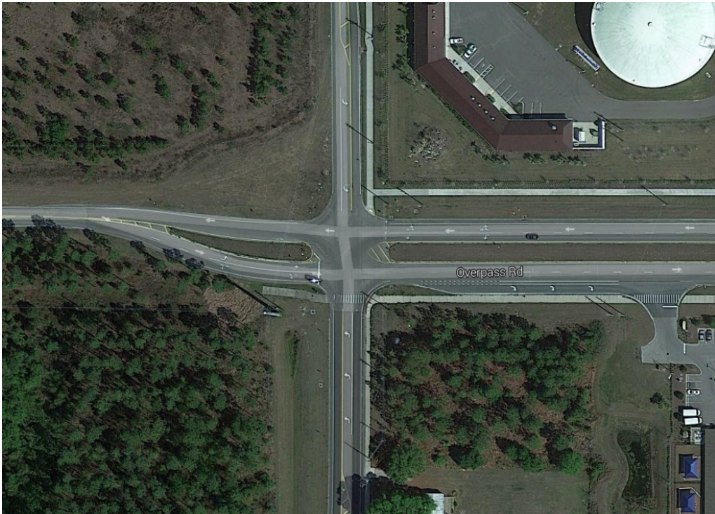
FIGURE 3-8 OVERPASS ROAD AT BOYETTE ROAD
