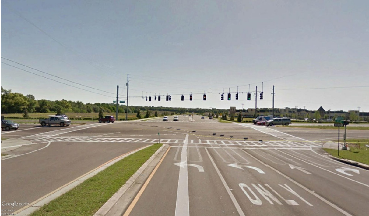
FIGURE 3-5 EXISTING TYPICAL SECTION KOSSIK ROAD JUST WEST OF US 301 (LOOKING EAST)
