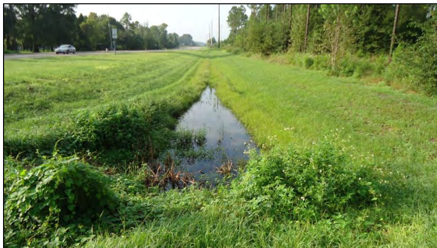
Ditch 3 facing south from Overpass Road FLUCFCS: 510 – Streams and Waterways
