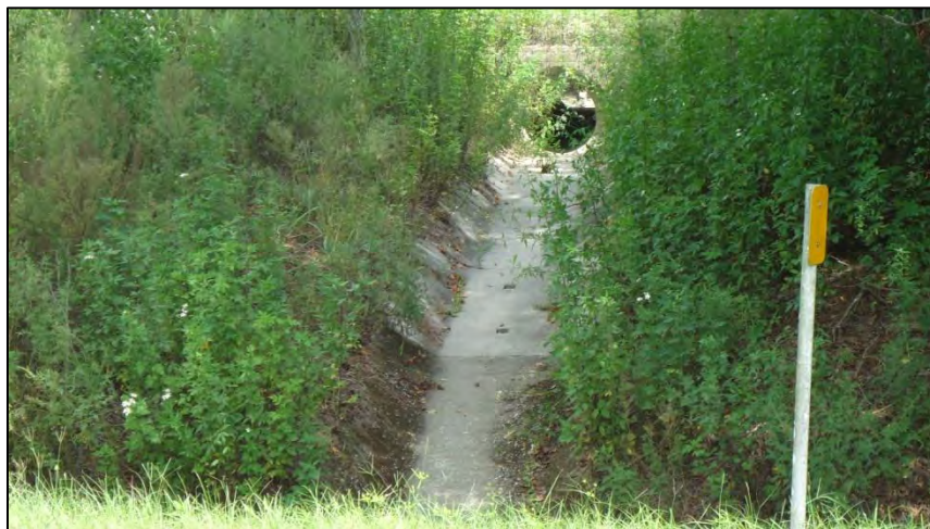
Ditch 22 facing east from I-75 FLUCFCS: 510 – Streams and Waterways
