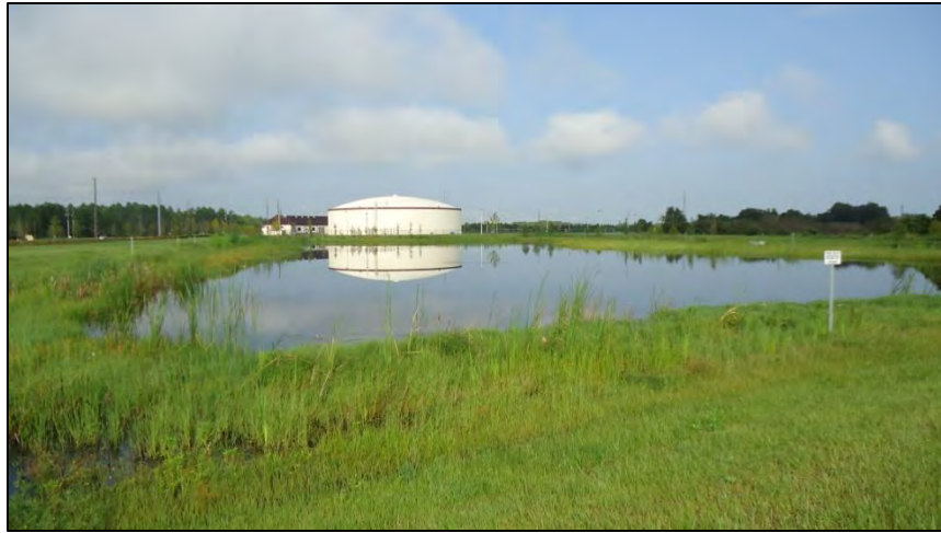
Surface Water 2 facing west FLUCFCS: 534 – Reservoirs less than 10 acres
