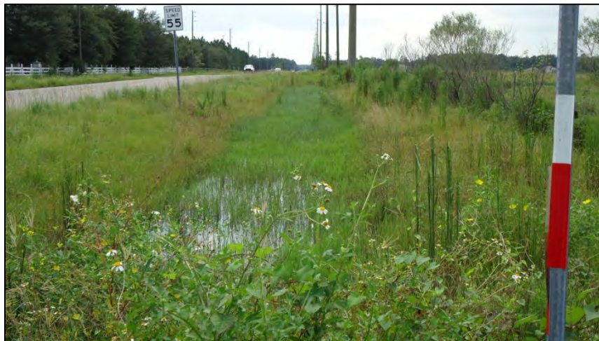
Ditch 9 facing north from Handcart Road FLUCFCS: 510 – Streams and Waterways
