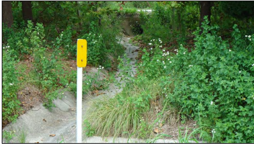
Ditch 23 facing east from I-75 FLUCFCS: 510 – Streams and Waterways
