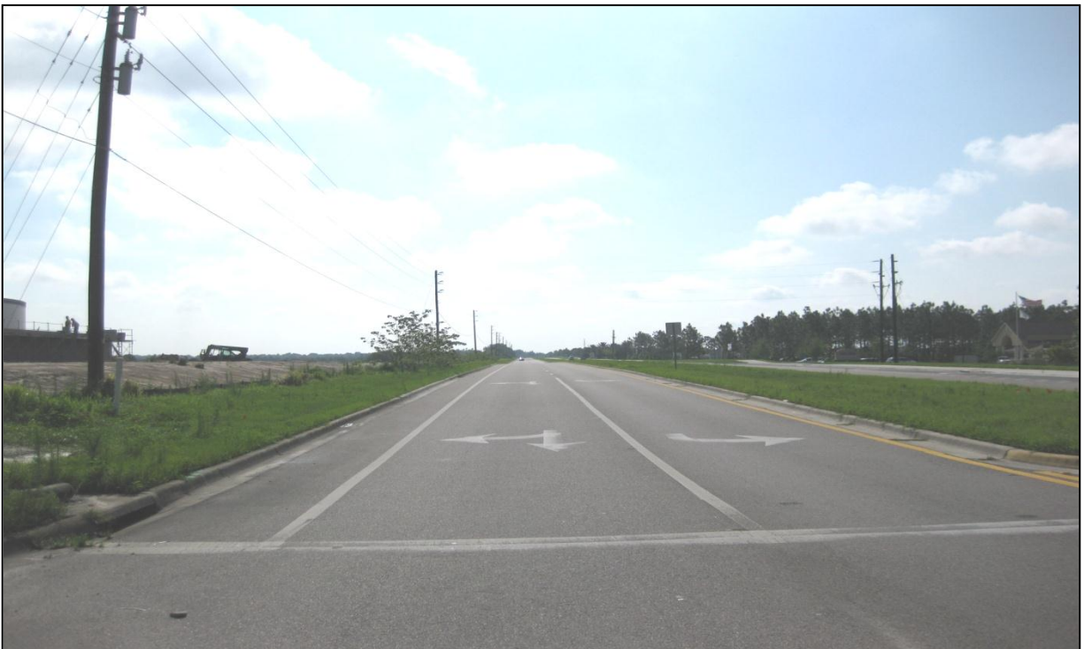
FIGURE 2-3 OVERPASS ROAD EXISTING TYPICAL SECTION EAST OF BOYETTE ROAD (LOOKING EAST)
