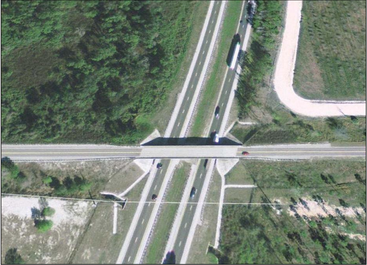
FIGURE 2-9 AERIAL VIEW OF OVERPASS ROAD BRIDGE OVER I-75
