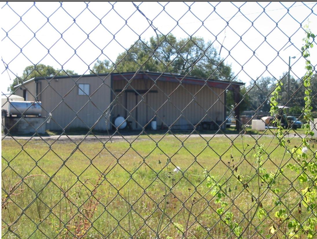
Site 5: Hemphill Groves
